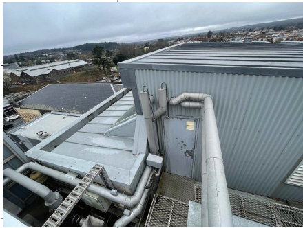
FIGURE 2 - EXISTING HHW / CHW FLOW AND RETURN PIPEWORK PENETRATING PLANT ROOM.
