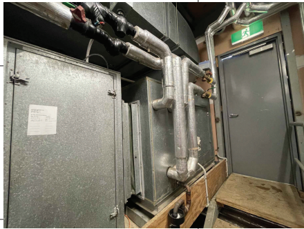
FIGURE 3 - EXISTING FAN COIL UNIT (TYPICAL FOR FCU 2.1, 2.2 AND 2.3).
