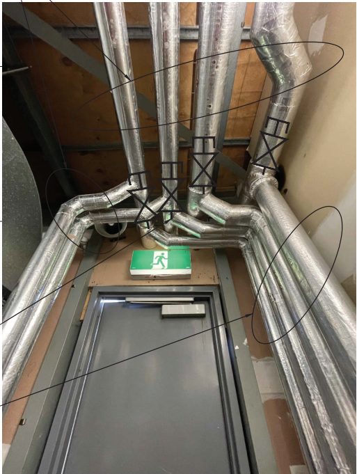
FIGURE 1 - HHW / CHW FLOW AND RETURN PENETRATING PLANT ROOM.
