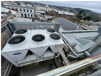
FIGURE 4 - EXISTING CHILLER AND ASSOCIATED EQUIPMENT.
