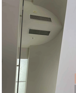
FIGURE 5 - EXISTING SUPPLY AIR PLENUM.
