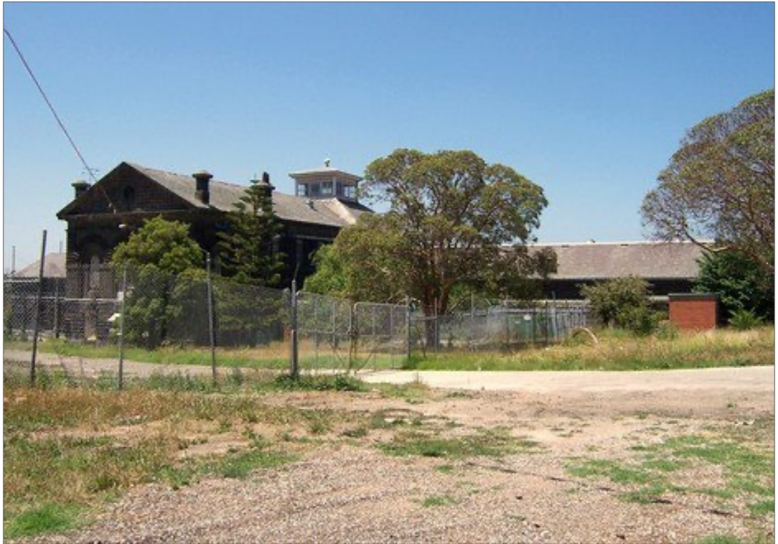
Figure 7 A Division viewed from the west, c2000. Note that the façade is partially obscured by mature trees. Source: H M Pentridge Prison Facebook page.
