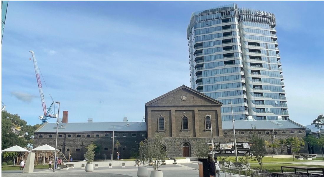
Figure 21 Adina Hotel/Apartment tower behind historic B Division.
