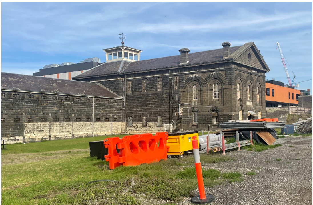
Figure 12 A Division viewed from the north-west.
