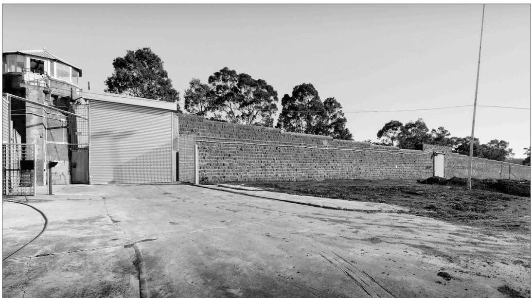
Figure 8 View from the south-west of A Division showing the Champ Street prison wall. Source: Hin Lim Photography
