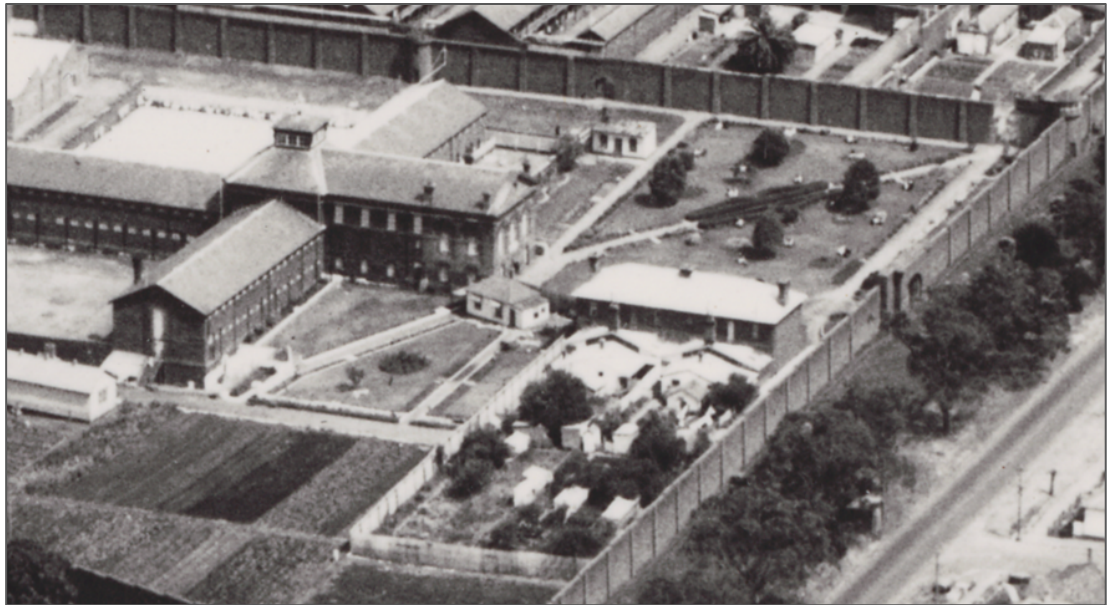
Figure 3 Part of a c1935-40 aerial photograph of Coburg showing the area to the west of A Division. Photographer Charles Daniel Pratt. Source: State Library of Victoria.
