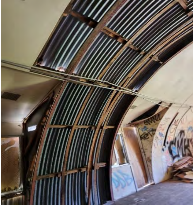
Figure 2 Interior of Structural Arch
