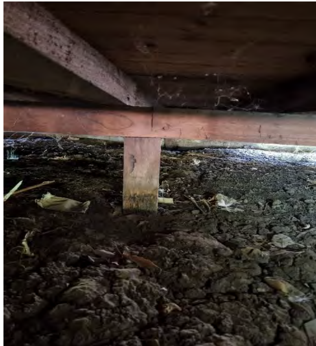
Figure 5 Floor Support Structure
