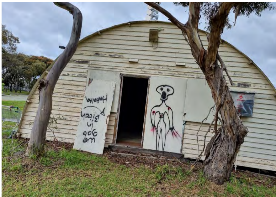
Figure 1 Nissen Hut Exterior - Front
