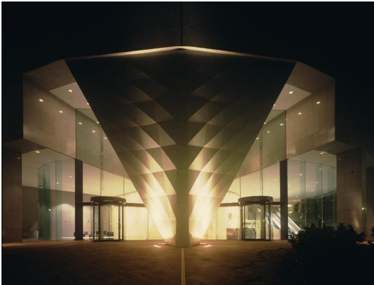
Figure 17 Photograph (c. 1989) showing the inverted triangular transfer column at the Spring Street entrance, which gathers three external tower columns onto a single footing Source: courtesy Harry Seidler & Associates
