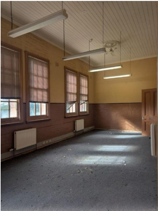
Figure 27 View of one of the dormitory on the first floor with the timber lined ceilings
