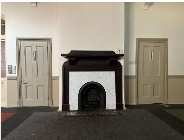
Figure 17 One of the fireplaces with the timber mantelpiece in the former Day Room
