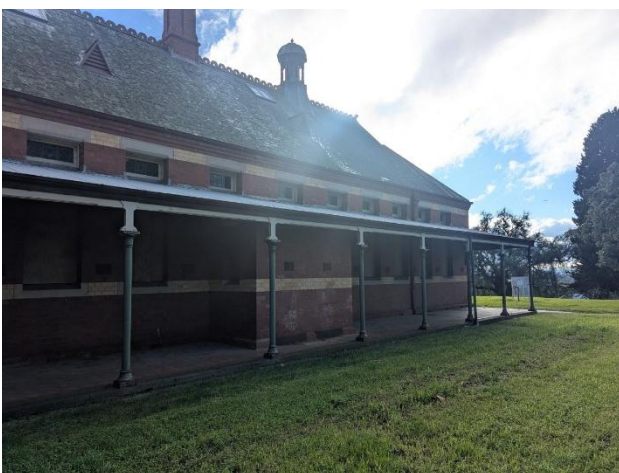
Figure 13 East elevation of B26 showing the lean-to verandah with the metal columns and timber detailing
