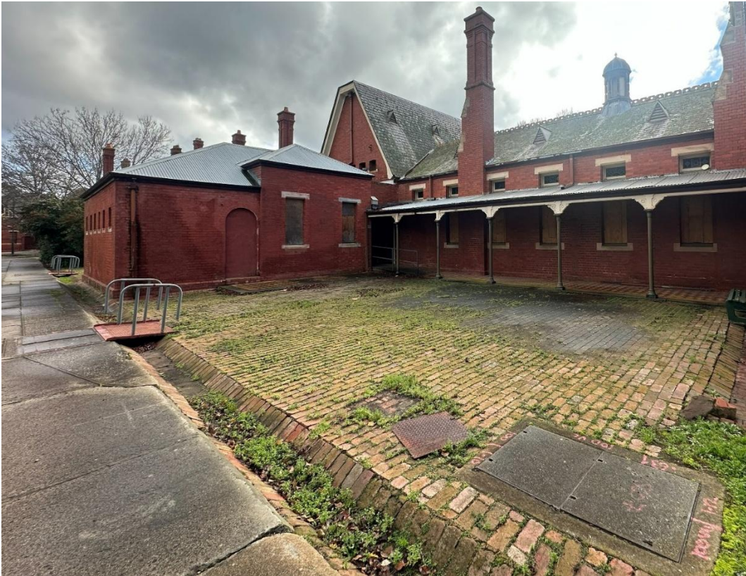
Figure 7 Brick paving and brick-lined drain to the rear (south) of B28: the alignment of Tram Road, visible at left, is finished in concrete
