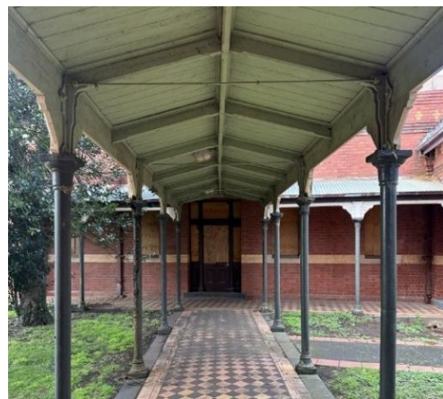
Figure 32 Verandah connecting from the Admin Building to B28
