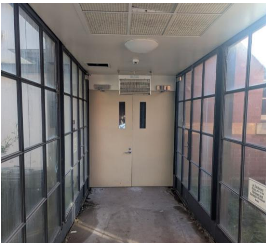
Figure 19 Modern glazed walkway at south of B26
