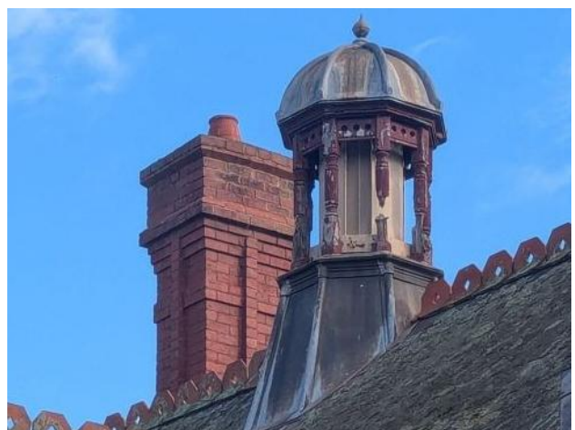
Figure 14 Detail of one of the timber cupolas and the corbelled brick chimney of B26
