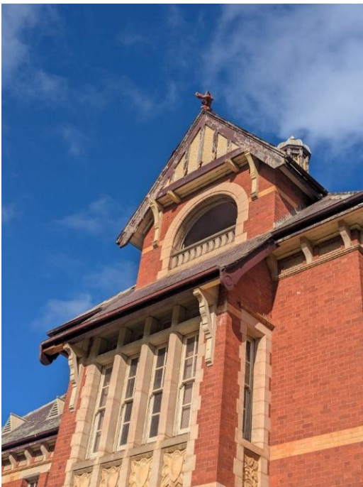
Figure 23 Detailed view of the balcony on the second floor set within the roof. Note the half timber detailing to the gable end
