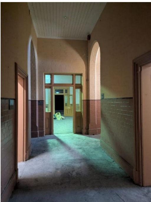
Figure 25 View of the central corridor on the ground floor with the flagstone flooring
