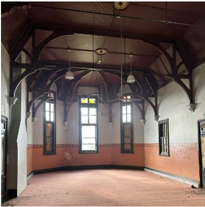
Figure 34 Central day room with the timber trusses and timber lined ceiling, facing north
