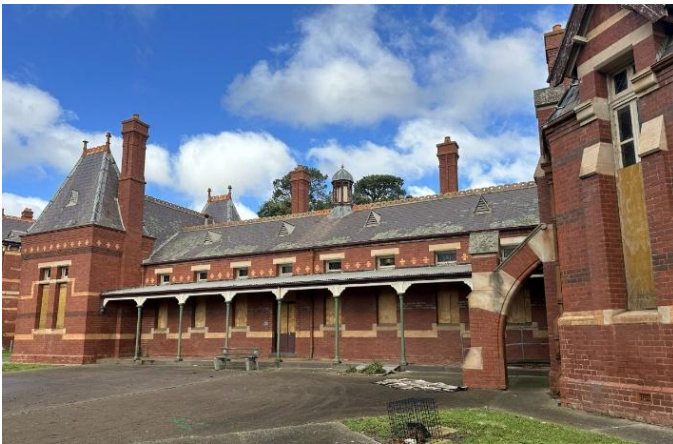
Figure 29 North elevation of B28. Note sloping roof with slate tiles above the east wing
