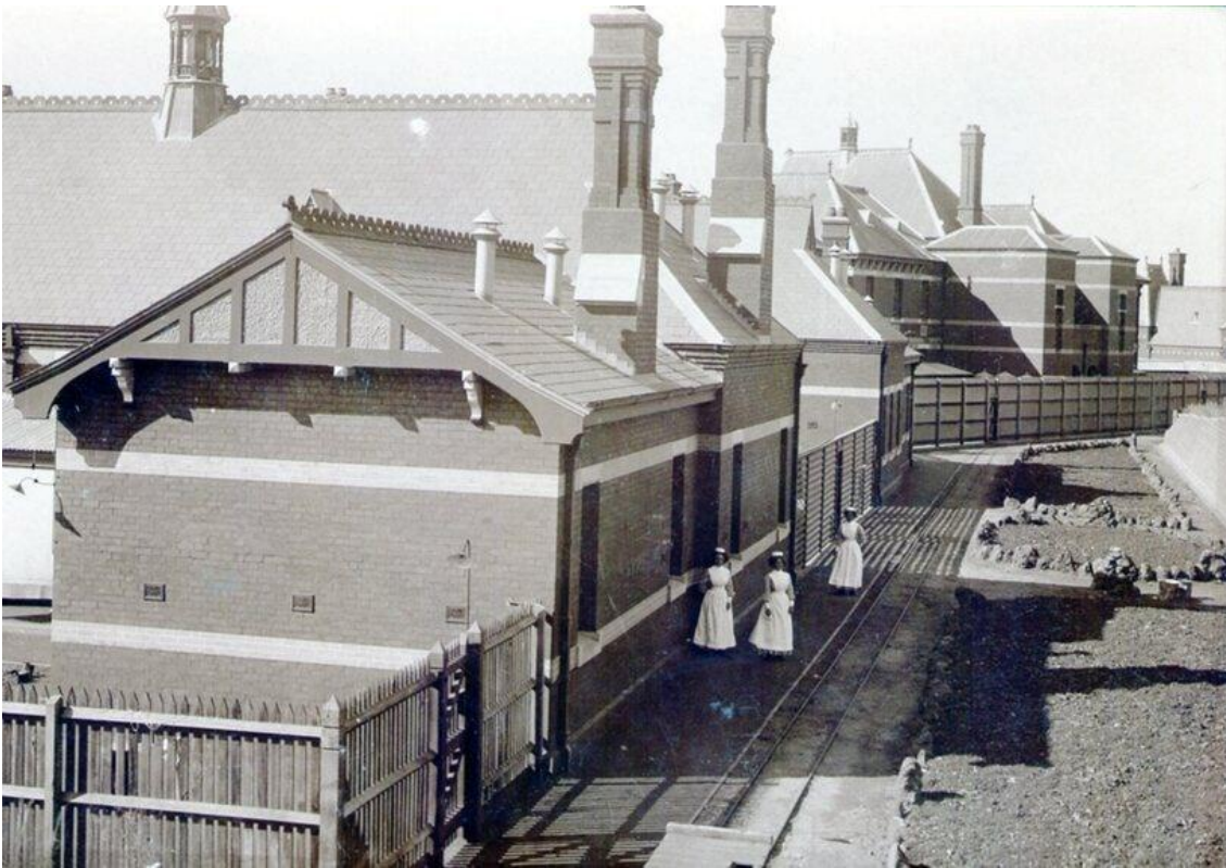
Figure 5 Photograph c.1920s of the rear of the Male Infirmary Ward (B32) showing the timber picket fence and the tramway, now the alignment of Tram Road Source: Victorian Collections, Sunbury Family and Heritage Society, Identifier: P0861
