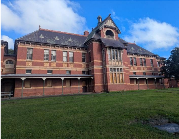
Figure 21 North elevation of B27 showing the central bay and the two-storey building on either side
