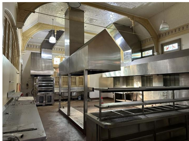
Figure 18 View of the former Infirmary Ward showing the modern kitchen fitouts
