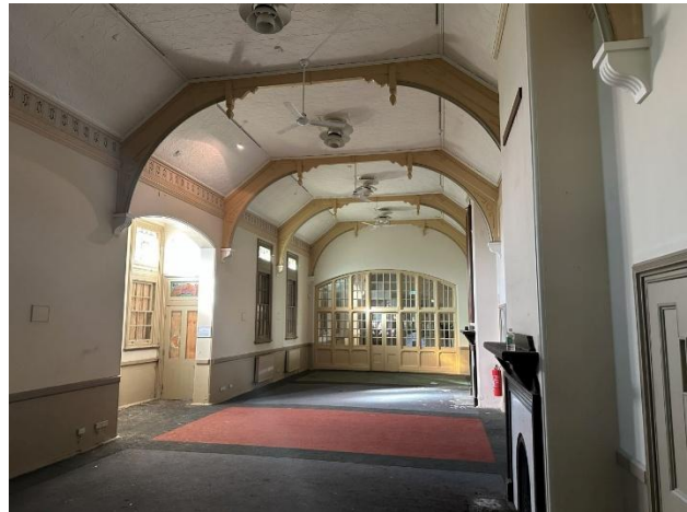
Figure 16 Day Room: note trusses, decorative cornices and pressed metal ceiling
