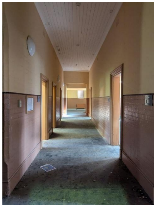
Figure 26 View of the central corridor on the first floor with the flagstone flooring
