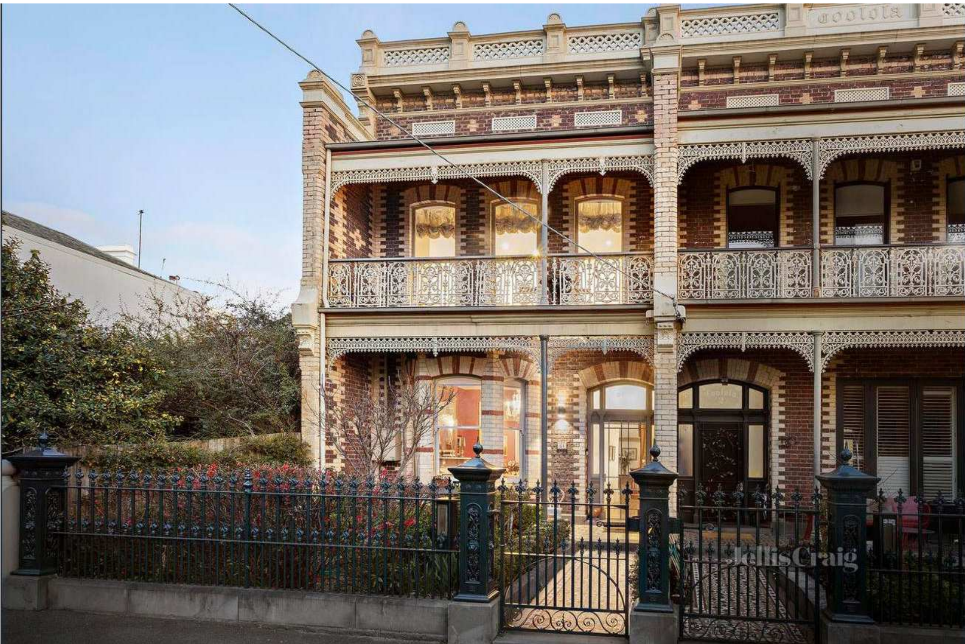
SUBJECT SITE - 61 ST VINCENT PLACE SOUTH. NO PROPOSED CHANGES TO FRONT FACADE OR FENCE
