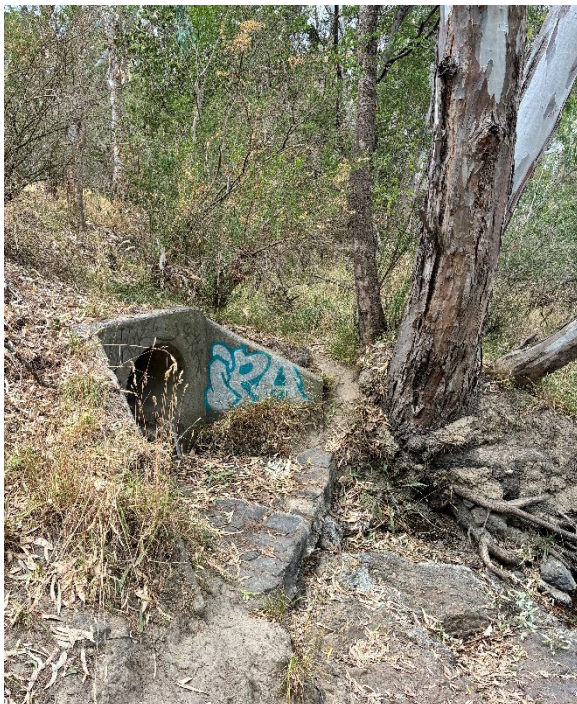
Figure 92: Concrete stormwater drain outlet on a bluestone platform adjacent the Yarra River, facing southeast (image: A. Dube 04/02/2026)
