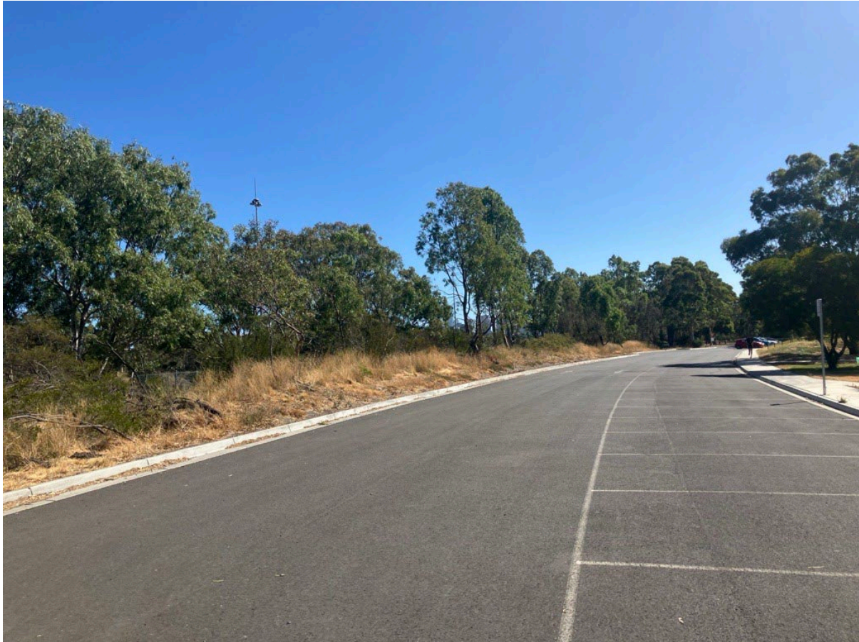
Figure 104: Fairlea Reserve Netball Courts carpark, with the earth mound on the left (image: A. Lagat 16/07/2026)
