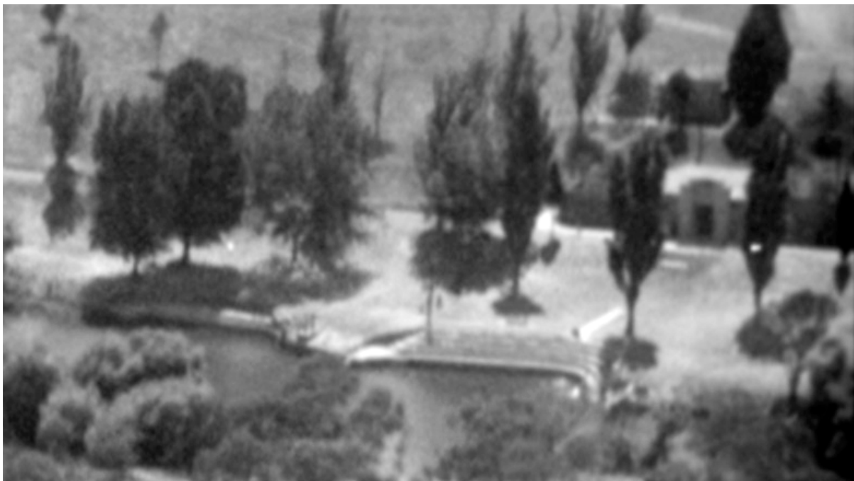
Figure 11: Close-up aerial of two concreted terraces, with the clubhouse and a building to the rear (Pratt 1958)
