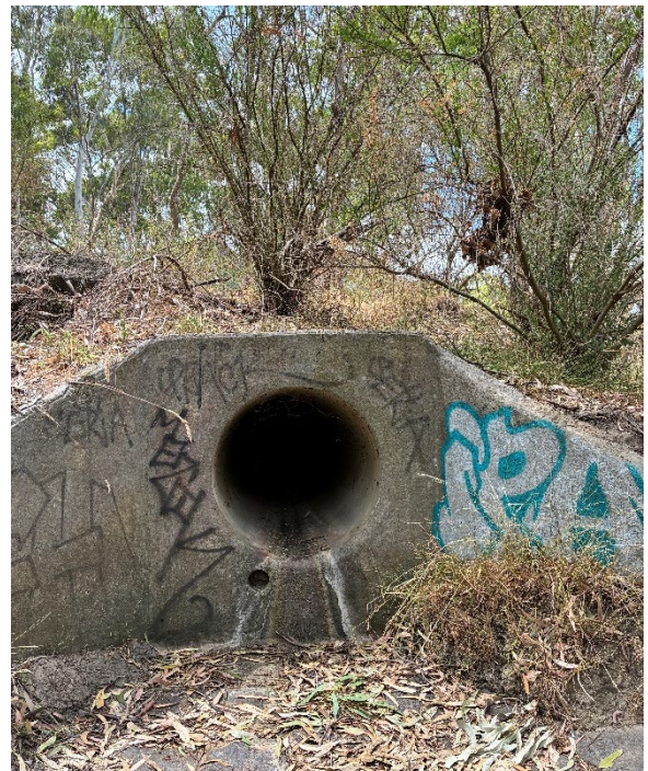
Figure 93: Concrete stormwater drain outlet on a bluestone platform adjacent the Yarra River, facing northeast (image: A. Dube 04/02/2026)
