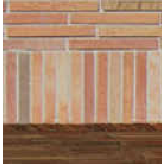
FC.03 - FACE BRICKWORK SOLDIER COURSE - BROWN CLAY FINISH
