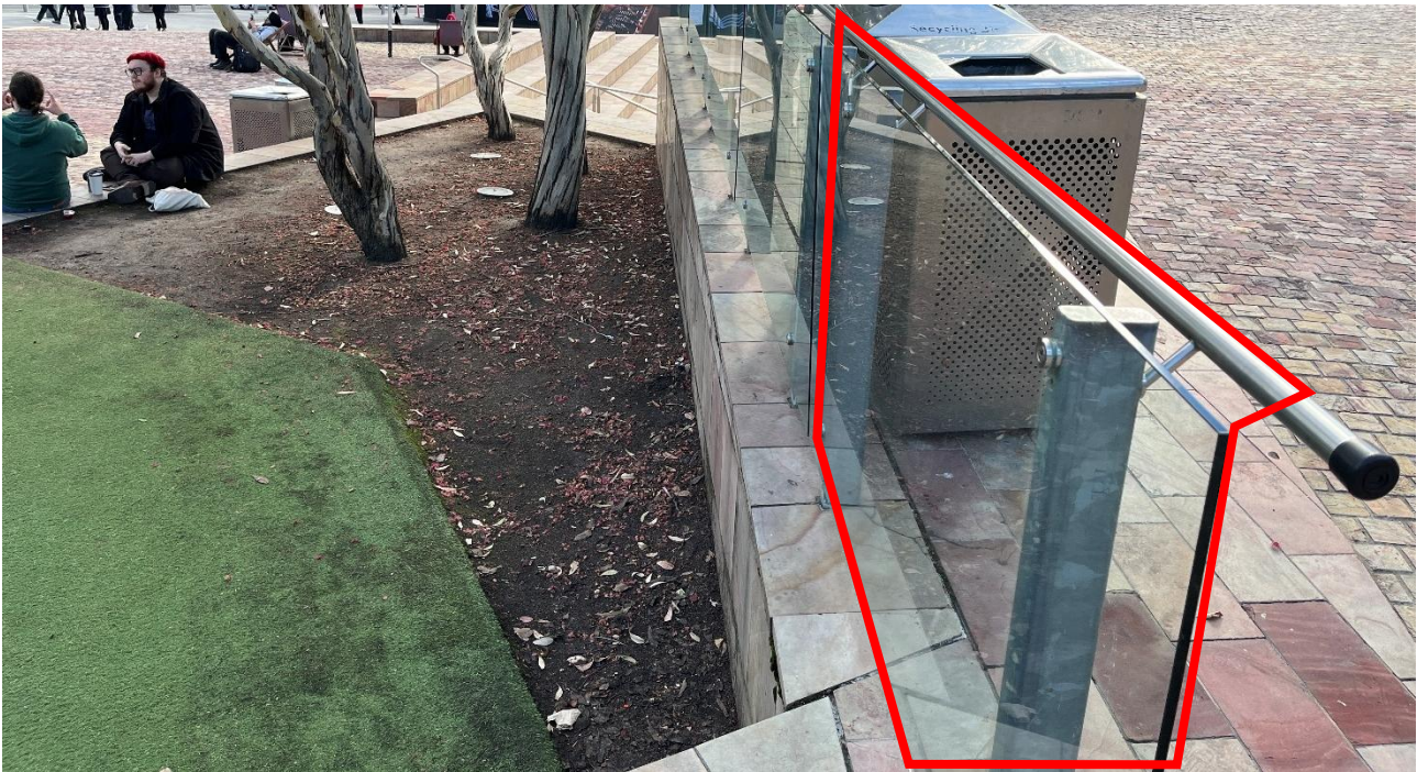
Figure 3 Section of balustrade and handrail to be temporarily dismantled, indicated in red
