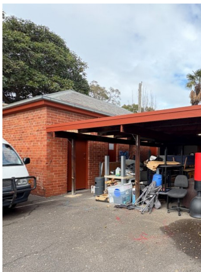
BRICK OUTER BUILDING AND CARPORT
