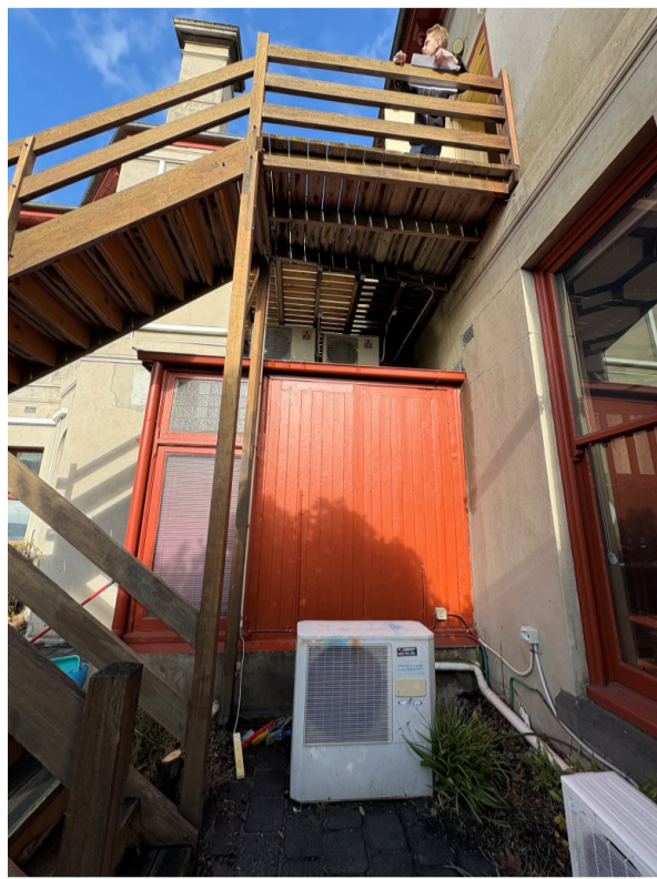
3. EXISTING AIR-LOCK (EXTERIOR)
