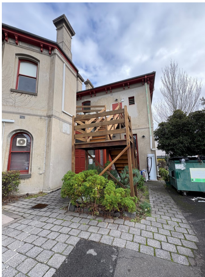
CARPARK-FACING FACADE (EAST)
