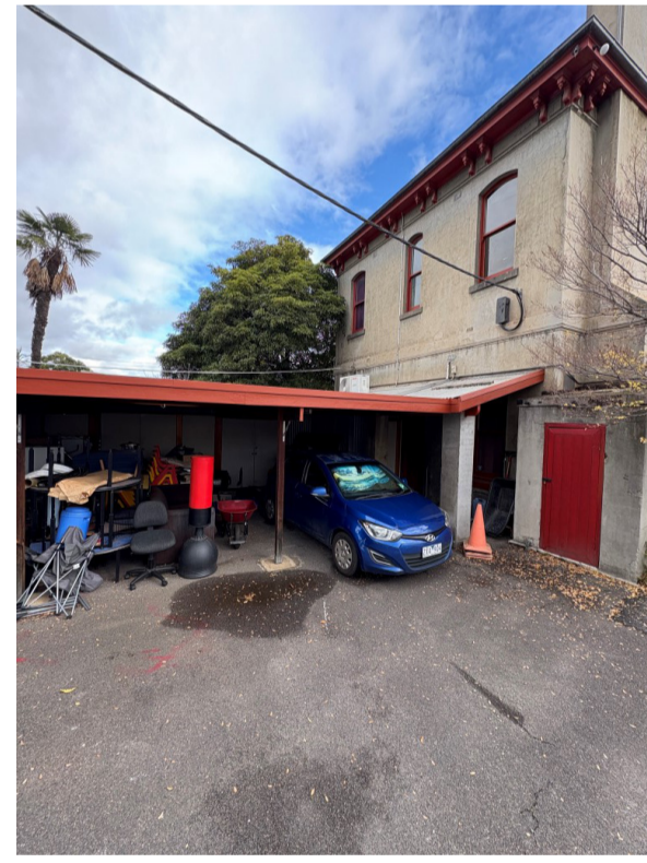
6. EXISTING CARPORT AND EASTERN VERANDAH
