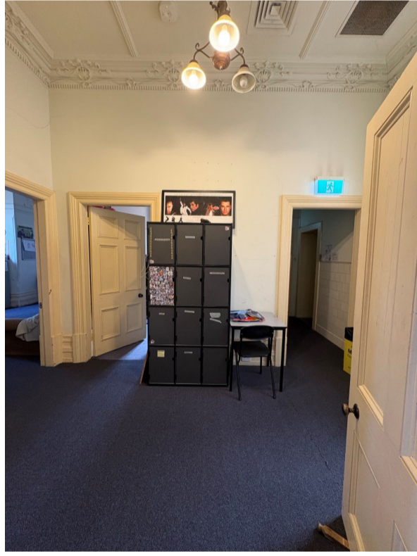
7. EXISTING DOOR TO FIRST FLOOR HALL
