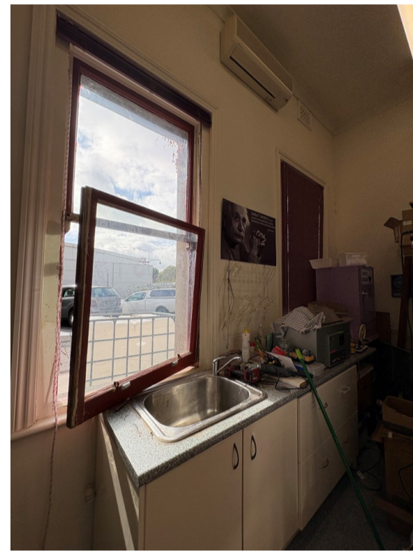
4. EXISTING NORTH WALL OF SCIENCE PREP
