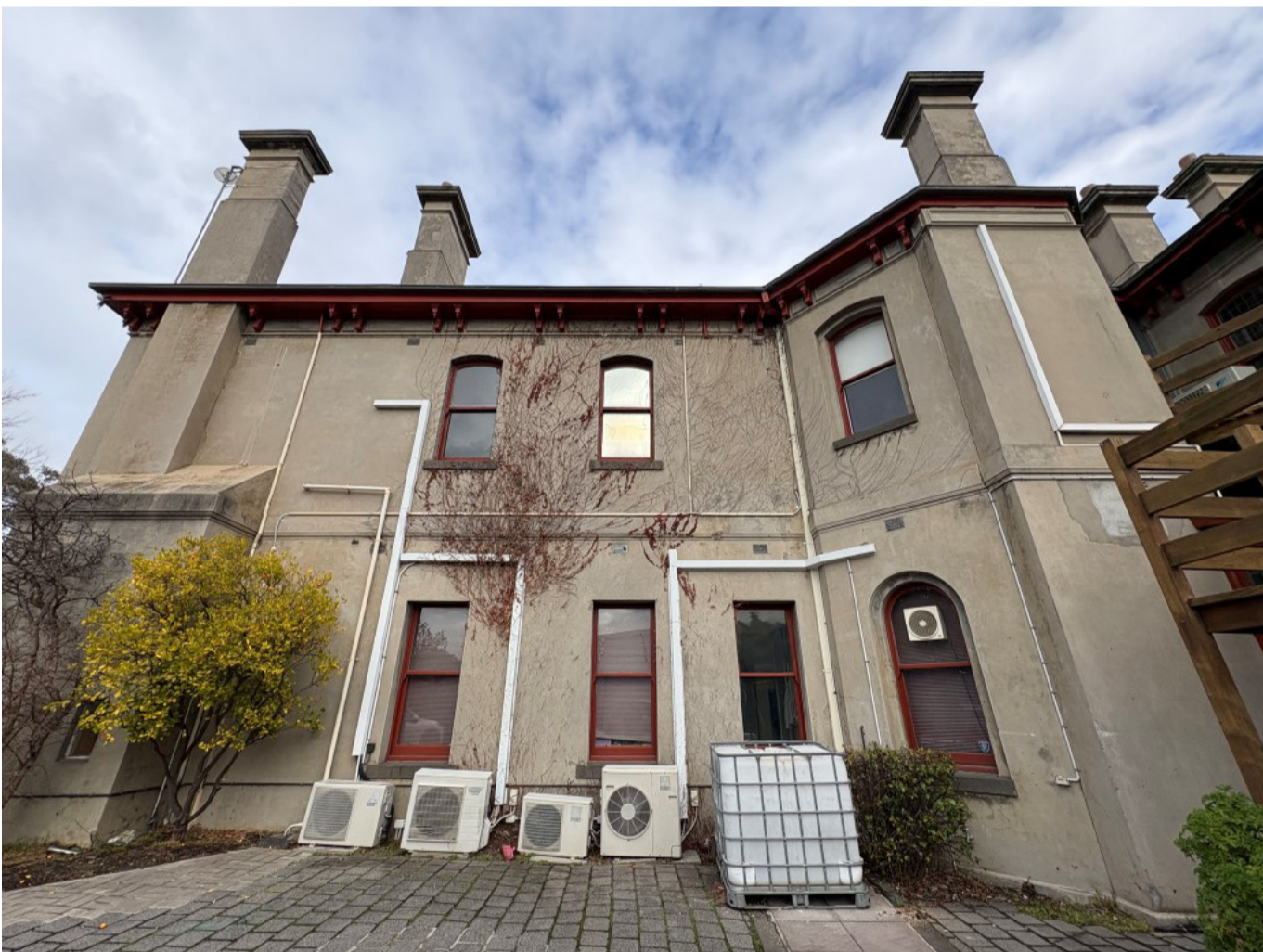
CARPARK-FACING FACADE (NORTH)
