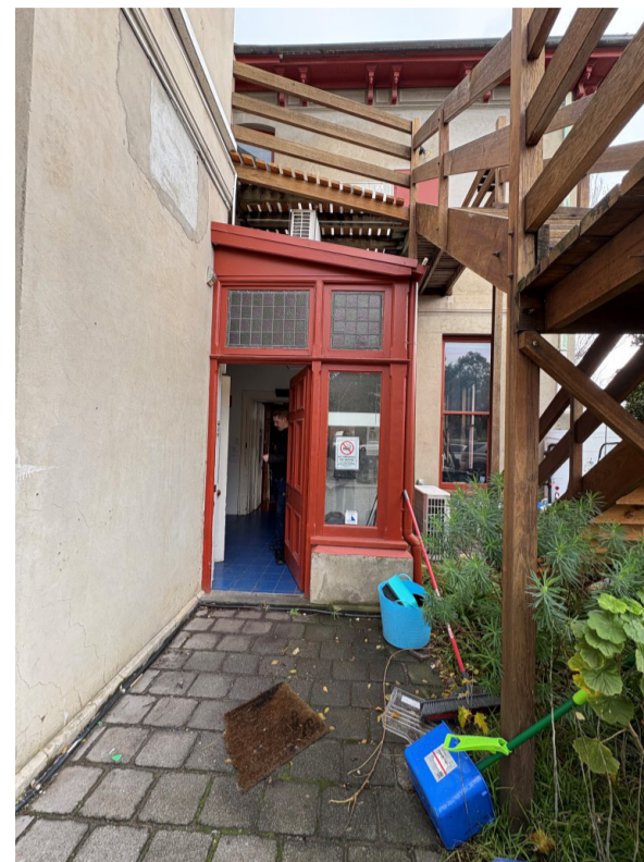
2. EXISTING AIR LOCK (EXTERIOR)
