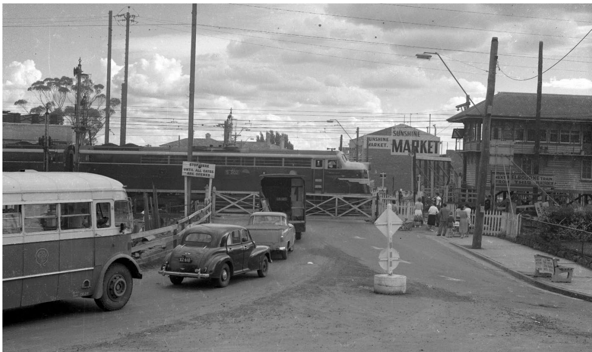
Figure 2: The level crossing at Hampshire Road, 1960. Facing south-west towards the Sunshine Market in the background. Signal box (extant) at right of frame. (DTP, historical pictures collection)
