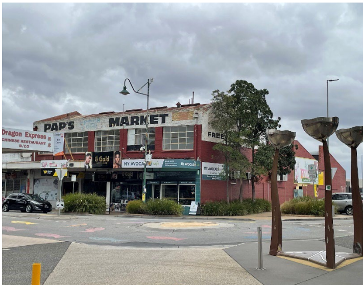
Former Sunshine Market from City Place, facing west
