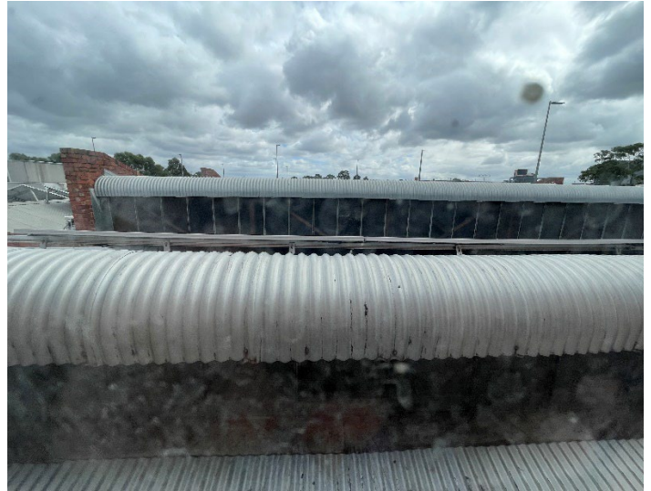
View from first floor rear window, looking onto the saw-toothed roof
