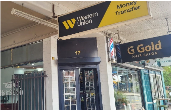
Arcade entry to market at left, with metal gate and two shop fronts. Note decorative pressed metal soffit
