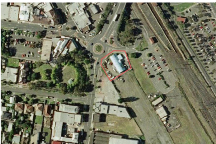
Figure 5: 2004, the eastern addition and entry structure has been added:
