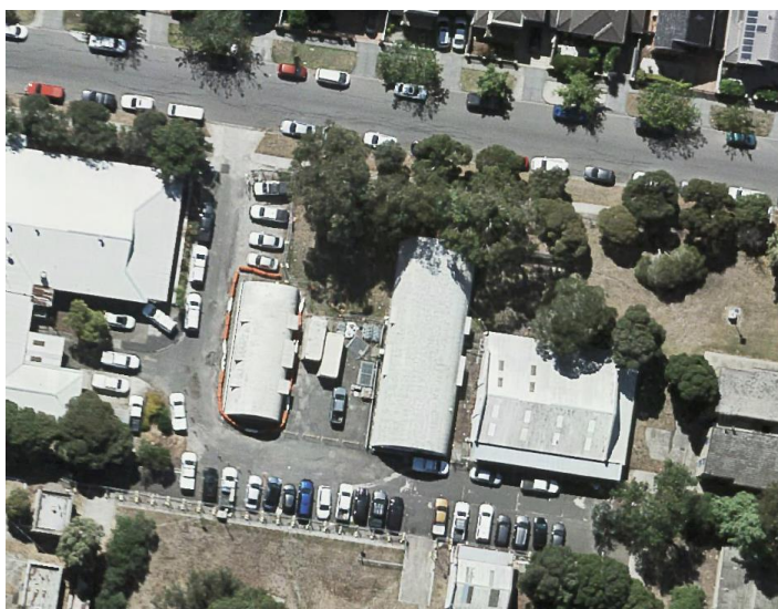
Figure 14: Part of the Former Maribyrnong Migrant Hostel site. The Nissen Hut at the centre left, the larger Romney hut centre right of image (Aerial imagery March 2025)
