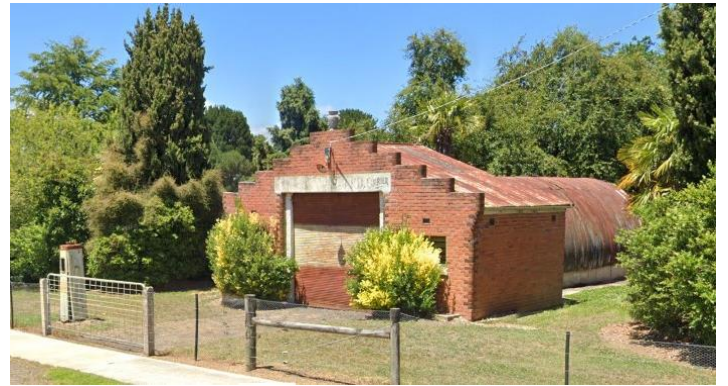
Figure 19: Howard's Carrying Depot, Former petrol station, Dean's Marsh, Surf Coast Shire, HO41 (Source: Google Streetview, December 2024)
