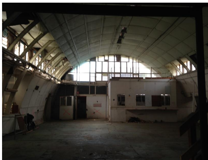
Figure 15: Interior Quonset Warehouse, Fletcher Jones Factory & Gardens (Heritage Victoria, file photograph 2014).
