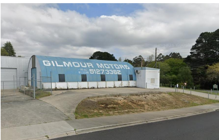
Figure 22: Gilmour Motors, Newborough, City of Latrobe (Source: Google Streetview, September 2023).
