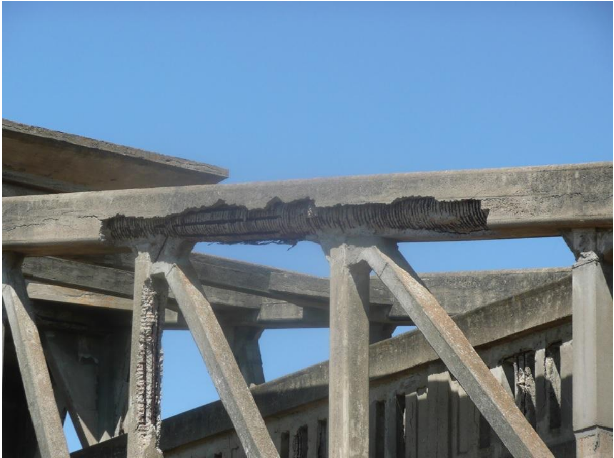
Figure 1: Example where concrete cover has 'spalled' and fallen away due to corroded internal steel reinforcement
