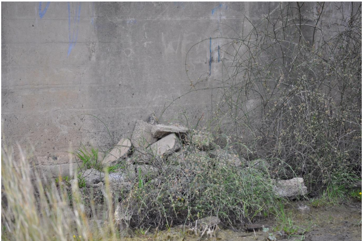
Figure 2: Brick-sized pieces of 'spalled' concrete that have fallen from the structure
