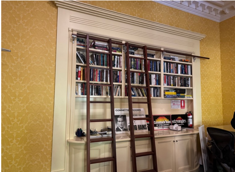
Figure 20 Original internal door opening in Room F2, infilled with a bookshelf/cabinetry.
