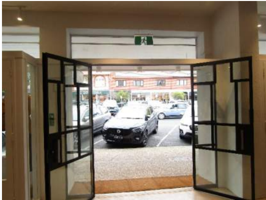
Figure 13 Entry doors with glazed highlight.
