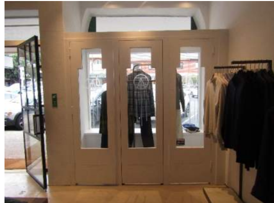
Figure 14 Original doors reconfigured as window display.
