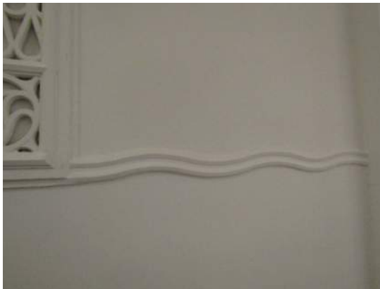
Figure 15 Dado moulding detail.
