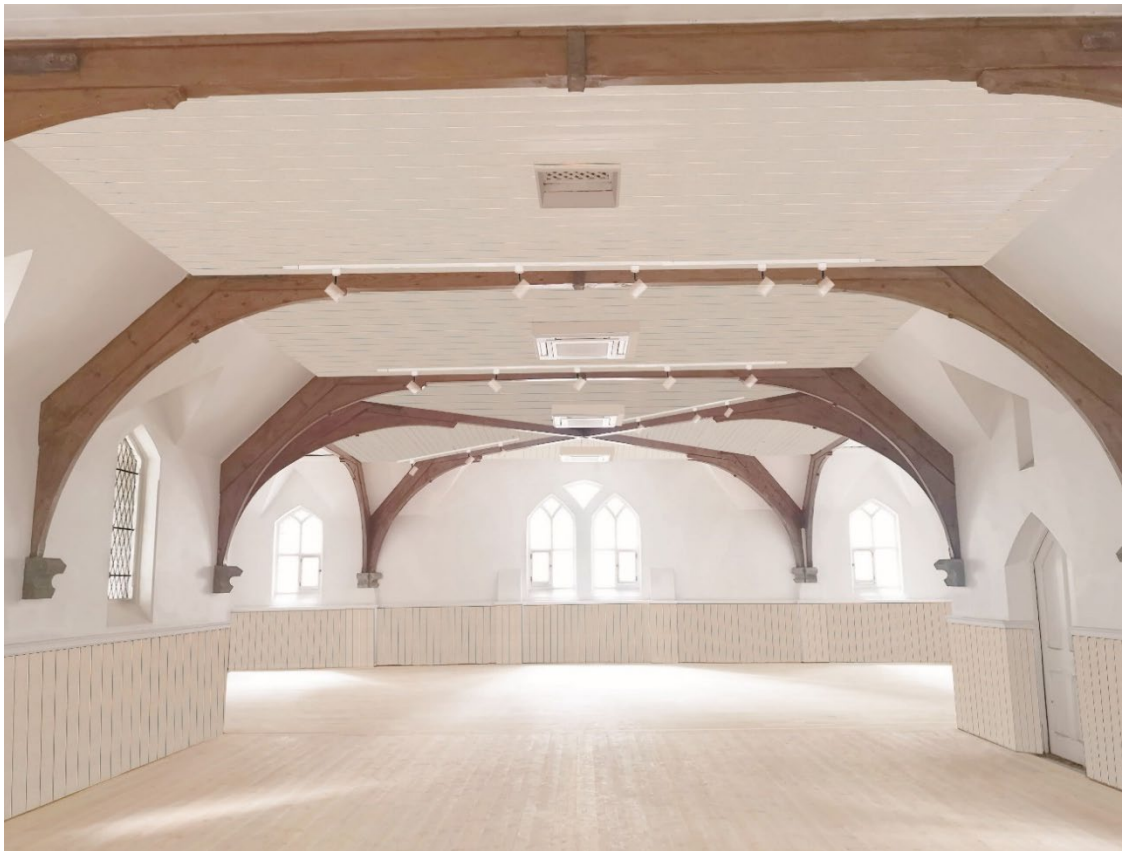
Figure 11 Montage of the lighting array set out parallel to the trusses, viewed to the south Source: Millar Architects
