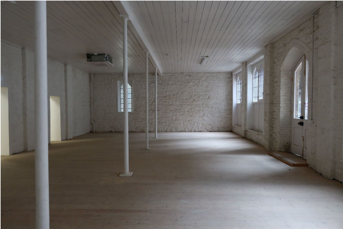
Figure 5 View to the east in the south wing of the ground floor; note modern openings to the dividing overpainted bluestone wall (at left) and cast iron columns
