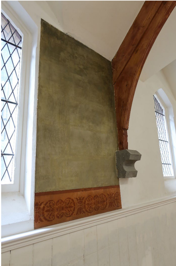
Figure 7 Exposed panel displaying early decorative scheme between a refurbished window and roof truss supported on a stone bracket
