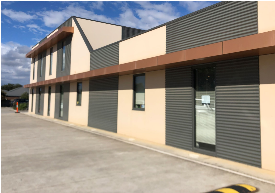
Figure 4 - Existing building at the rear
