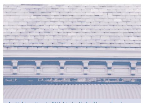
Spanish slates used to replace Welsh slates show bleeding of ferrous oxides and some delamination only 10 years after placement on this railway station roof.
