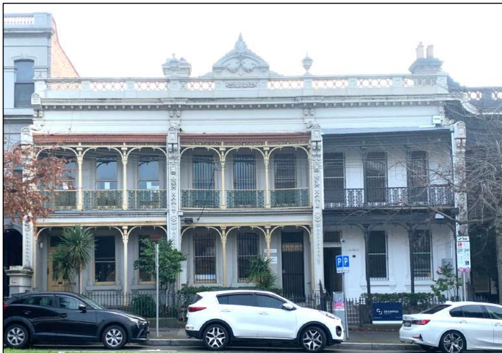
Figure 6 Burlington Terrace (left to right) 400, 398 and 396.
