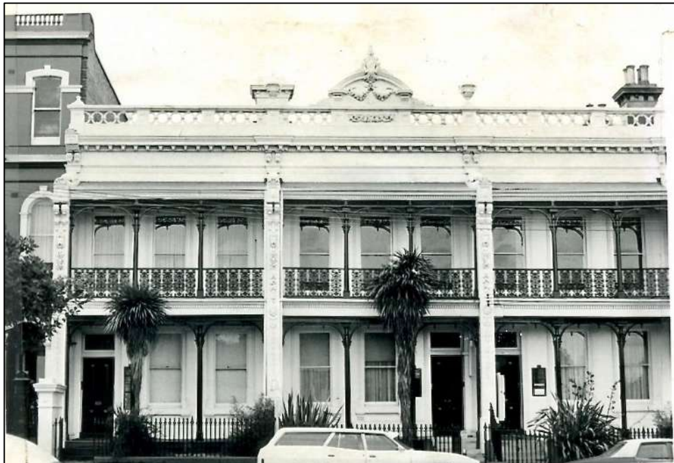
Figure 5 Burlington Terrace 1974, (left to right) 400-396 Albert Street, the subject site is the middle. Source: The East Melbourne Historical Society
