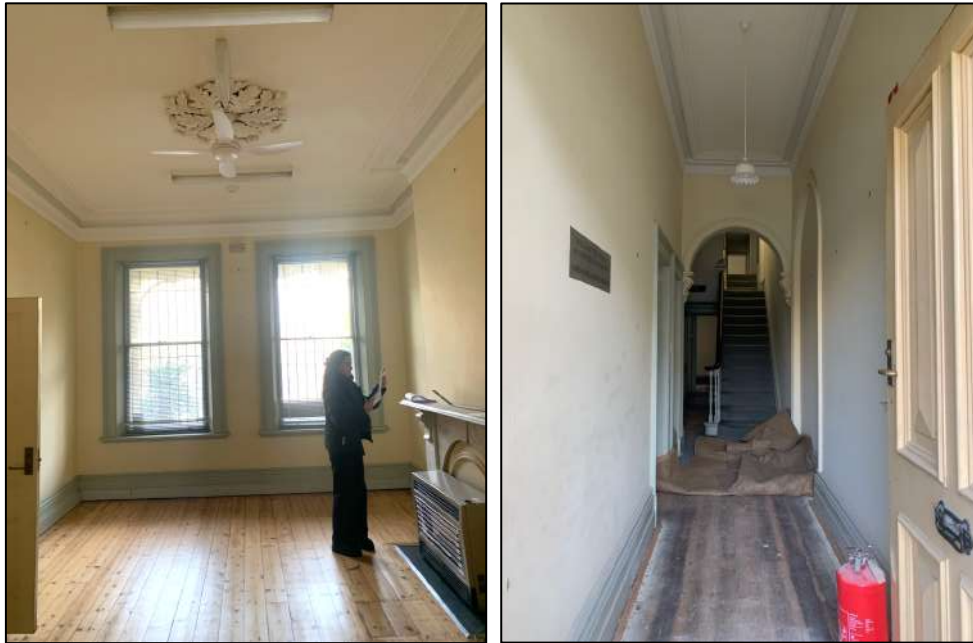
Figure 10 (left) View of the front room on ground level, (right) view of hallway front entrance.
