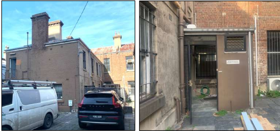
Figure 8 (left) View of the rear of the site, (right) rear entry to the property.
