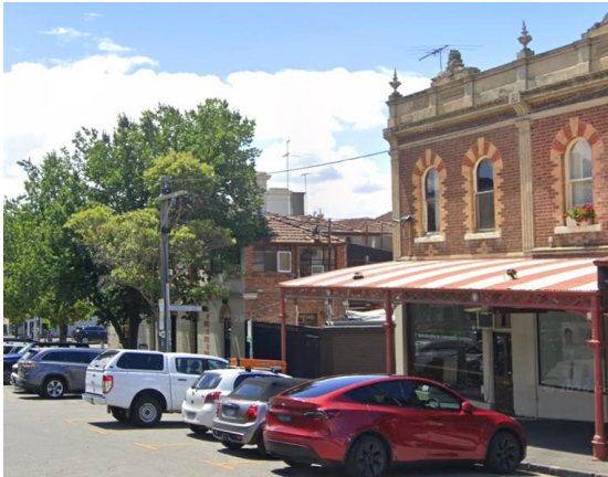
Figure 57: View to the west (rear) façade of the subject site, from South Melbourne Town Hall. Source: Google Street View, 2026.
