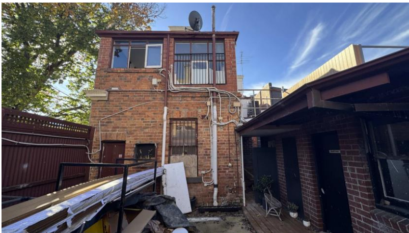
Figure 23: External view of the rear of the northern terrace, with toilets and storerooms to the right. Source: Trethowan Heritage, 2026.
