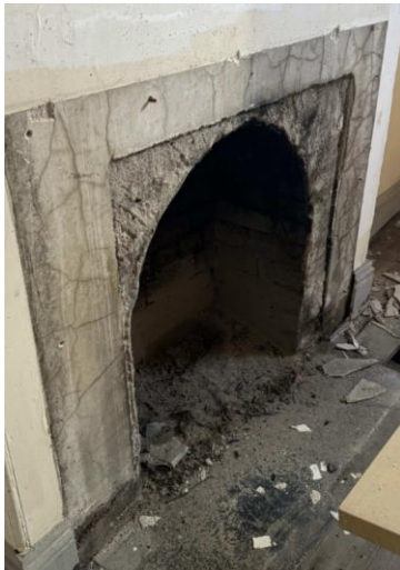
Figure 42: View of the southernmost premise, rear room's exposed fireplace stripped of decoration. Source: Trethowan Heritage, 2026.
