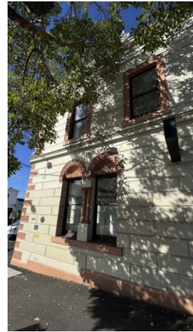
Figure 15: View of the Bank Street (north) façade. Source: Trethowan Heritage, 2026.
