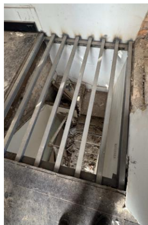
Figure 33: View of the northernmost premise's floor opening, previously a staircase connecting the ground floor. Source: Trethowan Heritage, 2026.
