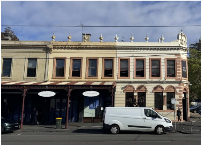
Figure 14: View of the Clarendon Street (east) façade. Source: Trethowan Heritage, 2026.
