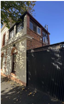
Figure 16: View of the Bank Street (north) façade. Source: Trethowan Heritage, 2026.
