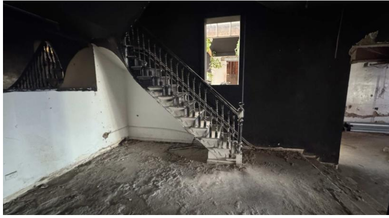
Figure 28: View of the southern terrace's timber staircase. Source: Trethowan Heritage, 2026.
