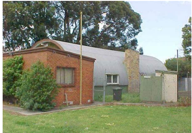
Figure 34. Former 1st Strathmore Scout Hall, Strathmore, dated 24 October 2003. (Source: Hermes; copyright Moonee Valley City Council)
