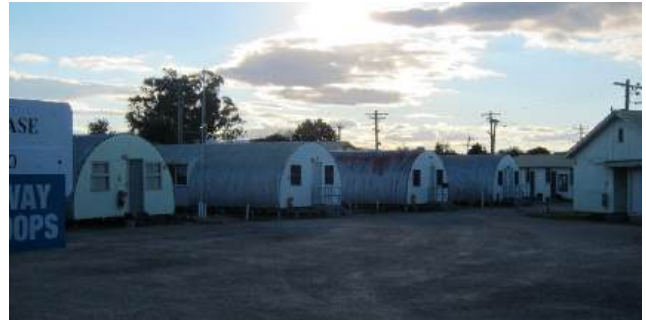
Figure 32. Nissen Huts at Beersheba Barracks, Wangaratta. (Source: Hermes; image by Context)
