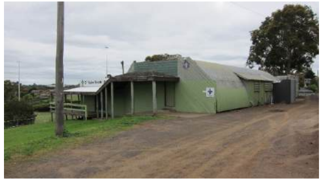
Figure 47. 5 th Keilor Scout Hall, 2013. (Source: City of Moonee Valley Heritage Gaps Study Stage 1, Context Pty Ltd)
