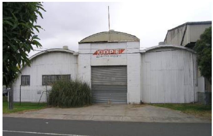
Figure 37. Standard Steel building [undated]. (Source: Hermes)
