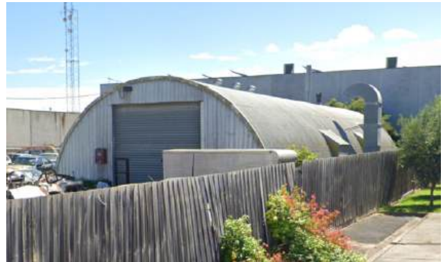
Figure 49. Single Nissen hut remaining from Williamstown Migrant Hostel. (Source: Google Street View, dated January 2023)
