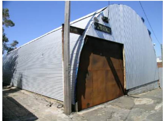
Figure 43. Prefabricated arched hut, Clifton Hill, 2010. (Source: Hermes)
