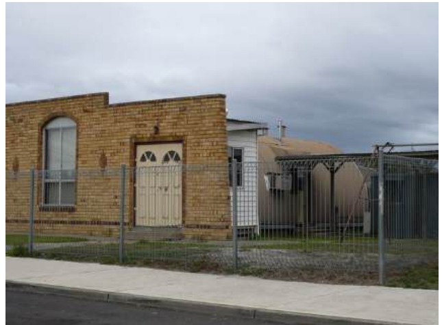
Figure 46. Wesleyan Methodist Church Hall, 2010. (Source: Hermes, copyright Context Pty Ltd)
