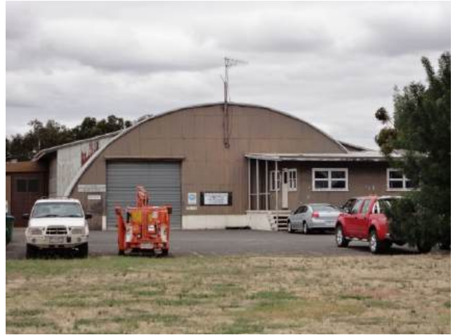
Figure 45. Quonset Hut, 46 Kalkee Road, Horsham, 2011. (Source: Horsham Rural City Council Heritage Study Stage 1, Grieve Gillett & Associates, June 2012)
