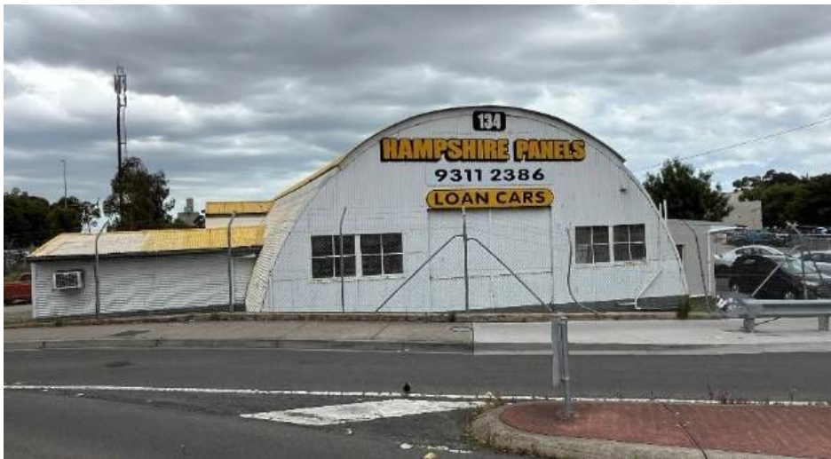
Figure 26. 134 Hampshire Road, Sunshine, looking south from opposite side of City Place to the northern elevation of the building. (Source: GJM Heritage, November 2025)
