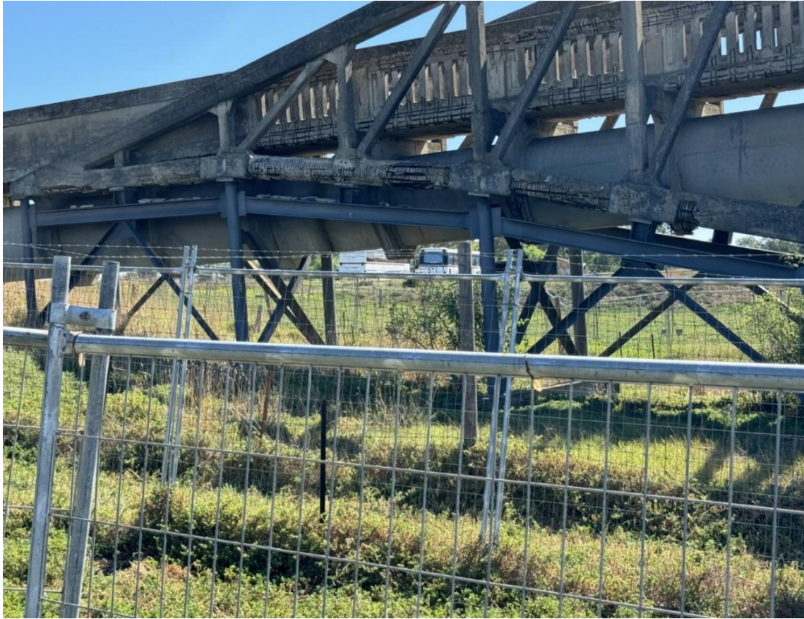
Image Showing Spalling and Concrete Pieces on top of Steelwork Propping Southern Spans
