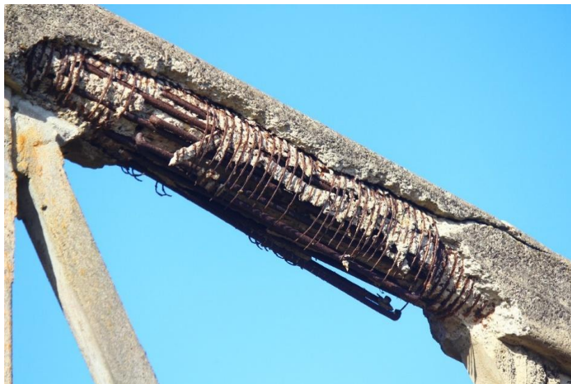
Photograph showing Spalled Concrete and Corroded Reinforcement to Truss Bottom Chord (Compression Member) and Truss Top Chord (Tension Member)
