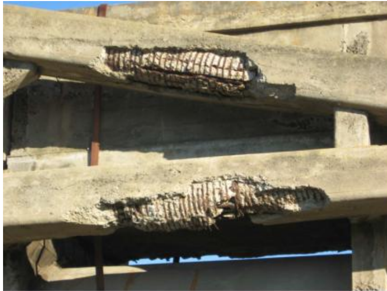
Photograph showing Spalled Concrete and Corroded Reinforcement to Truss Bottom Chord (Compression Member) and Truss Top Chord (Tension Member)
