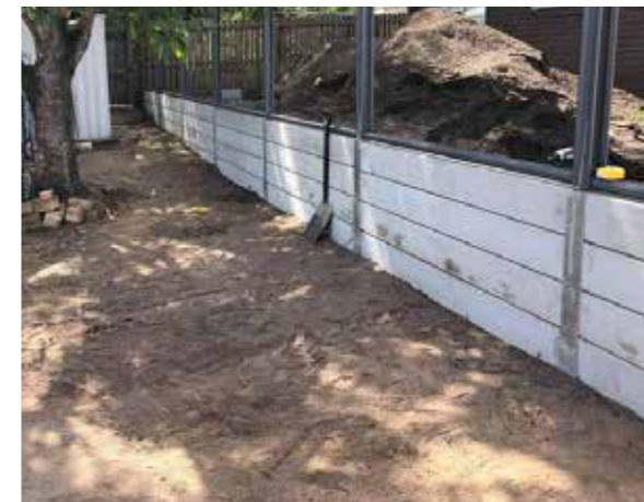
'Fence Connectors' allow display walls to be easily assembled and disassembled to move material in and out of the horticultural display areas
