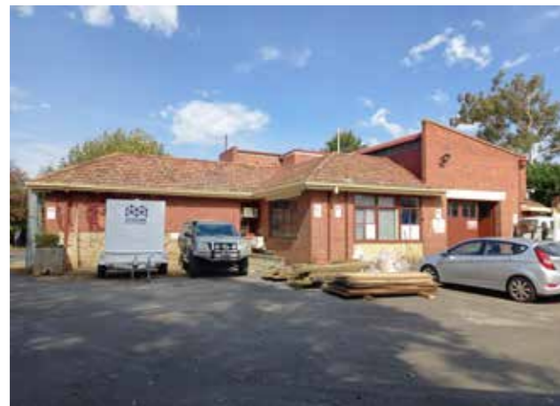
Existing site photo
