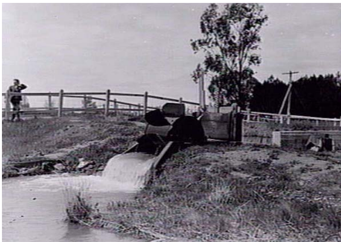
Irrigation channel at Rochester showing a Dethridge Meter Wheel
