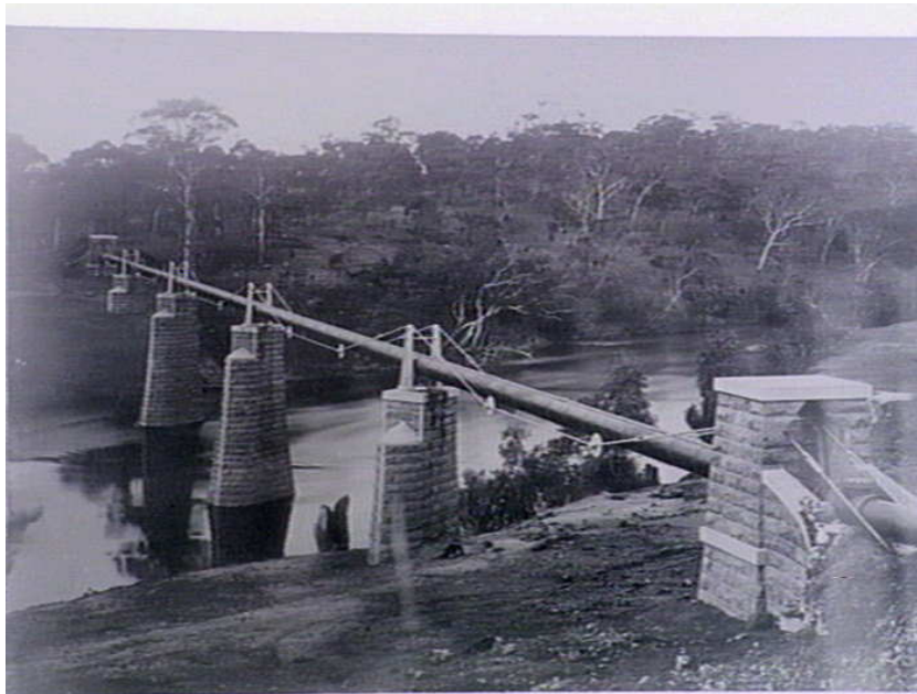
Flume carrying the 'high-level' pipe over the Yarra River at Kew
