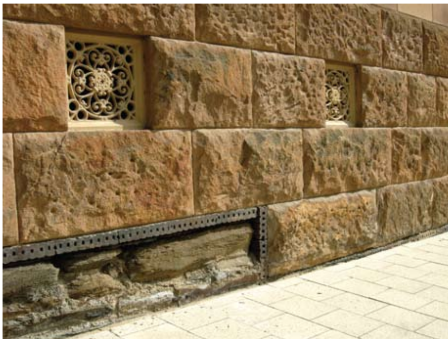
Figure 34 Stonework below the DPC needs attention as salts accumulate and the mortar and bluestone erode. In the first instance sacrificial treatments should be used to manage the problem. The 1879 ceramic DPC is doing an excellent job of protecting the sandstone above it, although where it steps down the slope it is compromised by hard paving that is laid too high, allowing splash onto the stone (see Box 2: Location of DPCs ).
