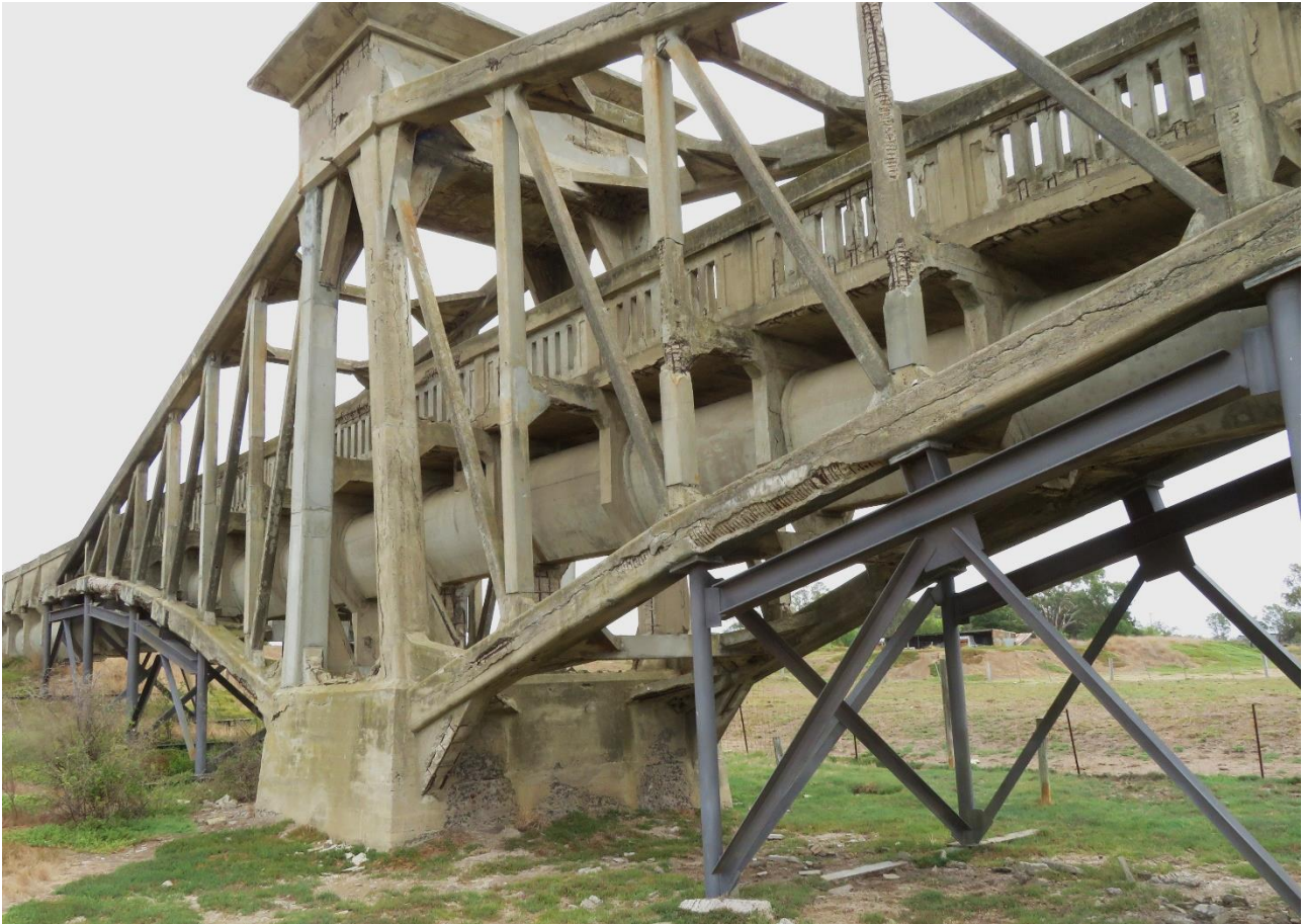
Figure 14 Truss 14 (south end of Aqueduct) with permanent propping installed c. 1991, exposed steel reinforcement, cracks, repaired and recast pier leg and web members, failed patch repairs Source: Lovell Chen archives (photographed 2019)
