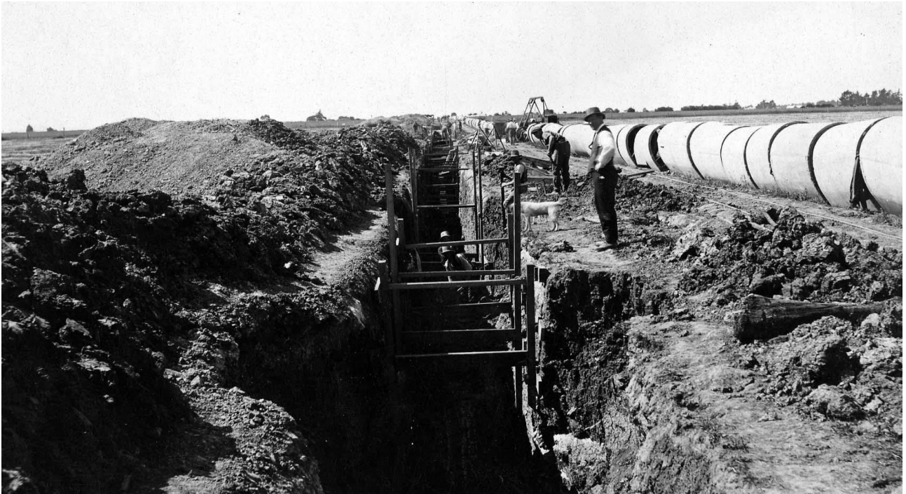
Figure 8 Trenching for the installation of the Geelong Outfall Sewer, c. 1912-1914, with ovoid sewer pipe manufactured by Stone & Siddeley lined up alongside the trench for installation Source: Barwon Water archives
