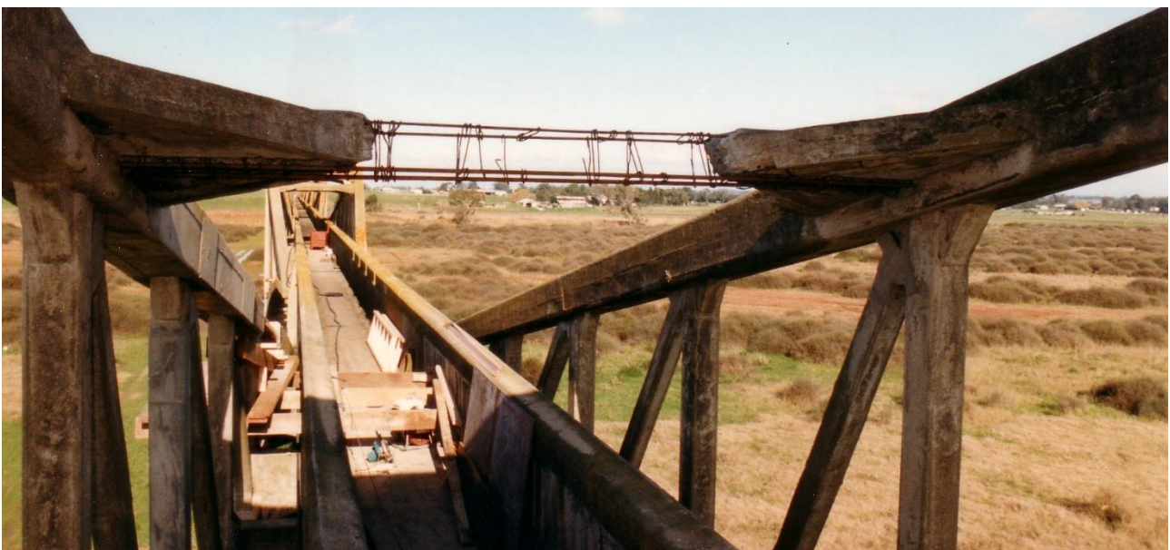
Figure 13 Recasting of a truss cross-brace beam while the structure remained in service, likely c. 1984; freshly repaired or recast sections are also seen just behind it on the truss top chord and vertical member at left Source: Barwon Water archives
