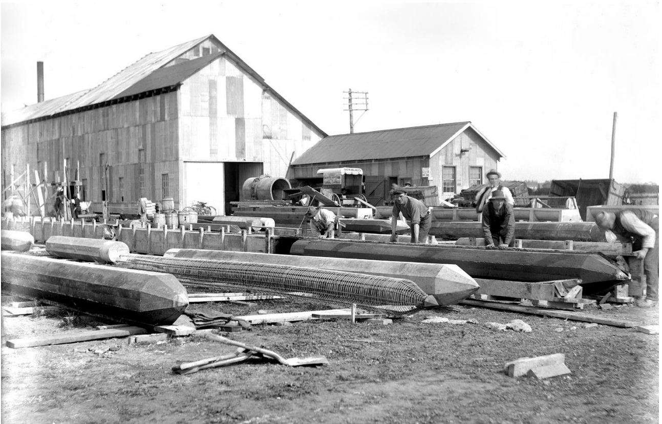
Figure 9 Manufacturing of Aqueduct's precast concrete piles at Stone & Siddeley's Marshall Pipe Factory, 1913 Source: Barwon Water archives
