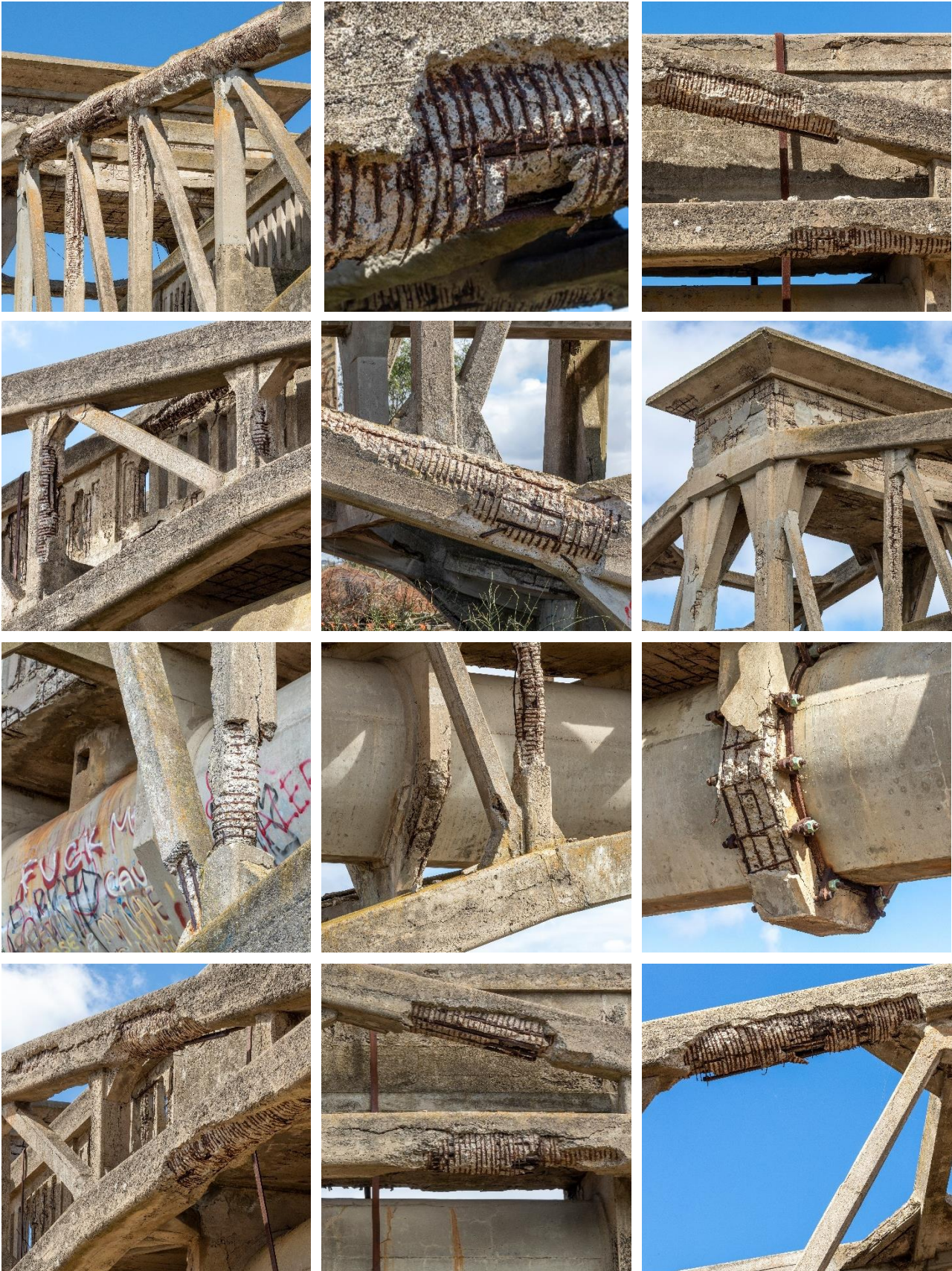
Figure 16 Example deterioration of the concrete cover and underlying steel reinforcement across the Aqueduct Source: Glasshouse Creative Media (2022), courtesy Barwon Water
