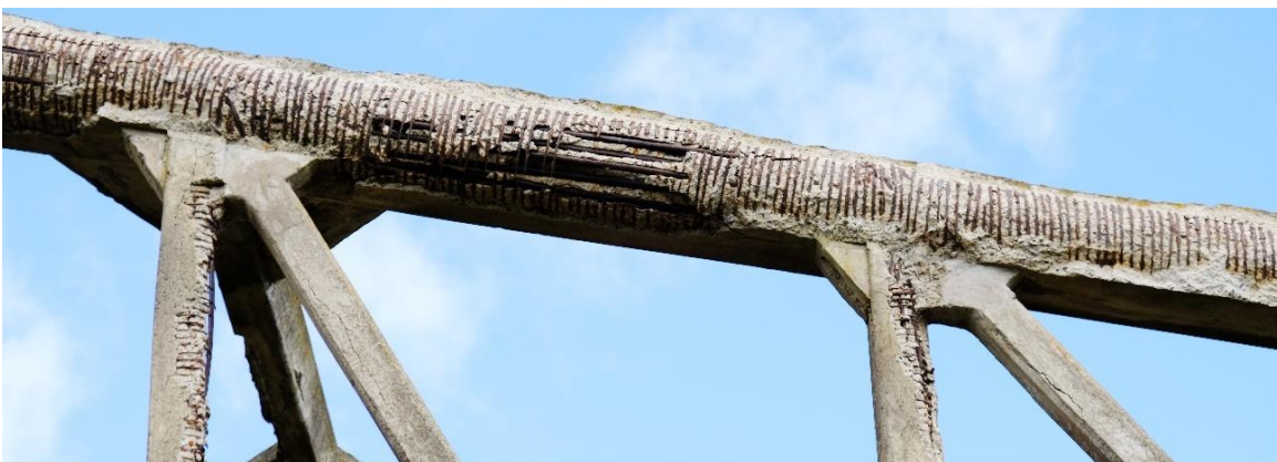
Figure 7 Example of advanced degradation of an upper chord and adjoining vertical members and crossbeam Source: Lovell Chen archives, photographed 2019
