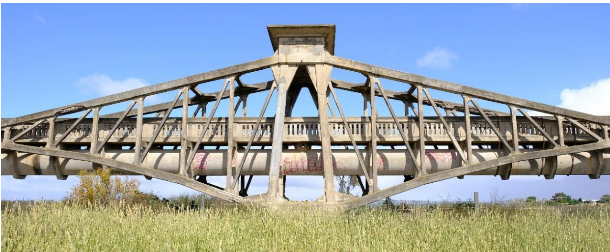
Figure 6 Typical pier and truss span; upper chord and diagonal web members are held in tension, while the lower chord and vertical web members are subject to compression forces Source: Lovell Chen archives, photographed 2019
