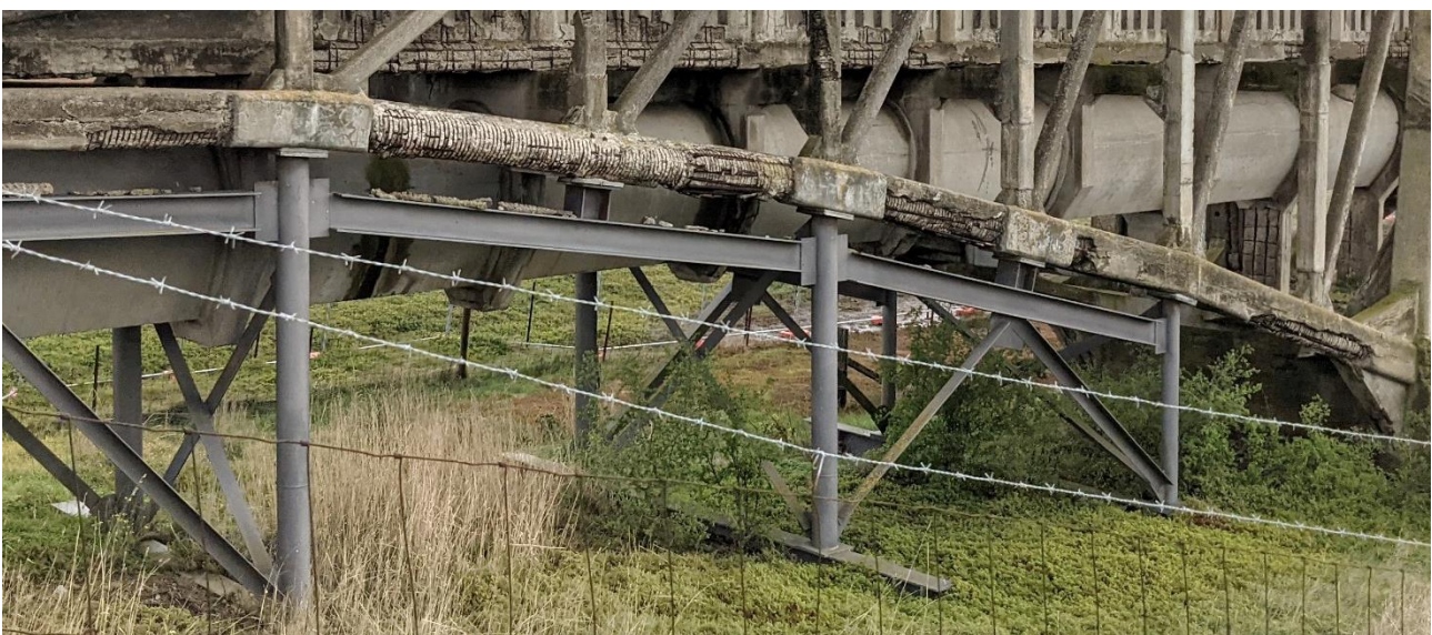
Figure 15 Detail of propped Bottom Chord on Truss 14 with exposed and buckled steel rods, apparent deflections and extensive concrete spalls accumulated on top of the c. 1991 steel props Source: Lovell Chen archives (photographed 2021)
