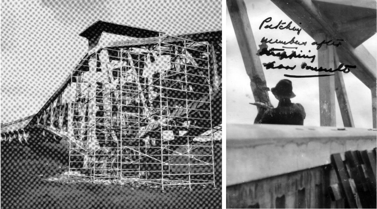
Figure 12 Historical photographs of concrete repair works, possibly those specified by E.G. Stone in 1924 Source: Barwon Water archives
