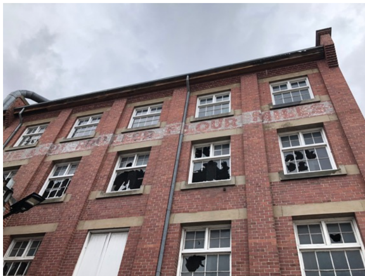
Figure 7: Replace broken glazing to prevent water and birds entering the building. Source of image: Peter Andrew Barrett Collection.
