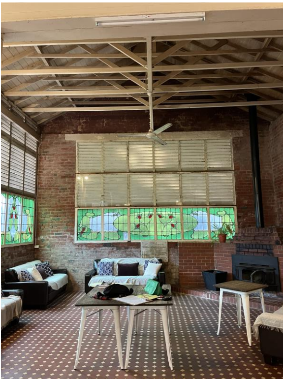
Image 6 View of the eastern transept with tiles and fireplace of later date, note the significant efflorescence and evidence of penetrating damp in this area
