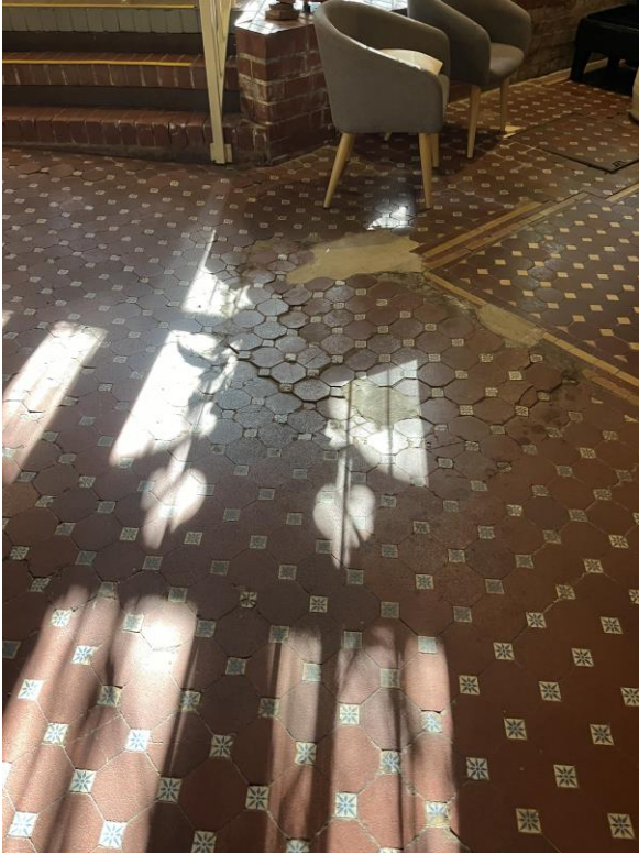
Image 5 Example of more significant settlement and undulation to original encaustic tiles at the base of the stairs adjoining the eastern transept
