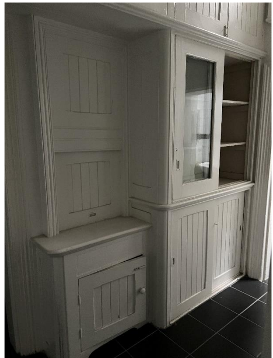
Figure 19 Timber joinery beneath the stairs and within the servery, including a dumb waiter
