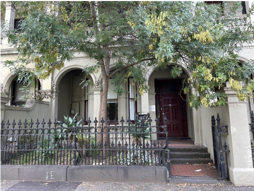
Figure 13 Ground level presentation of no. 95 including the fence, tessellated tile path and verandah and timber door case/bay window
