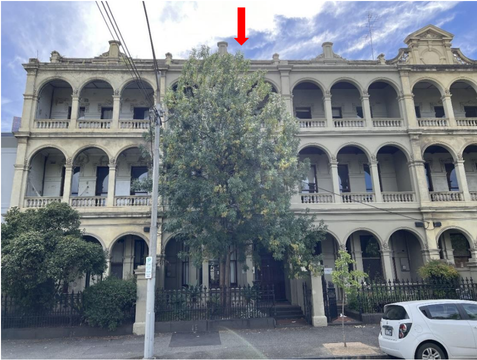
Figure 12 95 Drummond Street, showing tree in front garden bed which screens the view of the façade
