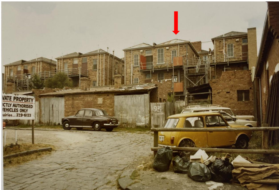
Figure 8 Rear elevation of Drummond Terrace with later (since replaced) fire stair. No. 95 (indicated) has multi-pane windows that have since been replaced Source: Anglican Diocese of Melbourne Archives
