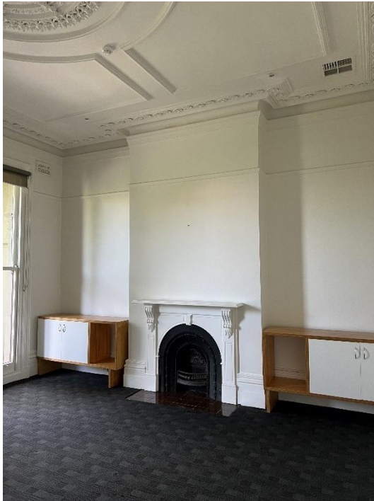
Figure 26 Front room to first floor level showing timber mantle to fire place and plaster ornamentation to ceiling and cornice
