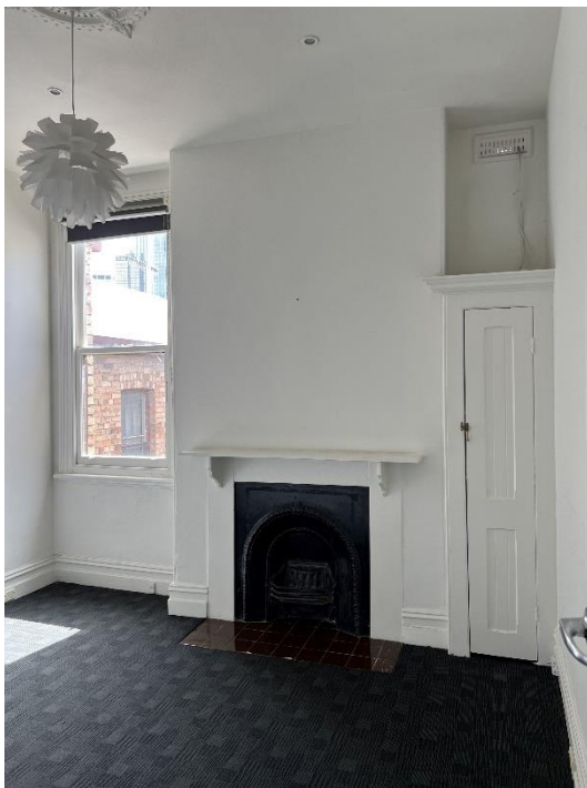
Figure 27 One of the front rooms showing simple timber mantle and timber joinery (left) and storage room at second floor level
