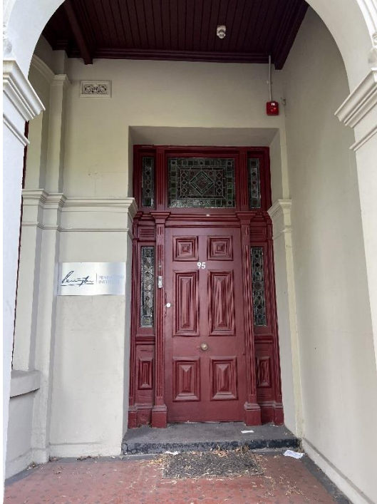
Figure 14 Timber door case showing stained glass side lights and fanlight
