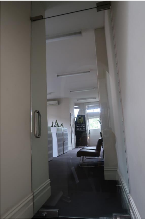
Figure 29 Frameless glass doors installed to define the office tenancies in no. 99
