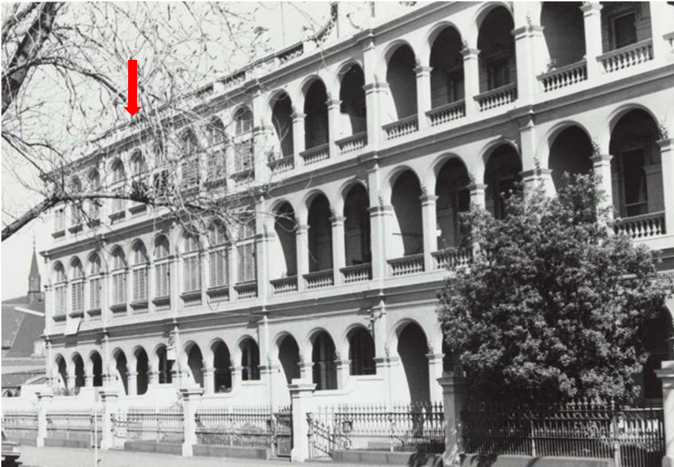
Figure 6 Drummond Terrace, dated 1976. The subject site with infilled balconies is indicated Source: SLV image no H94.200-62
