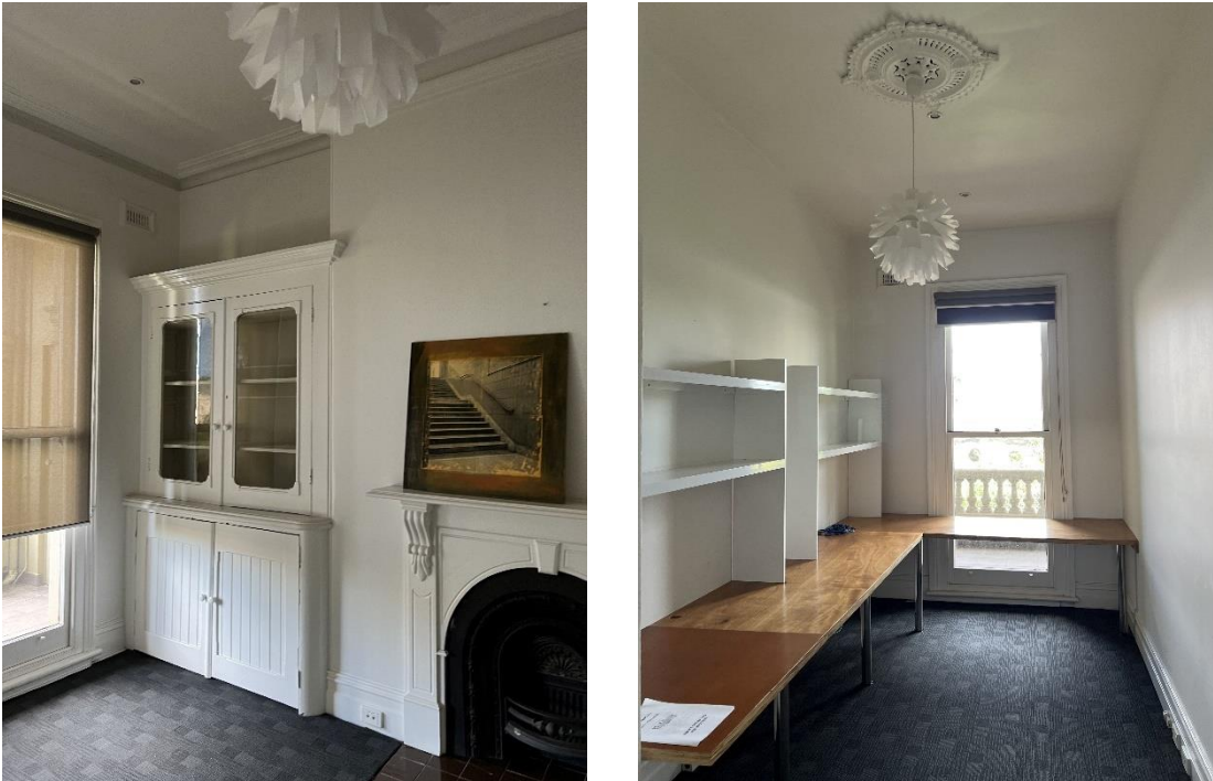
Figure 28 Front rooms to second floor levels showing inbuilt timber joinery (left) and altered front room/space, noting the lack of cornice (right)
