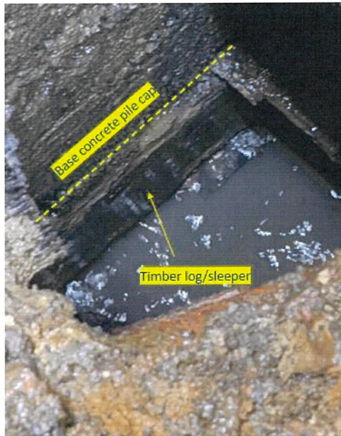
Concrete in pile cap appears to be in good conditions with no obvious cracking/defects. Difficult to assess condition of timber but looks to be relatively well preserved
