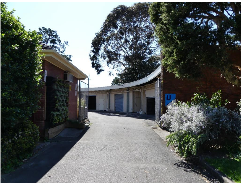
Figure 19 View to the eastern end of the Ambulance Garage and driveway, Staff Quarters on left Source: Lovell Chen, 2021
