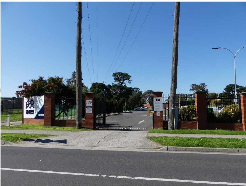
Figure 11 View from Yarra Bend Road looking east to the existing boundary fence and carpark access Source: Lovell Chen, 2021
