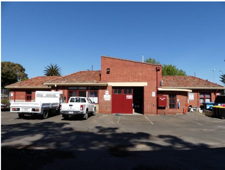
Figure 17 View from the Ambulance Garage driveway to the north elevation of the Staff Quarters Source: Lovell Chen, 2021
