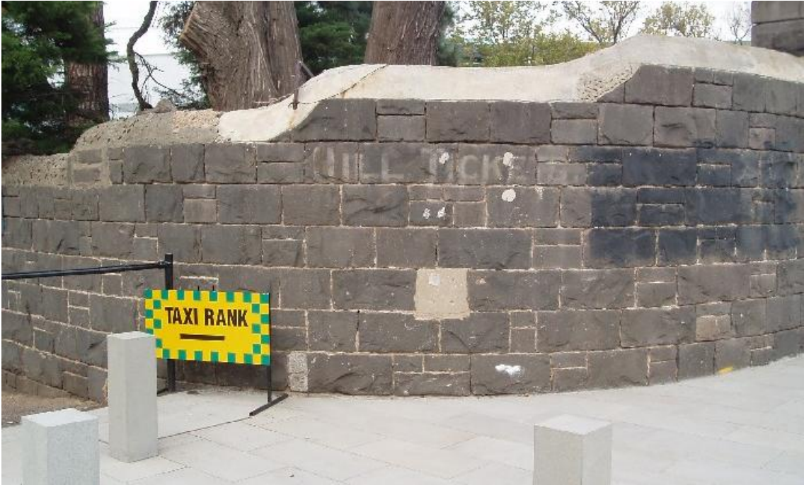
Figure 44 Bluestone wall at Hill Entrance with original 'Hill Ticket Box' painted signage.
