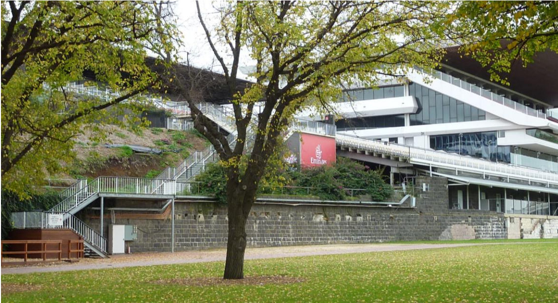
Figure 38 Base of the 1870s/80s bluestone stand. Note the Old Hill Stand above.
