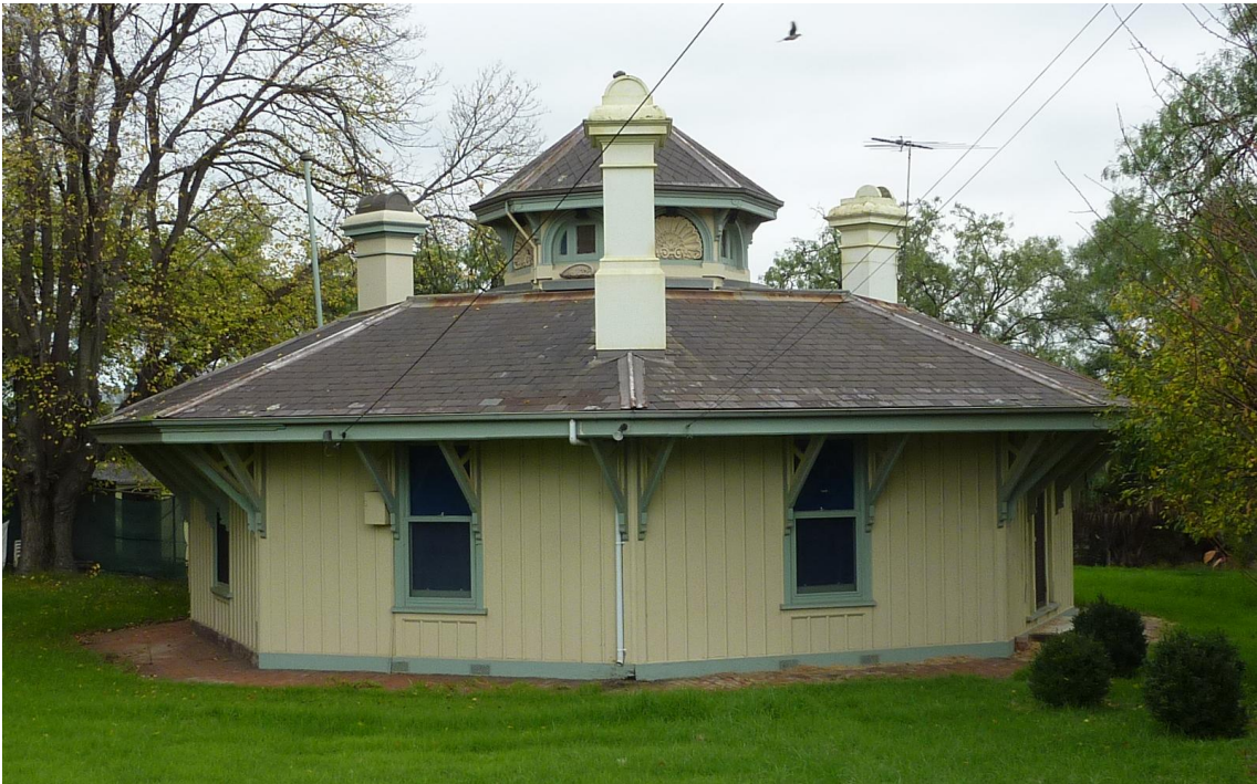
Figure 54 Jockeys' Convalescent Lodge, viewed from the north.
