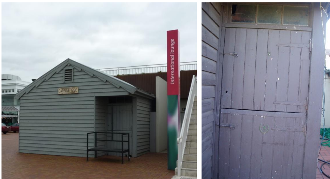
Figure 52 Left: Carbine's stall viewed from the south. Right: Detail of stall door, with tripartite lights above.
