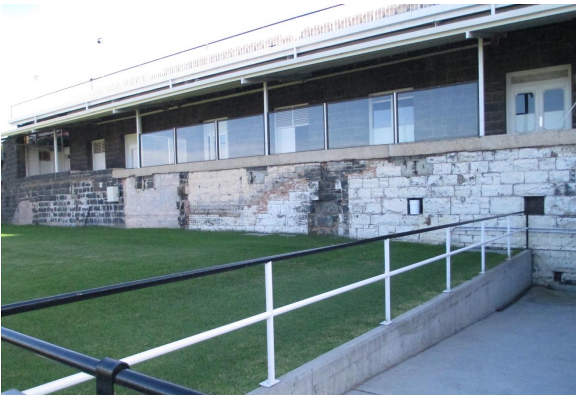
Figure 39 Remnant bluestone stand, showing the bluestone wall at ground level, bluestone building at level 1, and modern terraced seating above.
