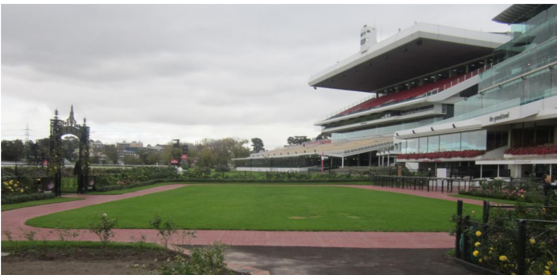
Figure 68 Looking west across the mounting yard.
