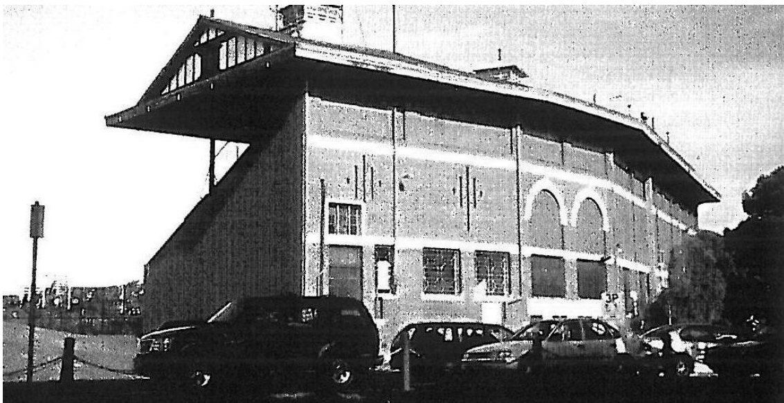
Figure 94 Grandstand at the Lakeside Oval, South Melbourne.
