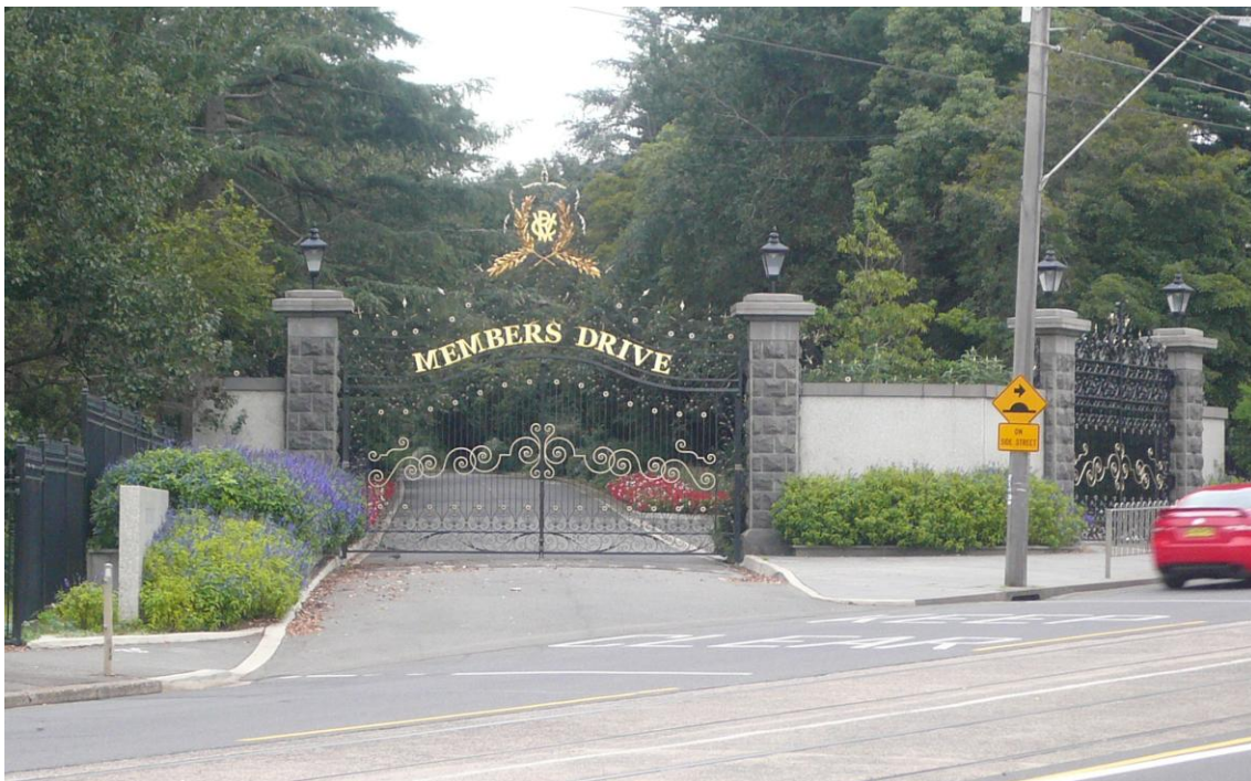
Figure 50 Members Drive entrance from Epsom Road. Note the existing bluestone piers (which date from 2007) and entrance gates do not form part of the significance of the Members Drive.
