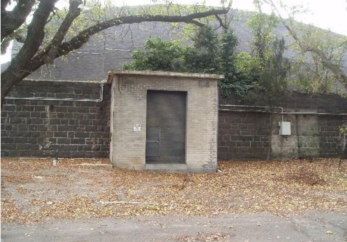
Figure 45 Bluestone wall with remnant horse tethering rings.
