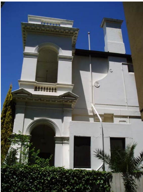
Figure 22 The eastern end of the north elevation.
