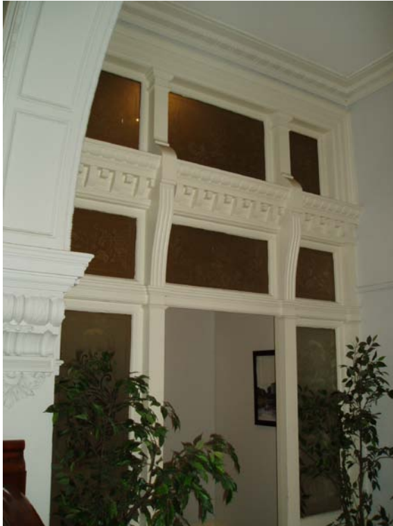
Figure 27 The glazed timber screen at the northern end of the main hall, ground floor.
