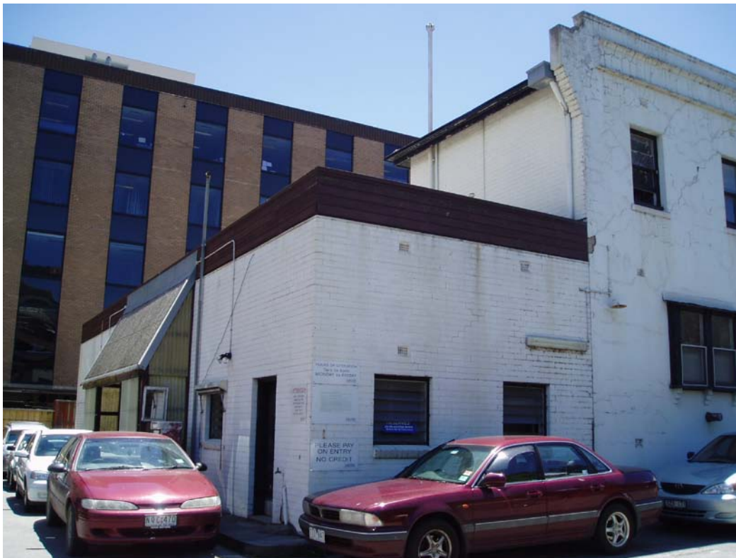
Figure 24 The west and south elevations of the 1954 additions.
