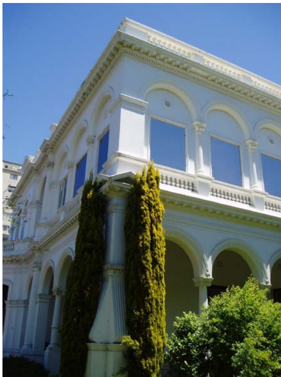
Figure 19 The enclosed south-eastern loggia.
