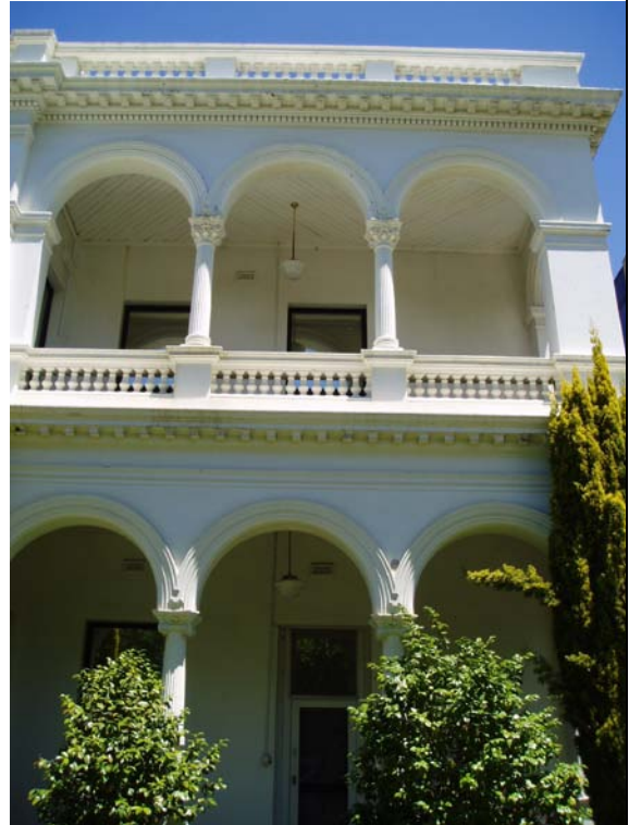
Figure 18 East elevation, the northern verandah and loggia.
