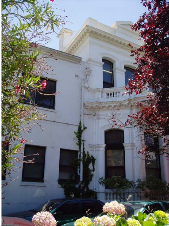
Figure 14 South elevation, junction of the 1930 wing and 1891 mansion.
