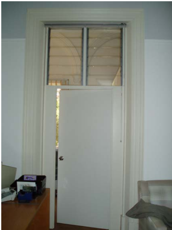
Figure 35 Modified opening between room F12 and the enclosed loggia.
