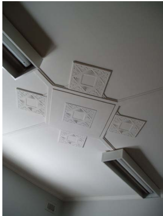
Figure 40 Typical decorative ceiling to a sitting room in the 1930 wing.
