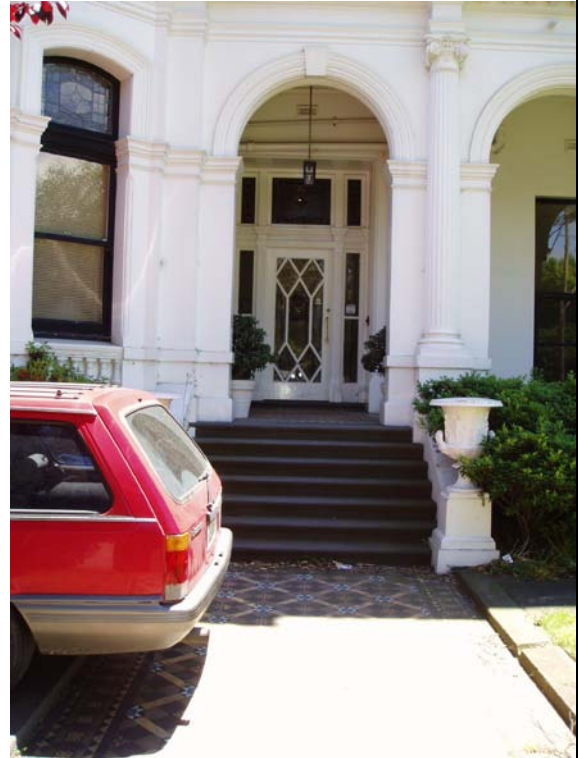
Figure 15 South elevation, entrance.
