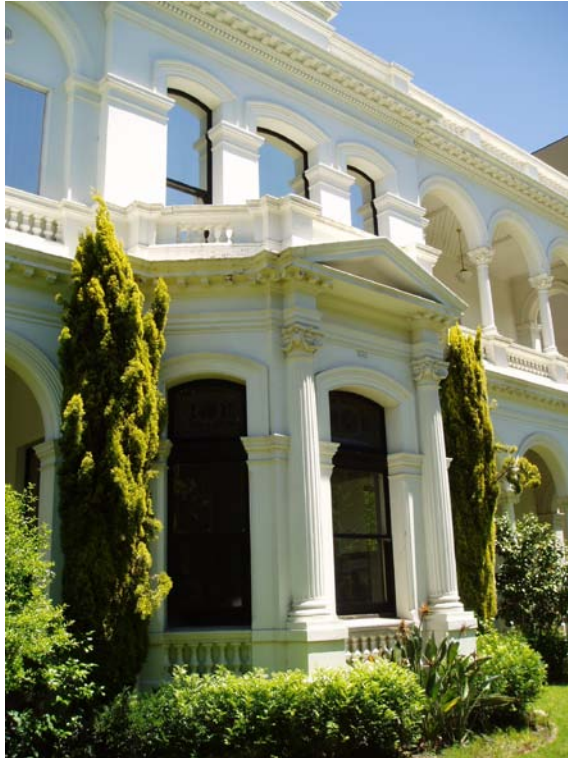
Figure 17 East elevation, the canted and breakfront central bay.
