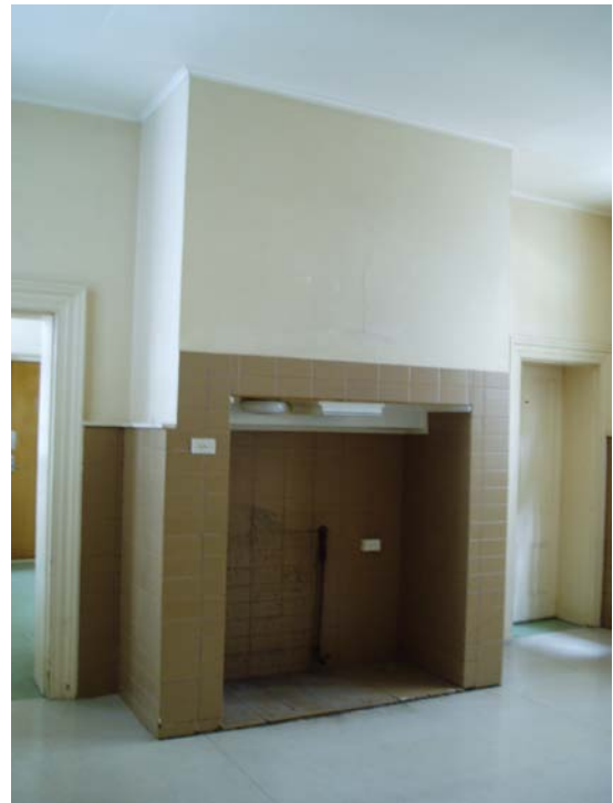
Figure 38 The chimneybreast to the kitchen range, room G10.
