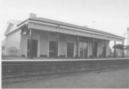
Williamstown Railway Station is a well restored and maintained public building.
