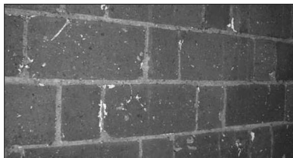
*Damage to brick surface as a result of inappropriate sandblasting*
