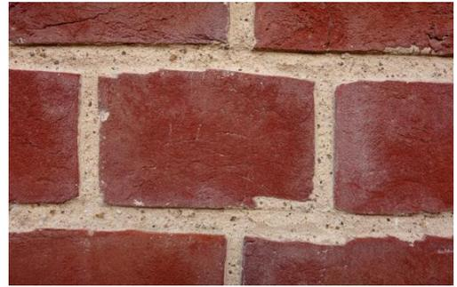
This photo illustrates damage to bricks from the use of angle grinders to cut out old mortar.
