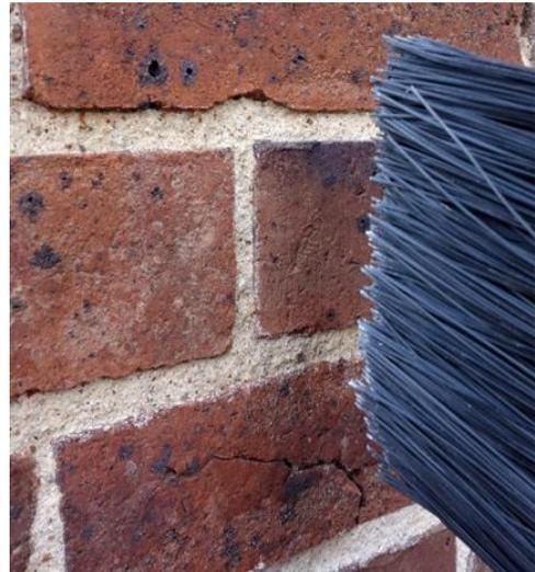
Tamping the surface with a stiff-bristled brush compacts the mortar, exposes the colour and texture of the sand grains and produces a weathered appearance. Tamping is undertaken when the joint surface is still leather hard—when a fingernail can just be pushed into the mortar.
