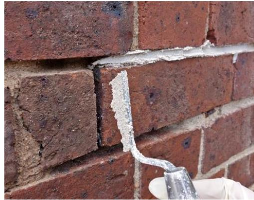
Caulking or finger trowels in a range of widths that fit snugly into the joints are a critical part of repointing. Here a wedge of stiff mortar is being inserted into a narrow perpend joint with a 4 mm wide trowel.
