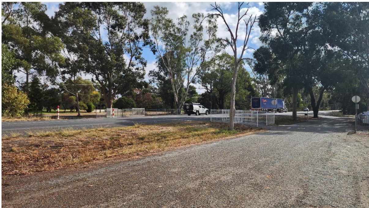
Figure 9: School crossing on Goulburn Valley Highway.
