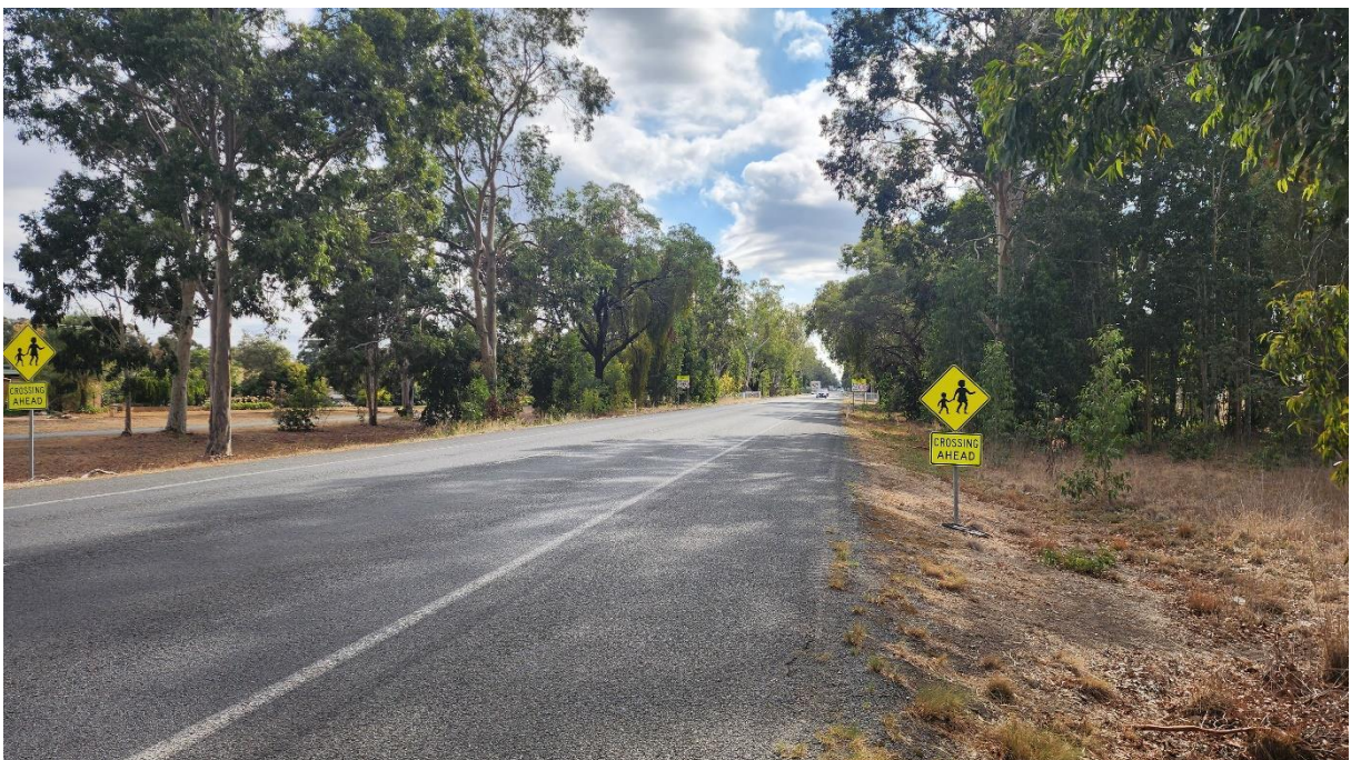
Figure 5: High retention trees along Goulburn Valley Highway.
