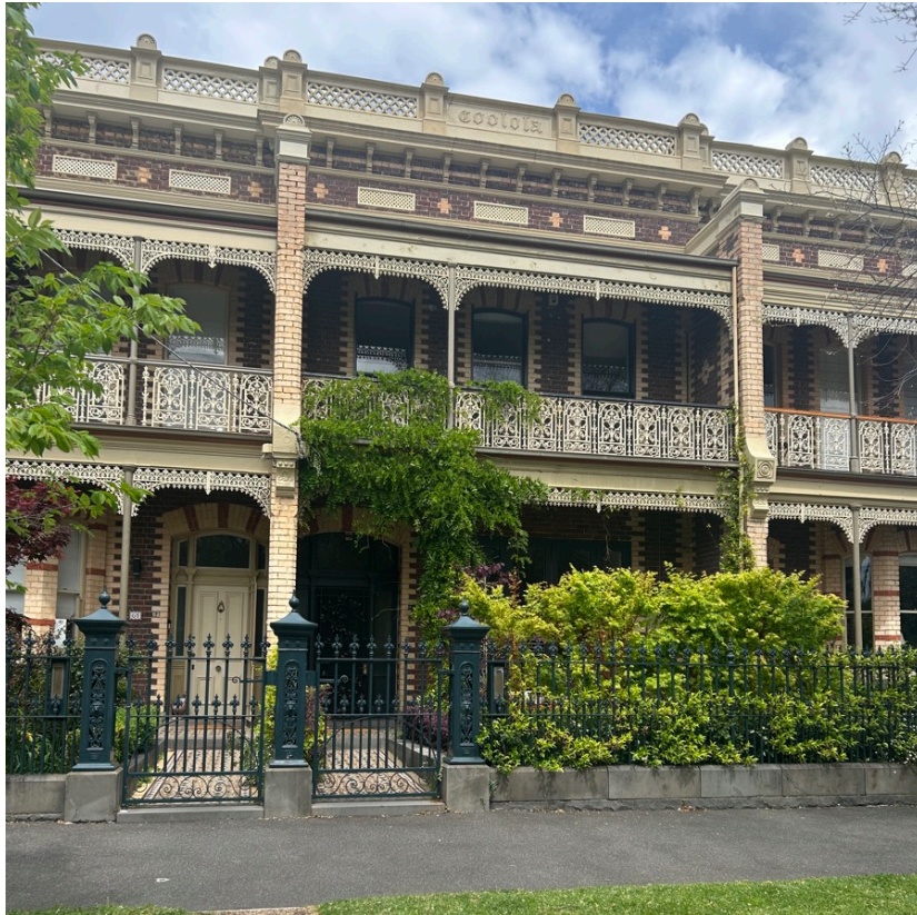
Figure 3 63 St Vincent Place South, the centre terrace, has lost the ground floor bay window. It is unfortunate that the original iron fence did not survive, the existing fence is a modern replacement.
