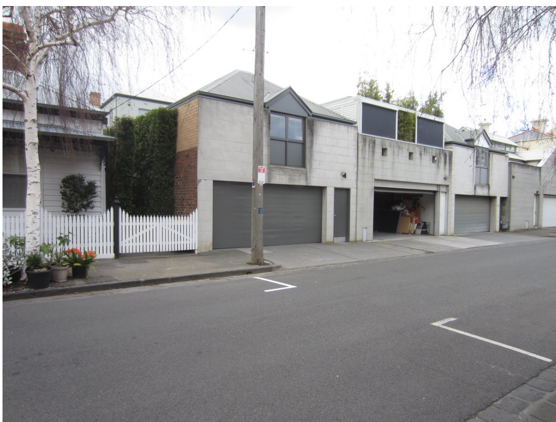
Figure 6 Rear of 61 to 65 St Vincent Place, Bevan Street.
