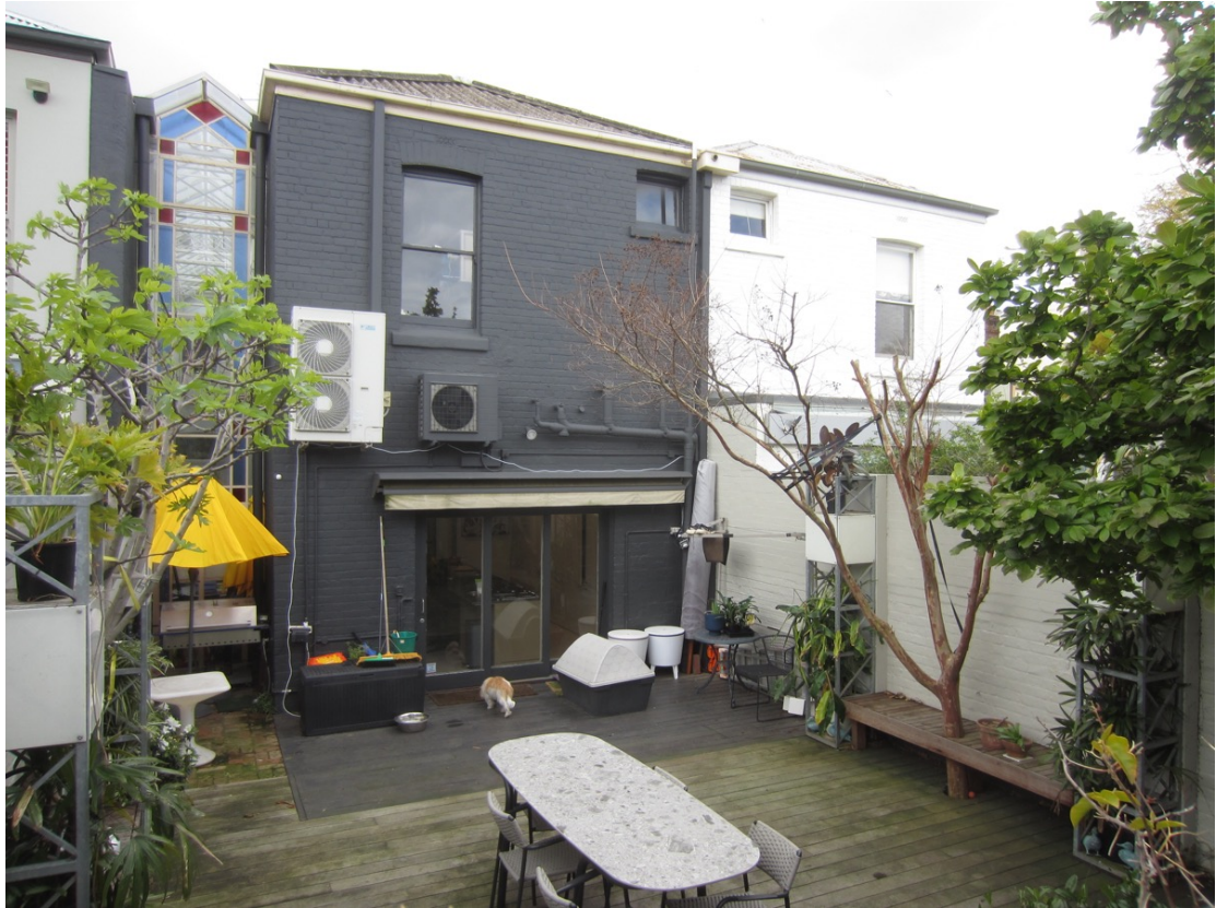
Figure 9 South elevation of 63 and 61 from terrace above 63 St Vincent Place garage.
