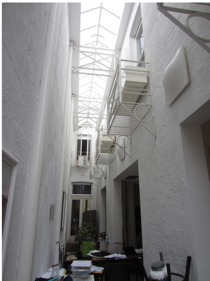
Figure 11 Interior view within the atrium looking north.
