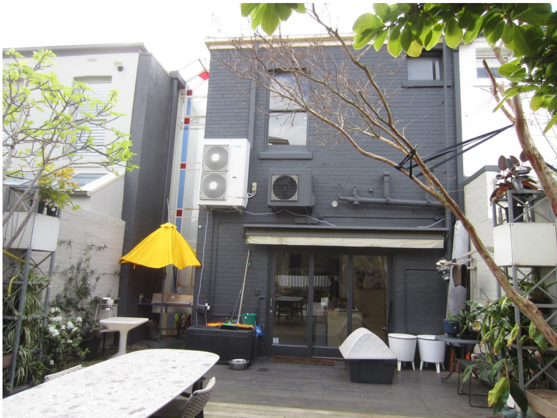
Figure 4 South wall of 63 St Vincent Place South.
