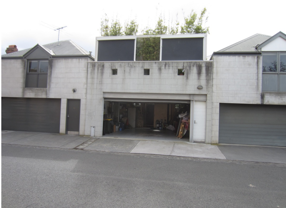
Figure 5 View of rear of 63 St Vincent Place South from Bevan Street.
