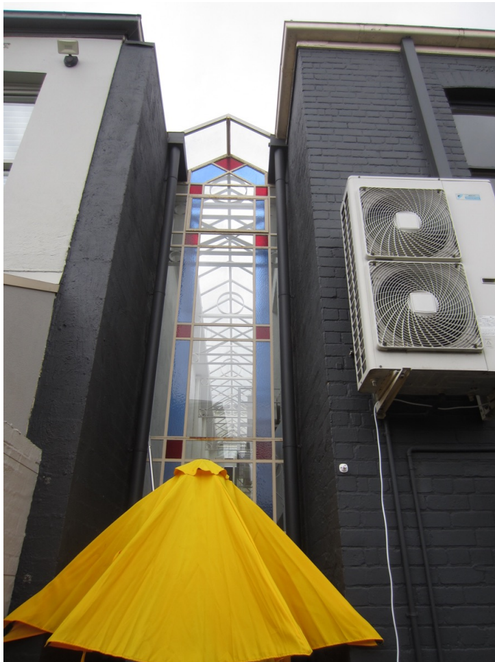
Figure 10 View from the south garden of the 1990s glazed atrium and west wall.
