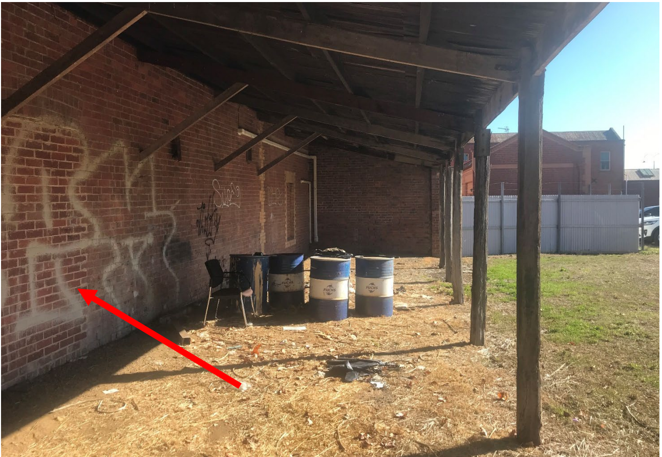
Figure 20 – The Oil Store Building verandah and ground beneath. Infilled opening indicated by red arrow.
