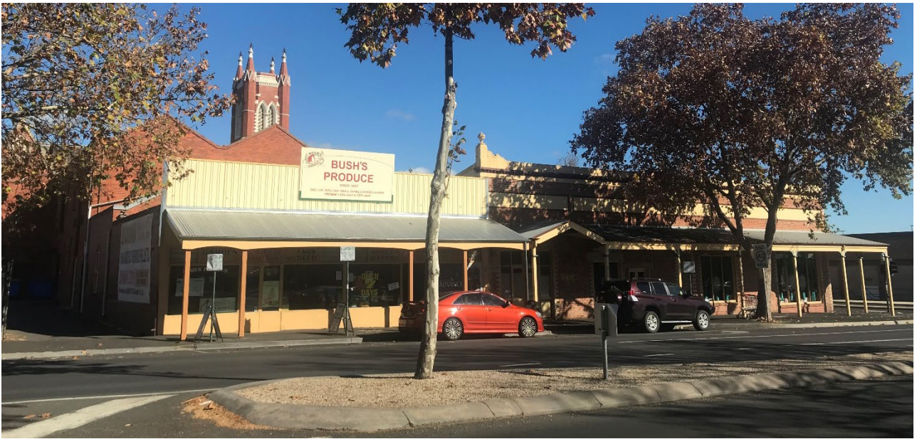
Figure 30 – The Bush's Store to the north of the subject site fronting Williamson Street.
