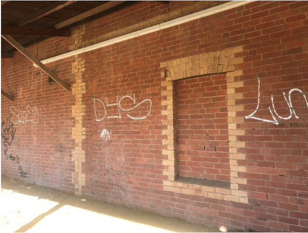
Figure 21 – Blind window to the northern end of the Oil Store Building.
