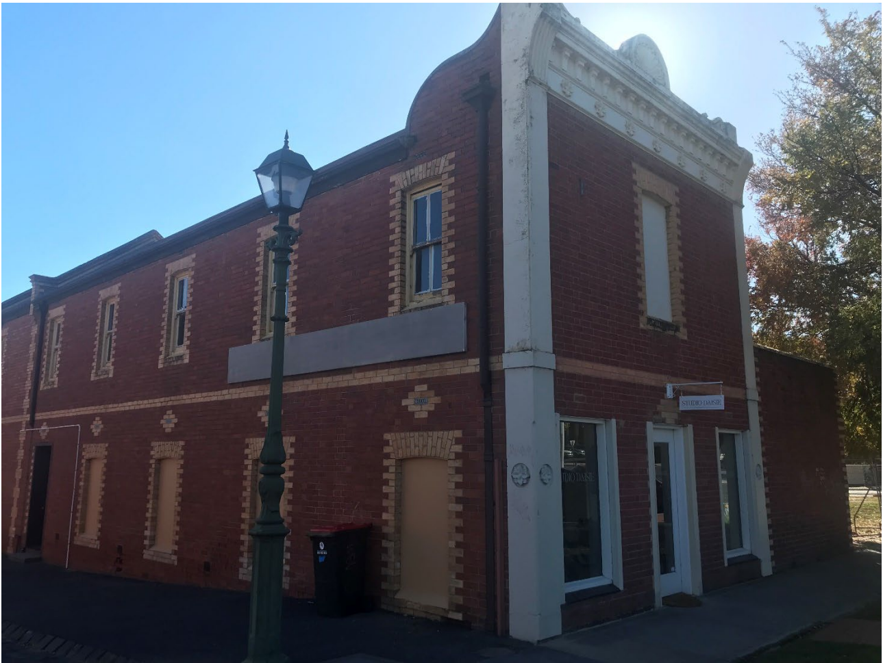
Figure 17 – The southern (Mollison Street) and western (Bushs Lane) elevations of the Oil Store building.
