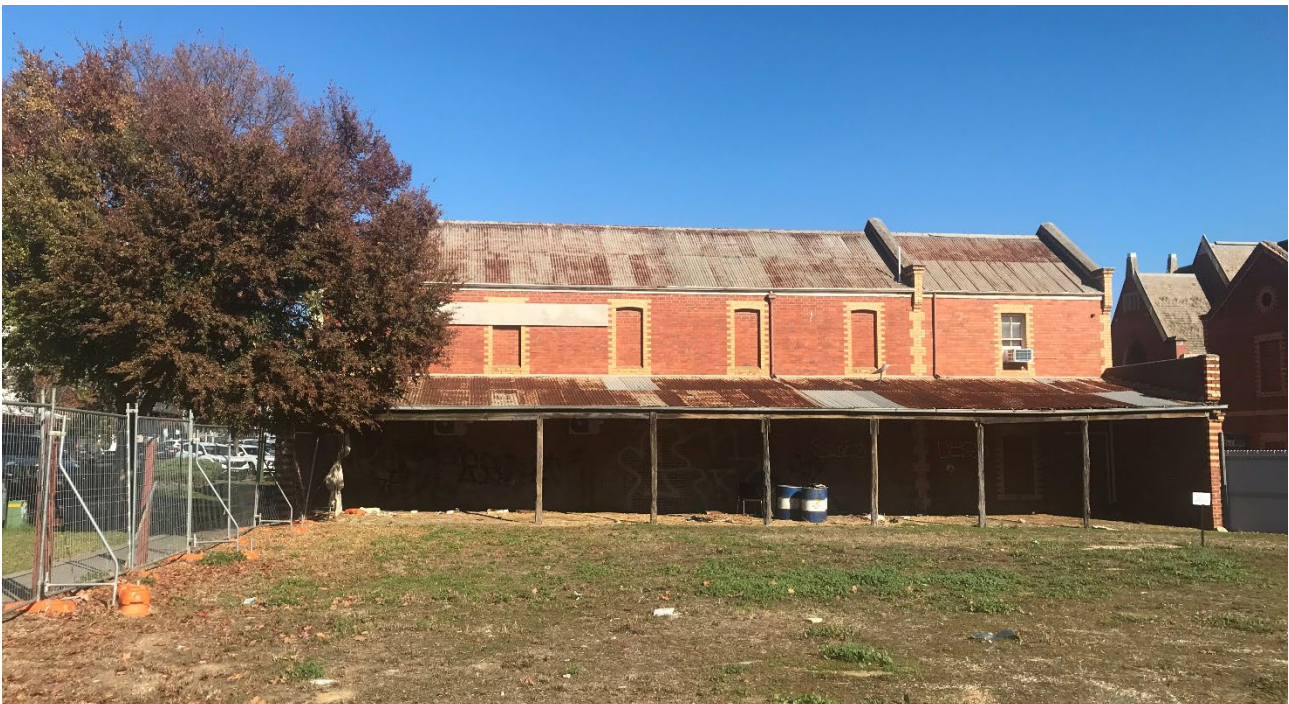
Figure 18 – The Oil Store Building and the verandah viewed from the east.
