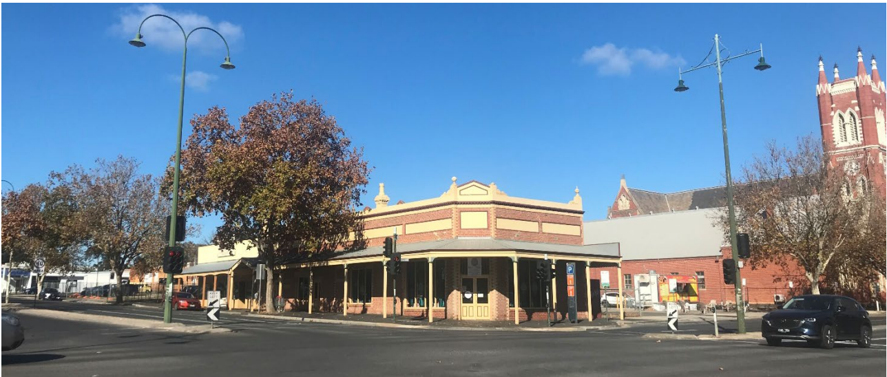
Figure 31 – The Bush's Store building fronting Williamson Street and Myers Street.
