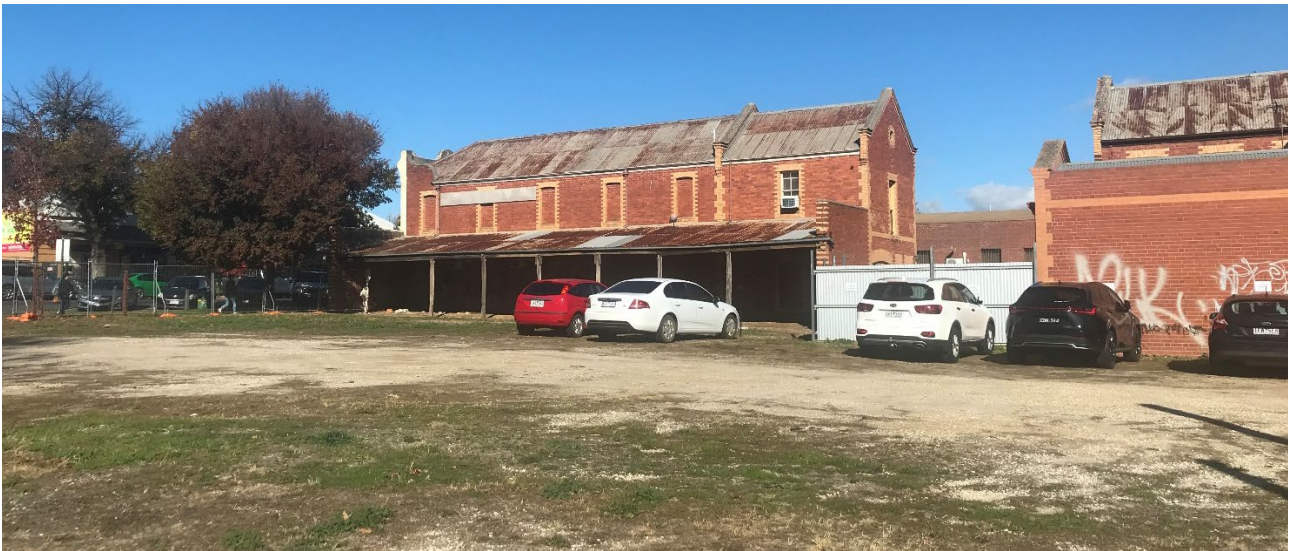
Figure 19 – The subject site looking southwest toward the northern end of the Oil Store Building.
