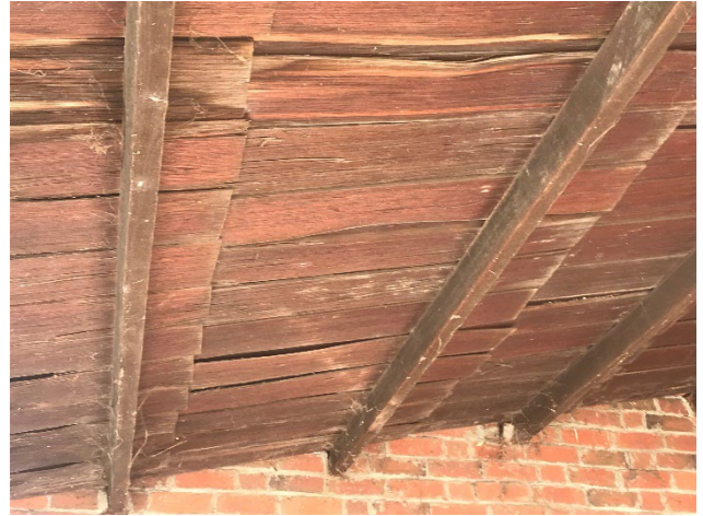
Figure 22 – Timber shingles beneath the corrugated sheet metal cladding of the verandah.
