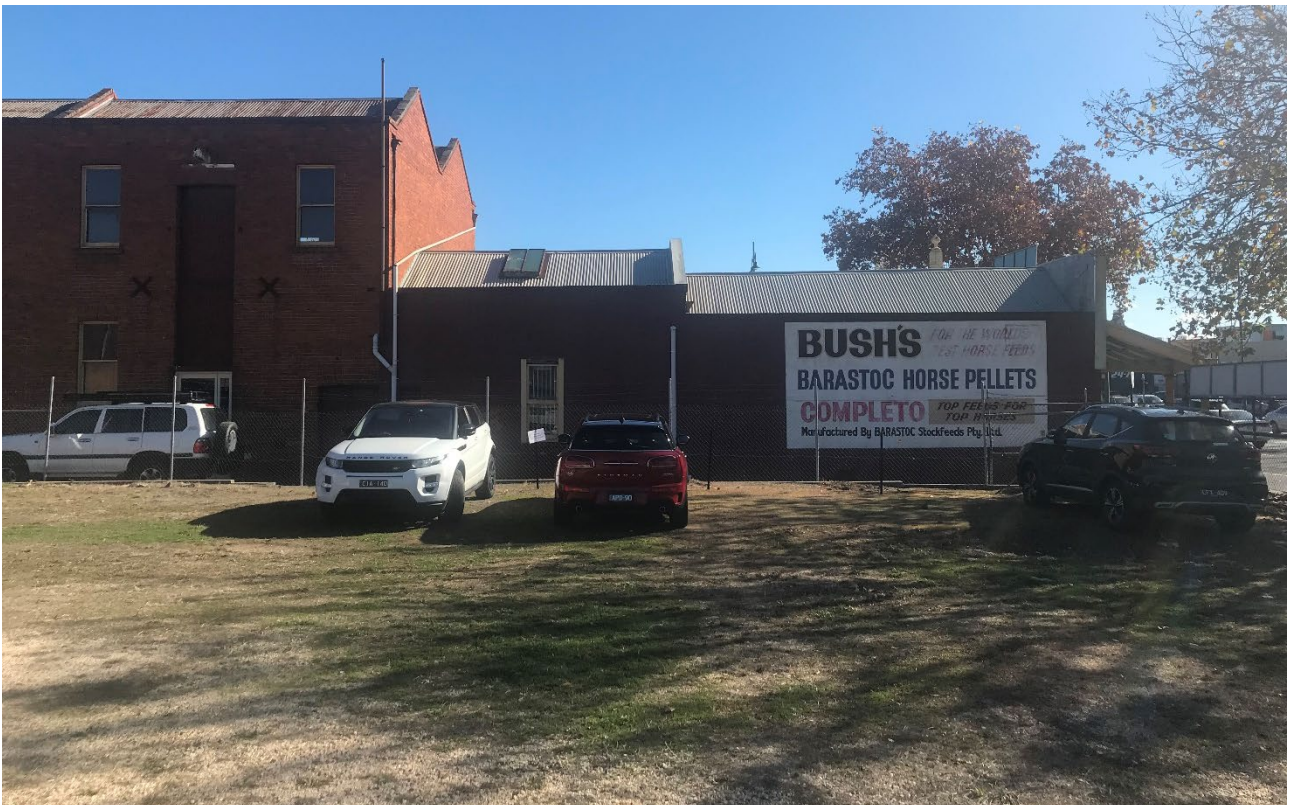
Figure 29 – The northern end of the subject site. A laneway divides the site from the southern wall of the Bush's Store.
