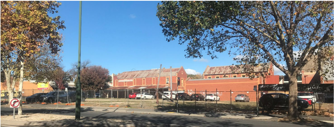
Figure 16 – The subject site, looking west from the opposite side of Williamson Street.
