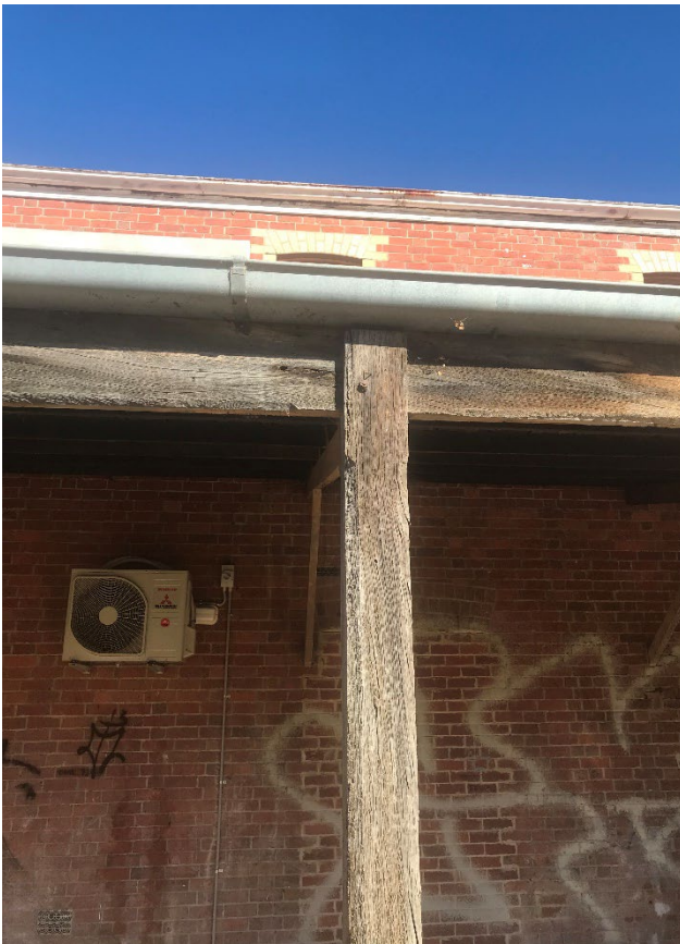
Figure 23 – Early timber posts and eaves. Non-original eaves gutter.
