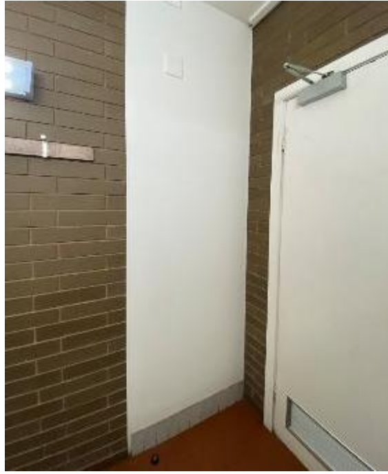
Figure 42: Female bathrooms, with plaster infill to previous alterations to change entry door locations. Source: Trethowan Architecture 2025.
