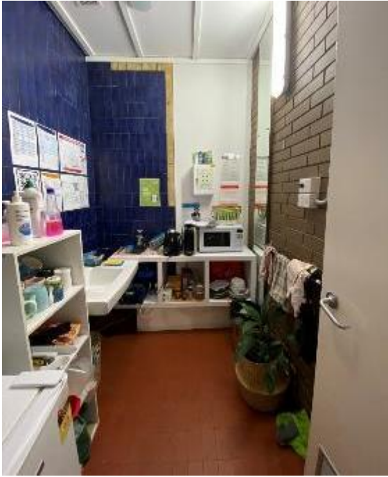
Figure 41: Staff kitchen area, noting basin fixture from its previous use as the Director office bathroom. Note missing tiles to back wall. Source: Trethowan Architecture 2025.
