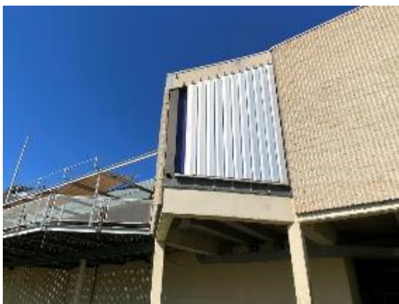
Figure 32: External aluminium louvres, presently in a 'closed' position. Source: Trethowan Architecture 2025.
