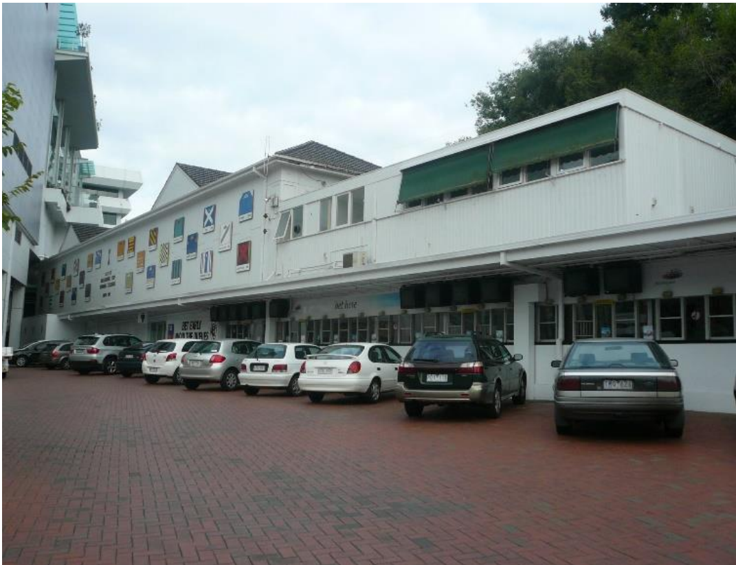
Figure 58 The former Colours building (left) and the adjacent totes (right) demolished in 2019
