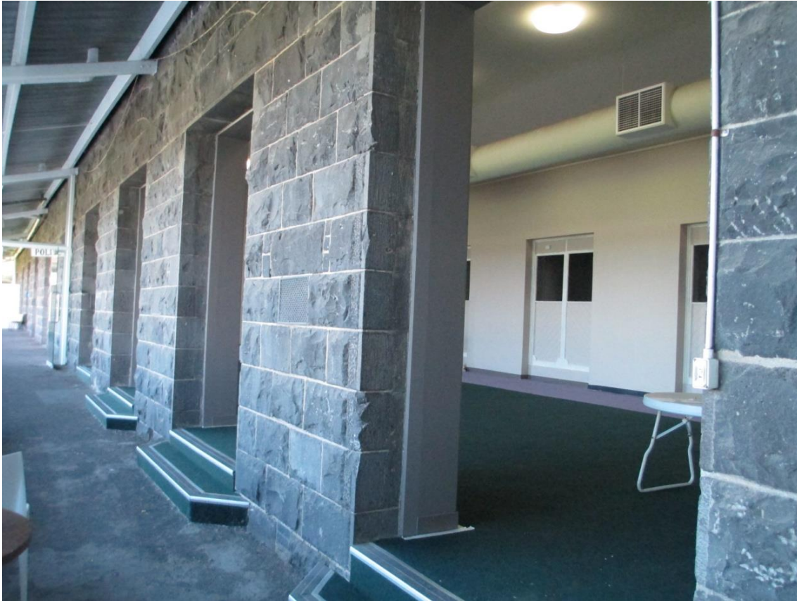
Figure 31 Level 1 of the bluestone stand with views into the interior spaces (2014 photograph)
