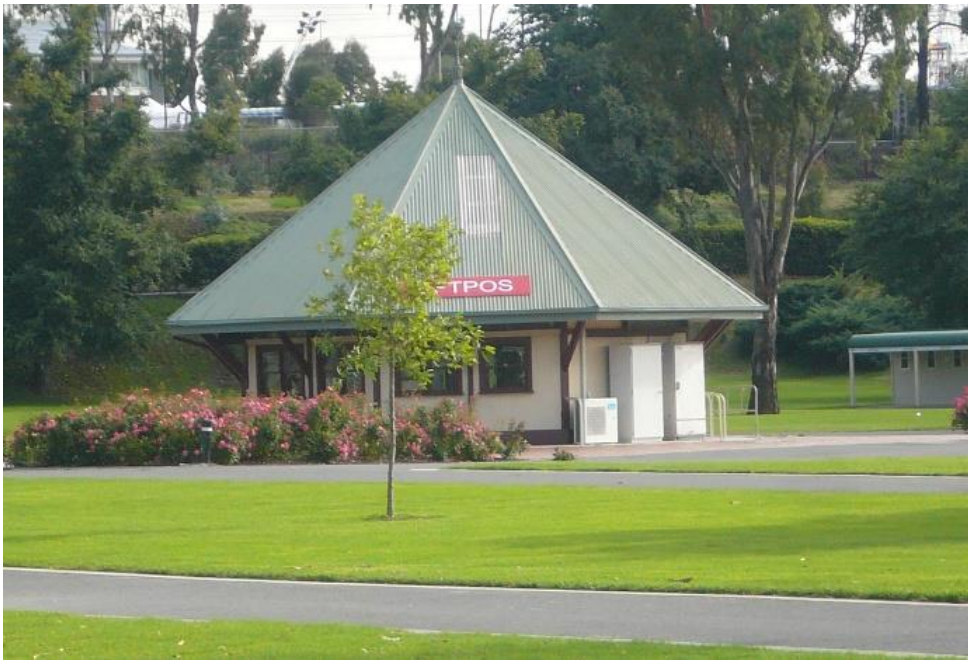
Figure 66 View of the Nursery Car Park Tote [2014 photograph]
