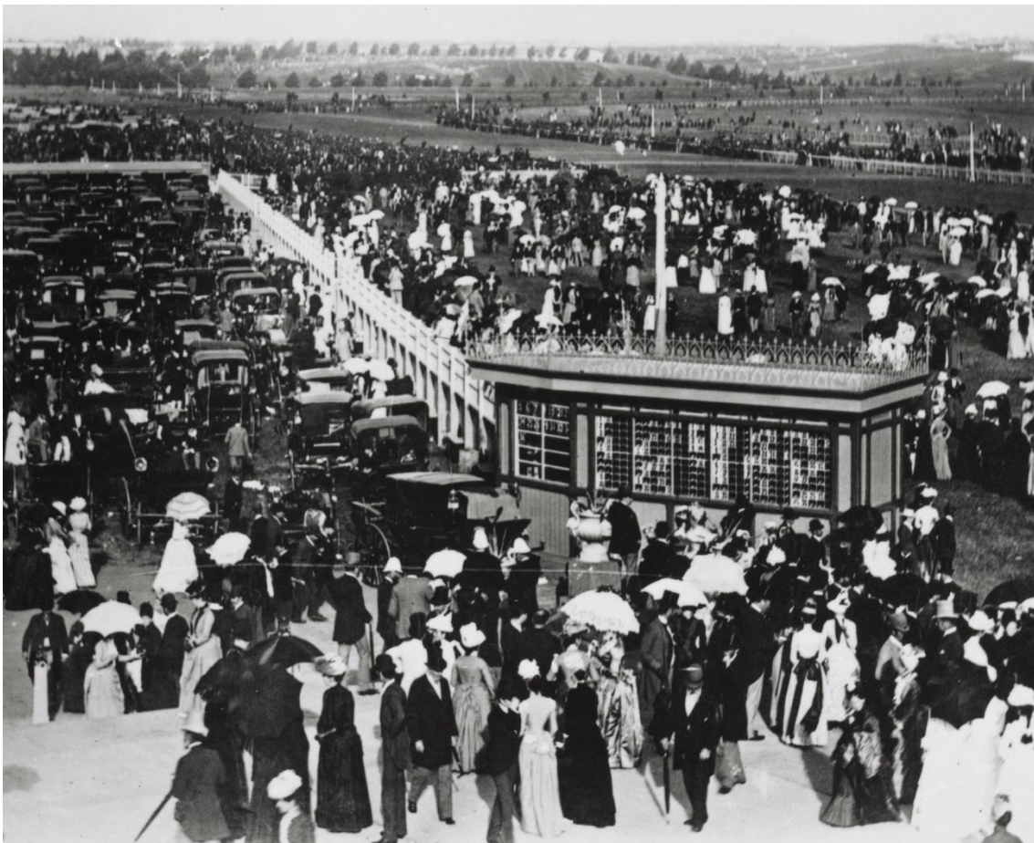
Figure 14 1895 photograph showing a semaphore or scratchings board at edge of the carriage paddock (near the current location of the Birdcage (car park) enclosures Source: Imperial Series, State Library of Victoria
