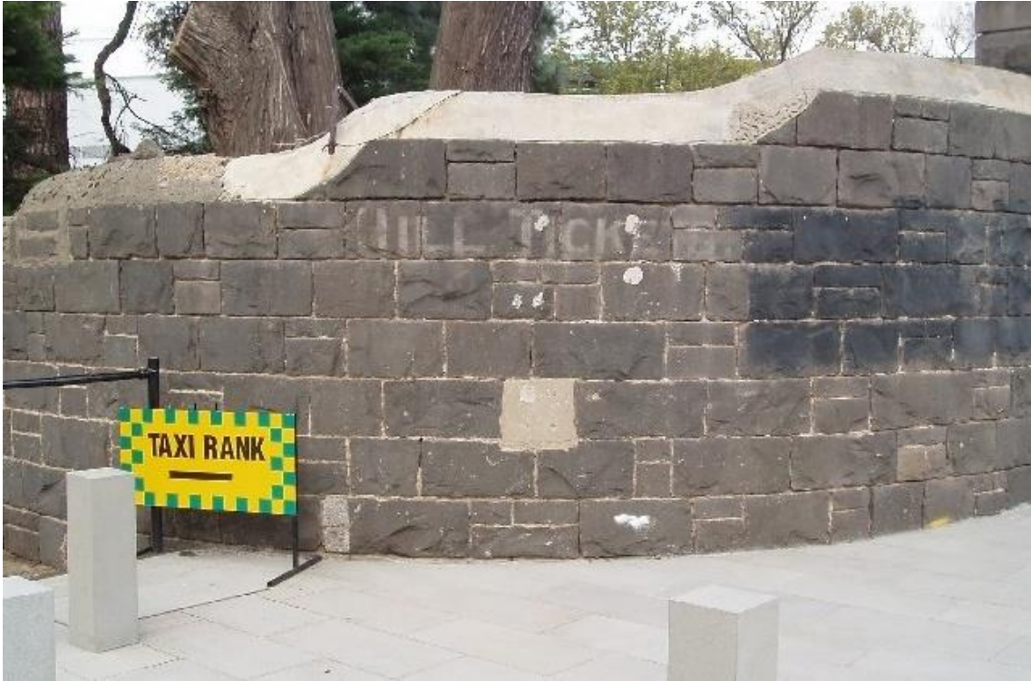
Figure 32 Bluestone wall at the Hill entrance showing the original 'Hill Ticket Box' painted signage (2014 photograph)
