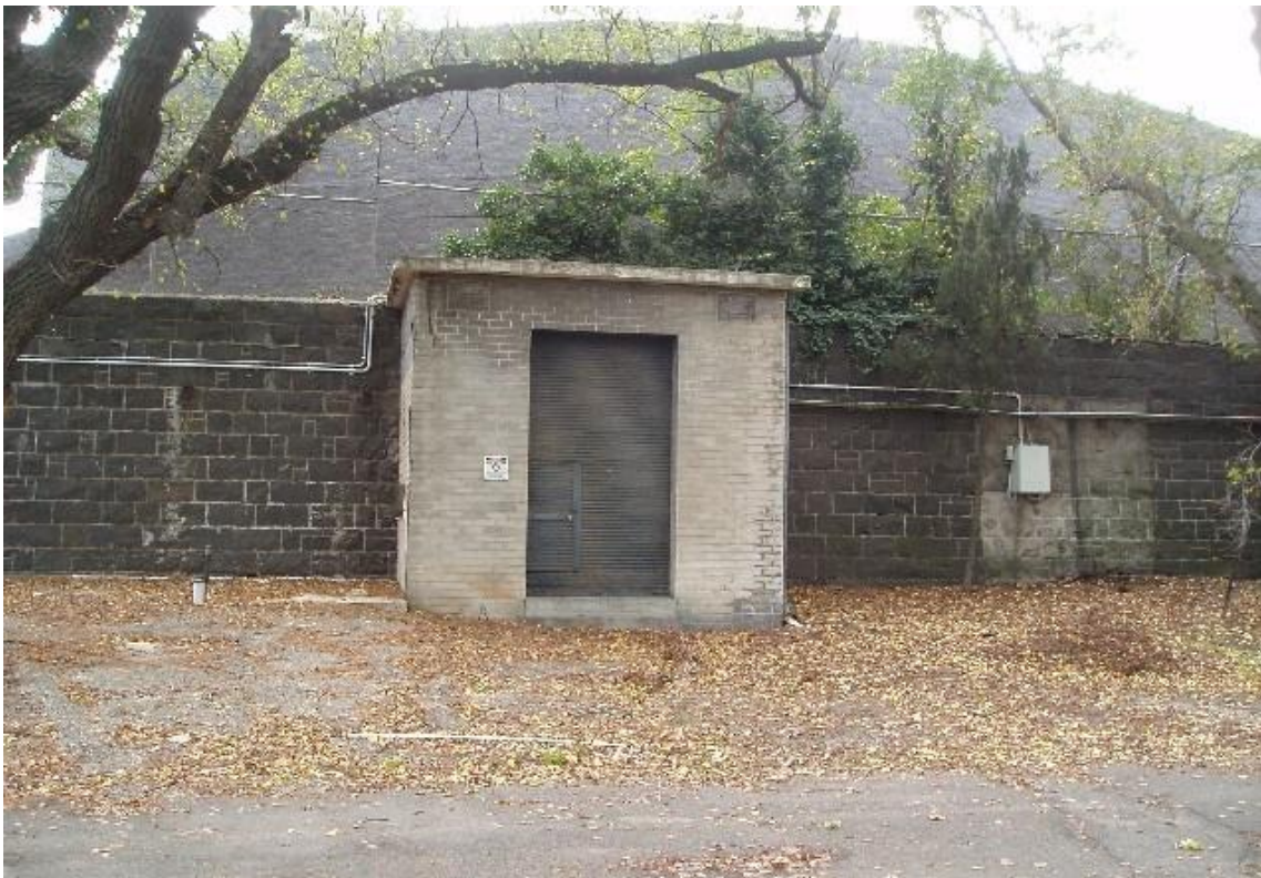
Figure 33 Bluestone wall with remnant horse tethering rings (2014 photograph)
