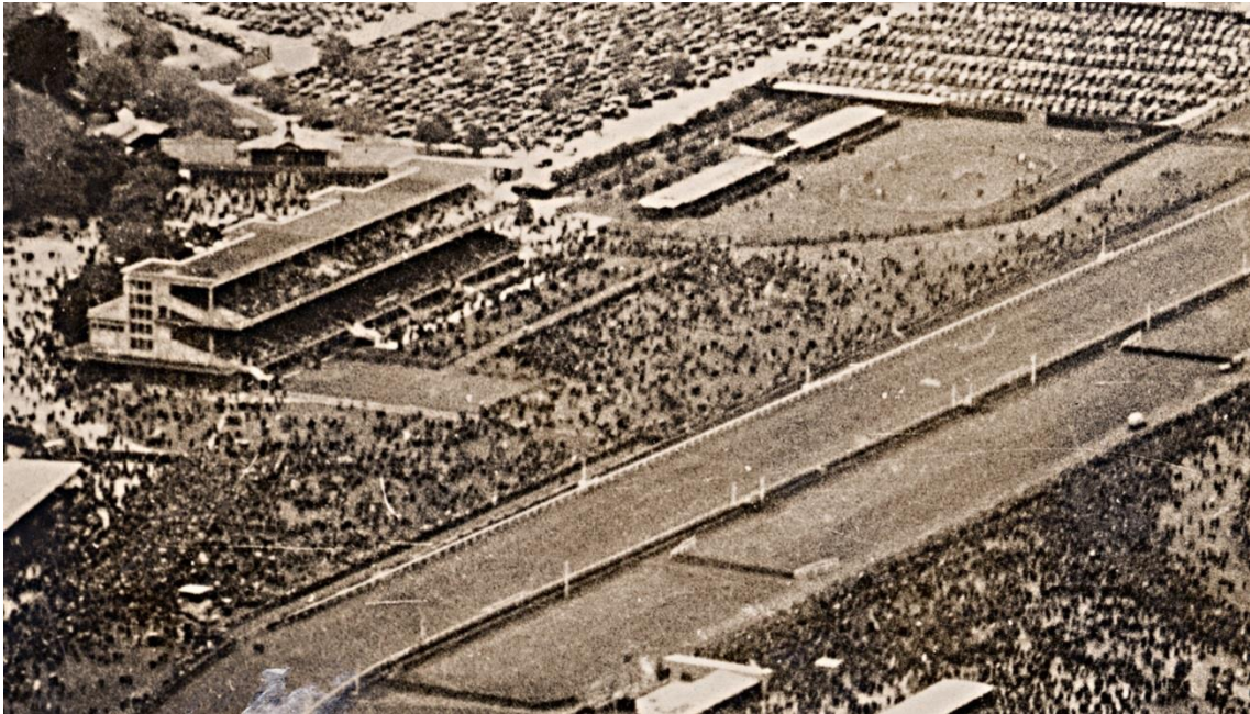
Figure 16 1932 aerial oblique photograph by Raymond Garrett showing the Race Day Stalls and Parade Ring, the connecting walk to the Mounting Yard located in front of the Members Grandstand (1924), and in the foreground the Horse Walk leading to a track entrance near the winning post, similar to its layout today Source: State Library of Victoria, photographer Raymond Garrett
