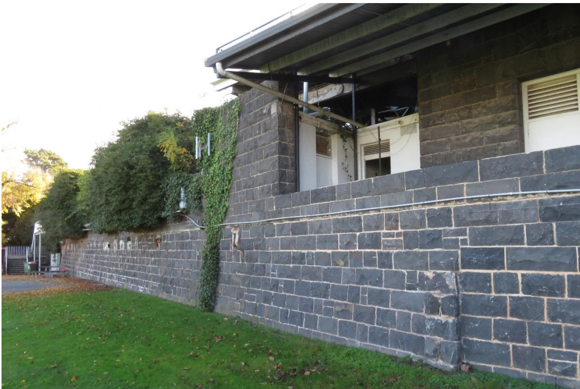
Figure 28 Remnant bluestone stand, showing the bluestone wall at ground level, bluestone building at level 1, and modern terraced seating above
