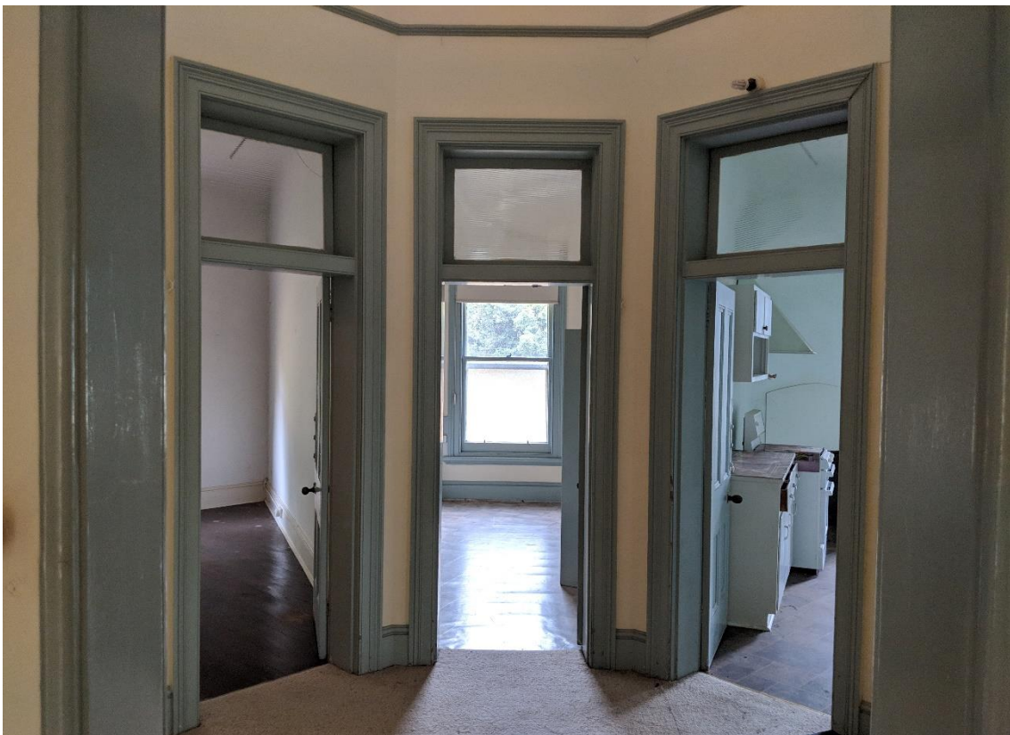
Figure 71 Octagonal hall and adjoining rooms of the former Jockeys' Convalescent Lodge
