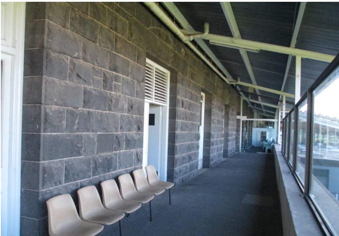
Figure 30 Level 1 of the bluestone stand showing entry to the rooms from the existing verandah (2014 photograph)
