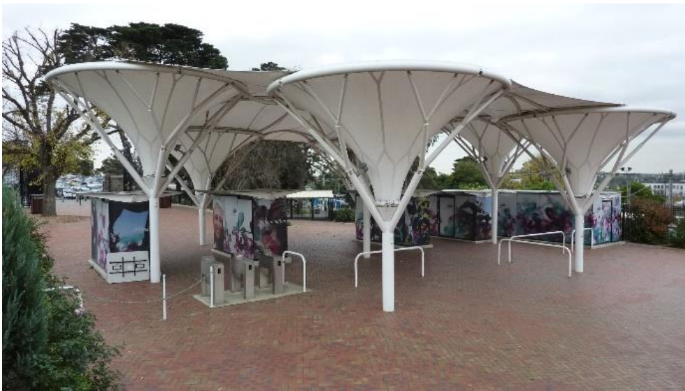
Figure 36 New Hill Gate pedestrian plaza and turnstiles
