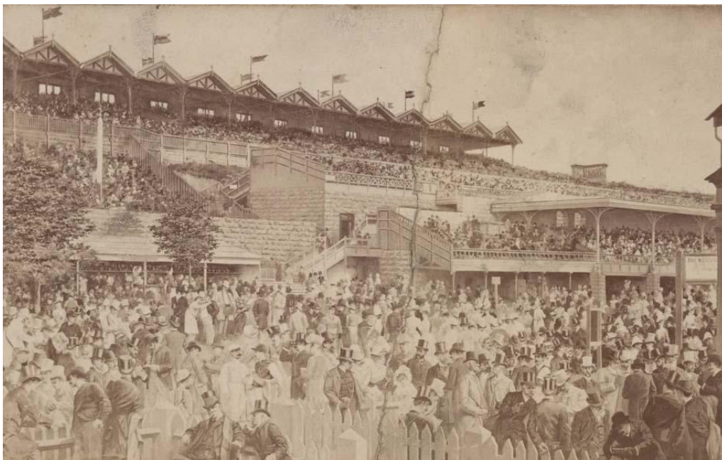
Figure 12 c.1890 image of Flemington Racecourse depicting the Hill Stand (top) and 'Bagot's Cowshed' (bottom). This image also shows the upper level stand behind the 1873 stand, as added in the 1880s.
