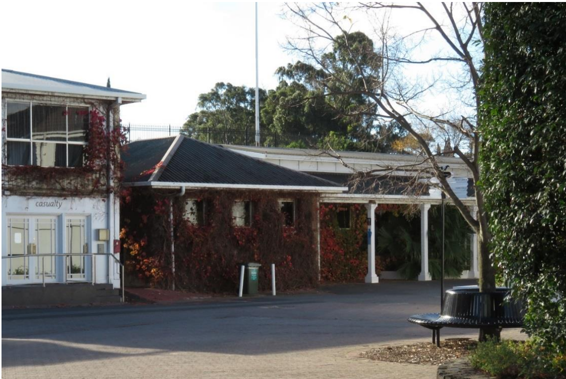
Figure 62 Toilet block along the northern perimeter of the Betting Ring
