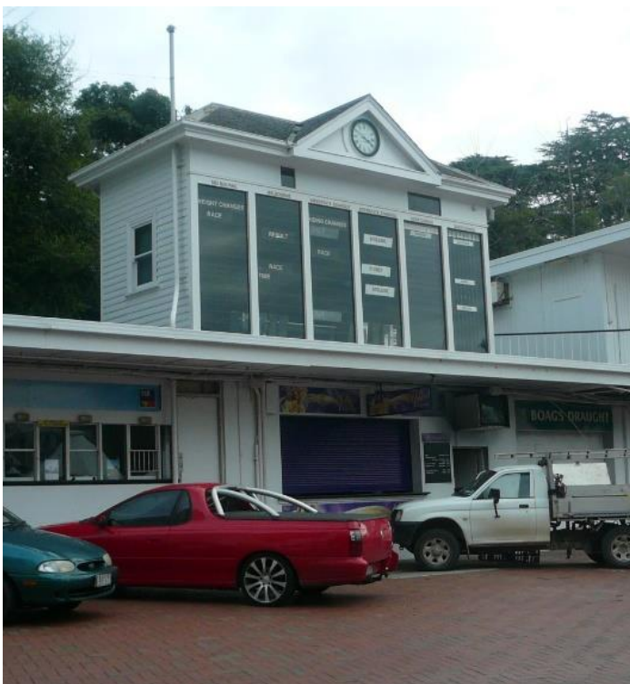
Figure 59 The 1926 'Semaphore' (Scratchings Frame) building, retained in the 2019 works (this view pre-dates the works)
