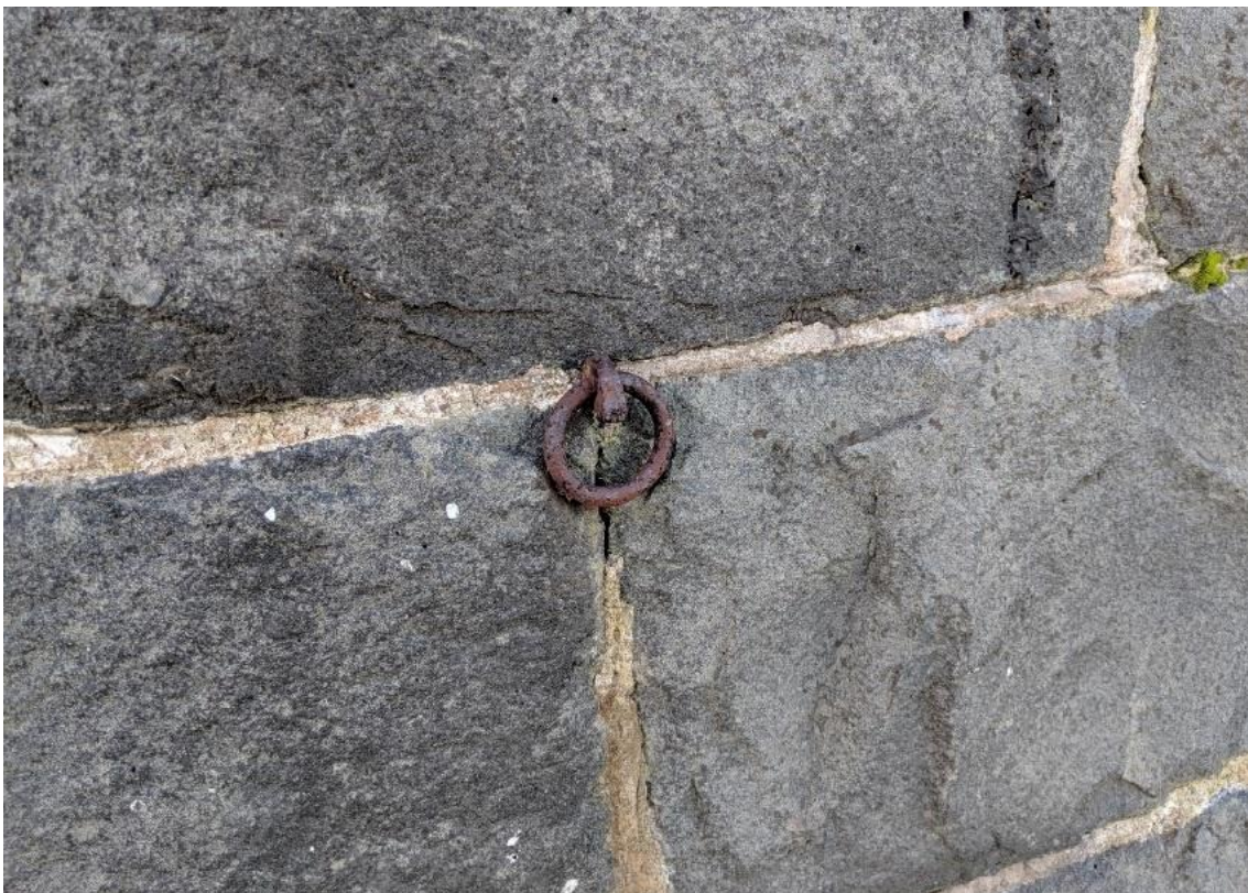
Figure 35 Detail of remnant horse tethering ring in the bluestone wall
