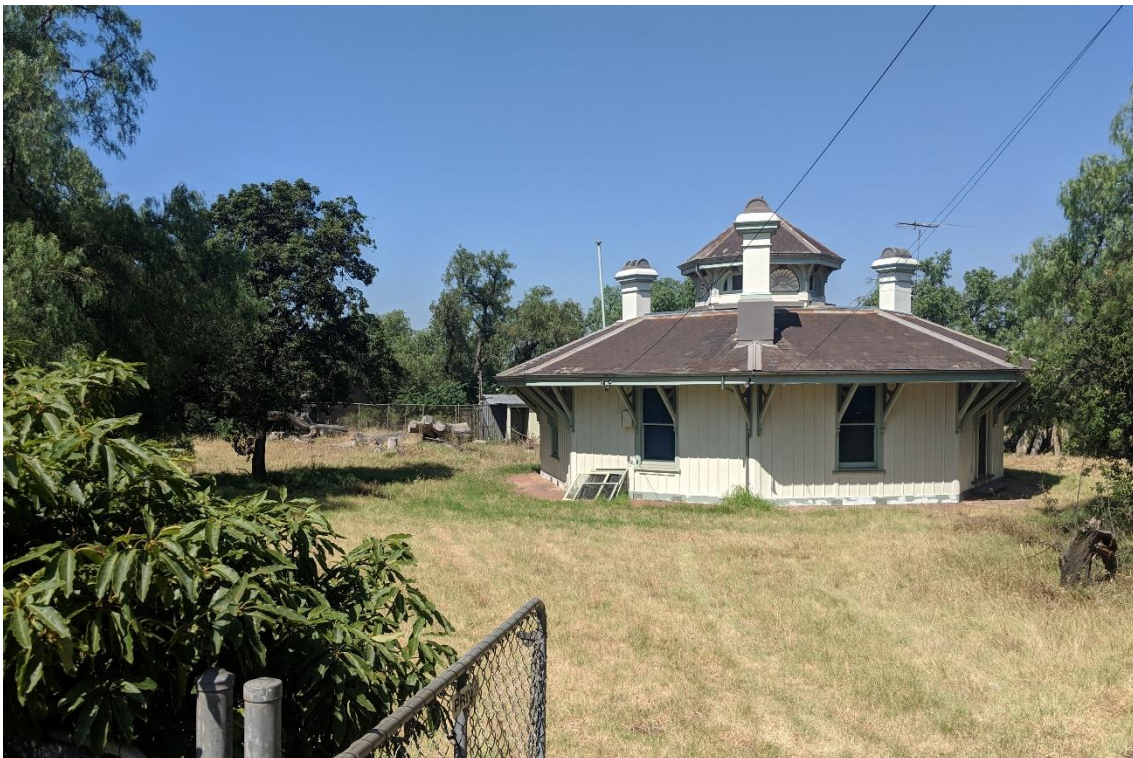
Figure 69 The Jockeys' Convalescent Lodge viewed from the access drive
