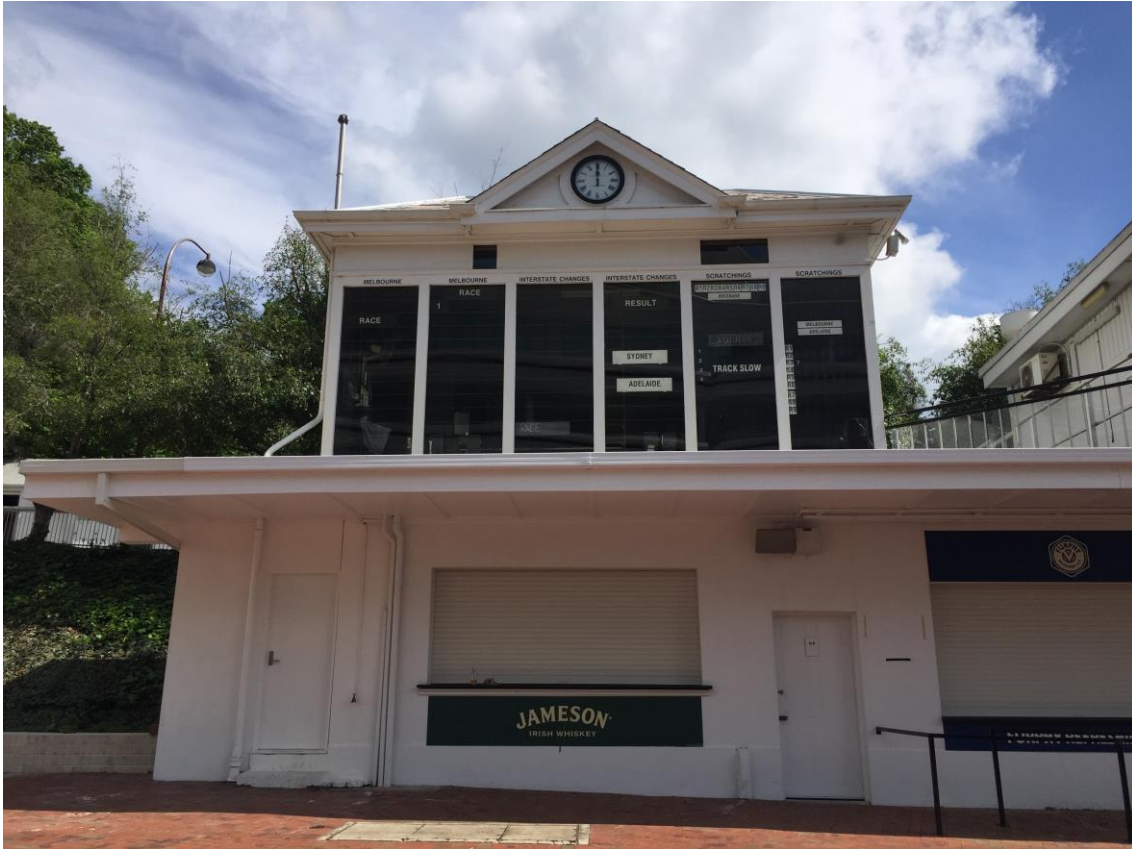
Figure 60 Retained section of the 1926 'Semaphore' (Scratchings Frame) building
