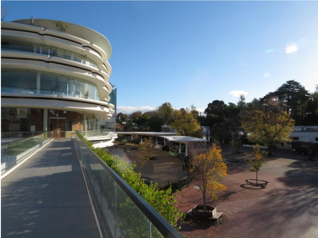
Figure 55 Overview of the Betting Ring looking north west from the elevated platform between the Parade Ring and the Club Stand
