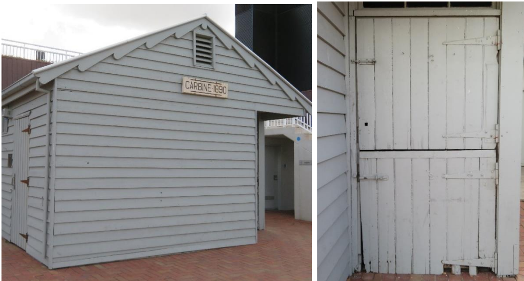
Figure 77 Left: Carbine's Stall viewed from the south. Right: Detail of stall door, with tripartite lights above
