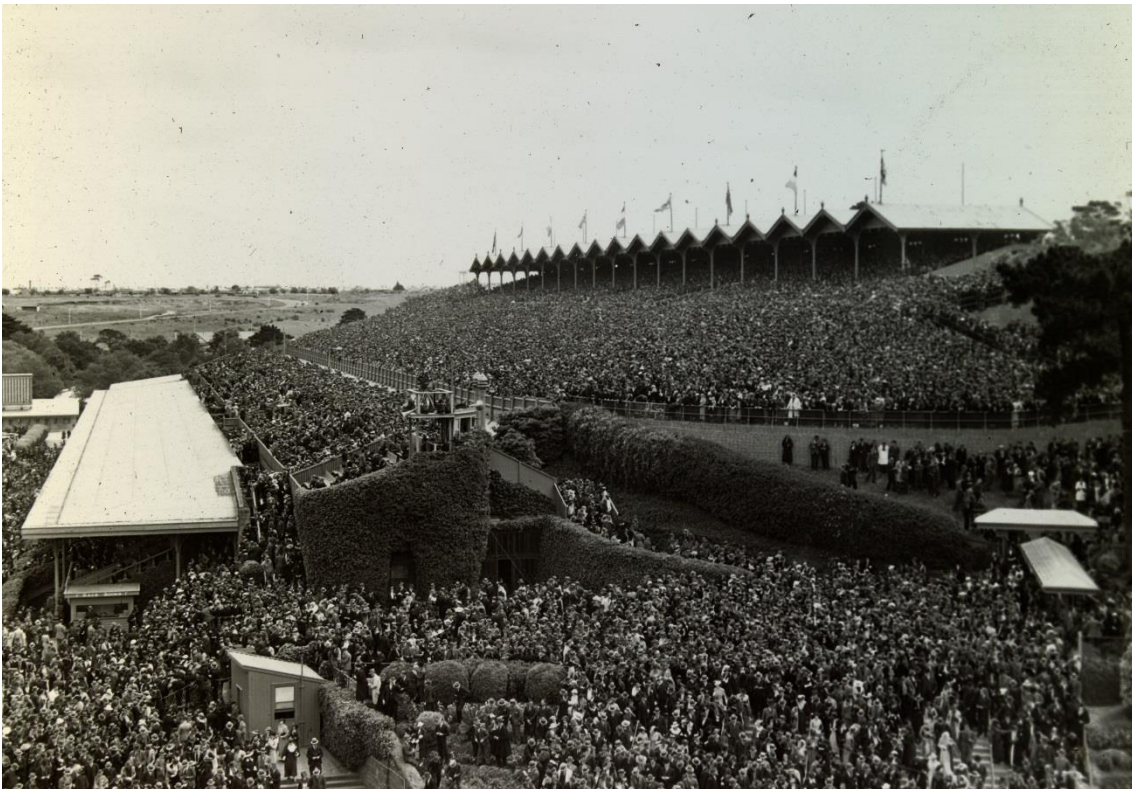
Figure 7 c.1900-1920 view of the Hill at Flemington during the Melbourne Cup, showing the various stairs, terraces and buttresses created to improve the topographic feature as a viewing stand. Much of these works were later removed in the construction of modern grandstands
