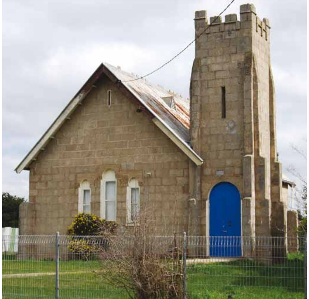
Figure 9: The Snake Valley Wesleyan Church constructed in 1908 is of architectural and scientific (technical) significance as the first known example of a building constructed in Victoria using concrete blocks to form a hollow cavity wall. The blocks are made with a mix which includes quartz pebble aggregate sourced from the nearby mullock heaps created by gold mining activities. Source: Heritage Victoria, 2008.
