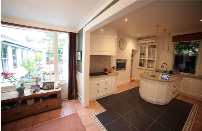
Figure 11: Existing kitchen/dining area looking south-east out to corridor proposed for demolition (The Heritage Conservancy, 2024)
