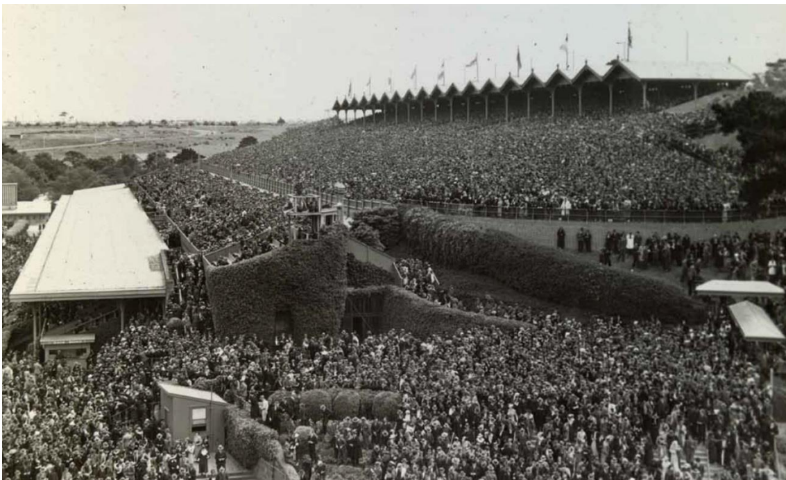
Figure 14 Stands at Flemington in the early 1920s. From left, Bagot's Cowshed, the Upper Grand Stand, the Hill Terrace and the Hill Reserve Stand Source: Public Record Office Victoria
