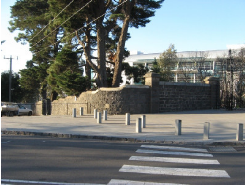
Flemington Racecourse_bluestone walls near Hill Entrance_KJ_15 Jun 09
