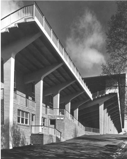
Figure 25 Rear view of the 1955-7 Hill Reserve Grandstand and terrace Source: State Library of Victoria Pictures Collection
