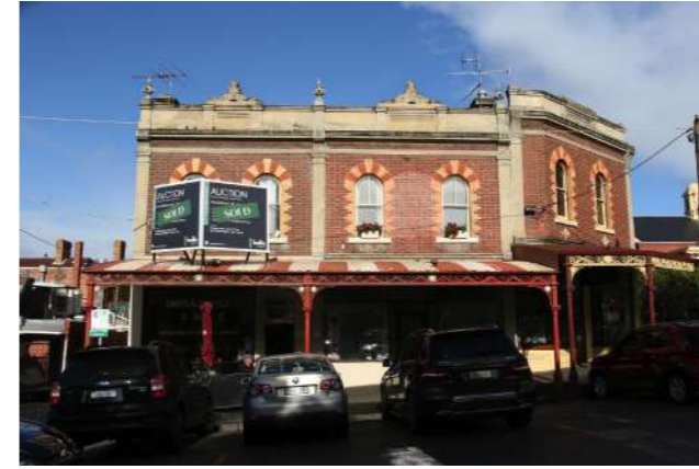
7. NORTHERN VIEW OF 189 BANK STREET
