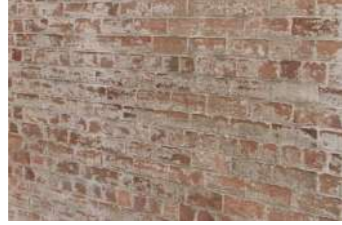
MAS01 EXISTING RED BRICKS
