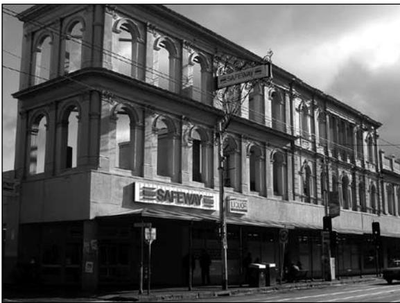
*Facadism resulting from inadequate fabric retention*
