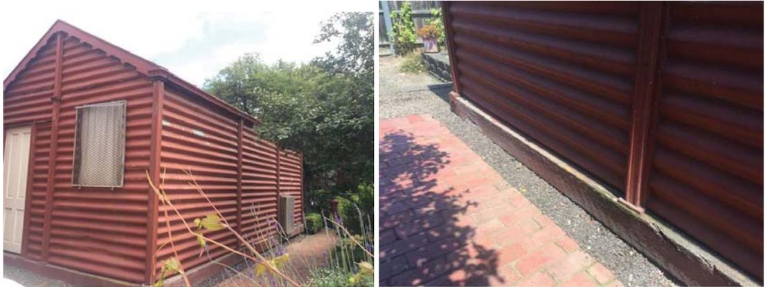
The existing timber base beam of the building, which is deteriorated and requires replacement
