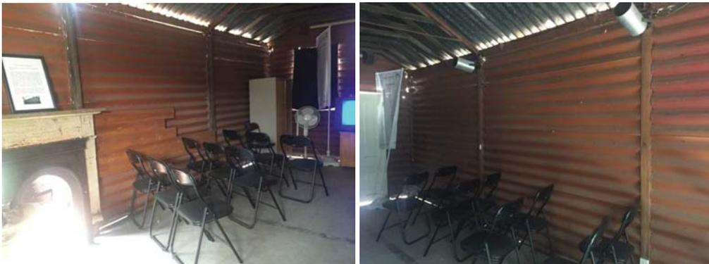
**The current interior of Bellhouse House showing the internal timber posts inserted into the structural cast iron posts – these will be used as the fixing points for the perimeter and cross lateral bracing.**
