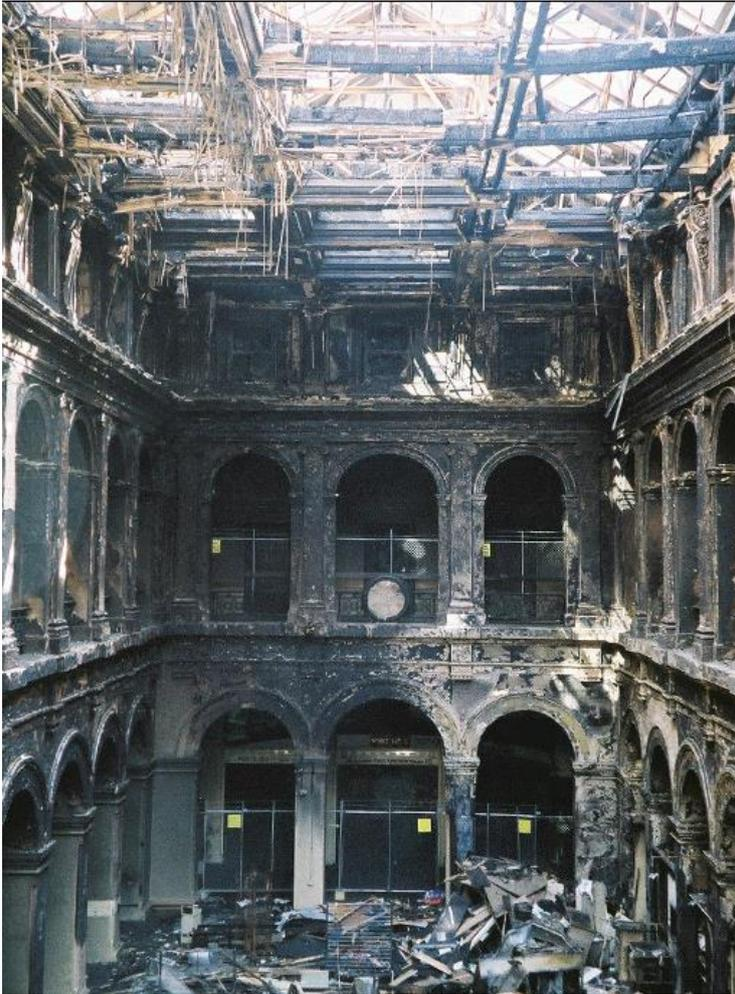
Figure 1      Extent of damage to the Melbourne GPO postal hall, following 2001 fire
