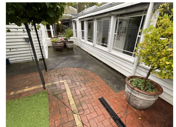
Existing Back Wall
