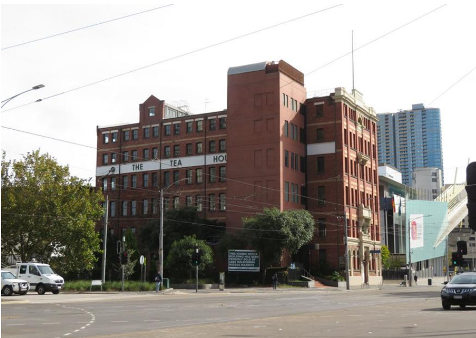
Figure 7 South-east elevation of the Robur Tea Building
