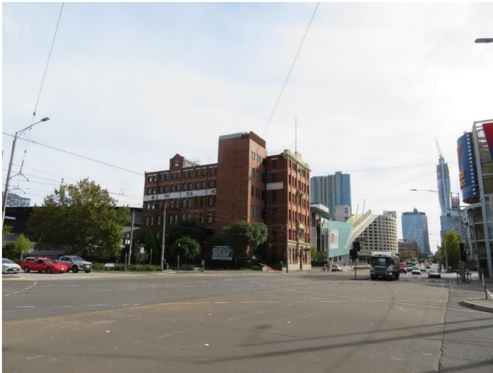
Figure 28 View from the south-east, with the services core prominent
