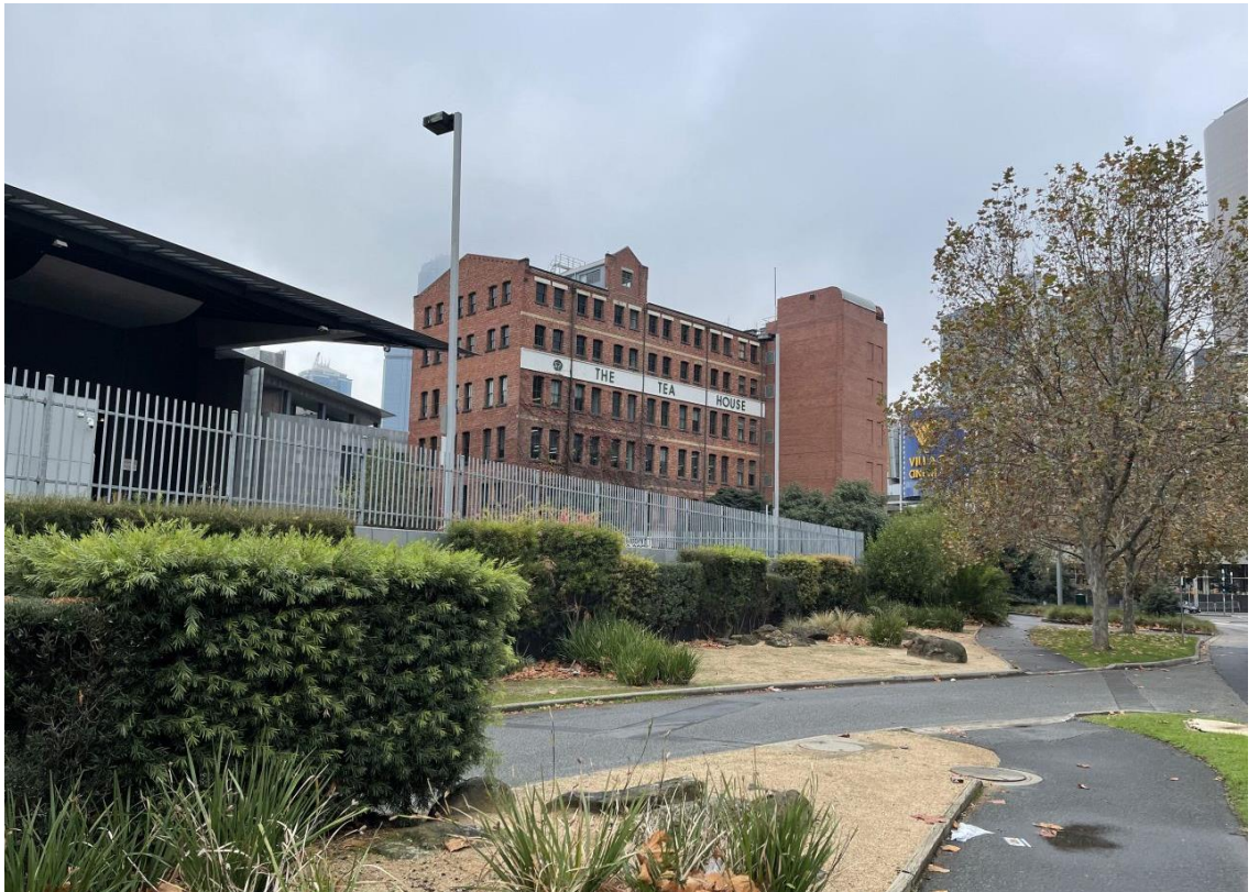
Figure 9 South and west elevations of the Robur Tea Building
