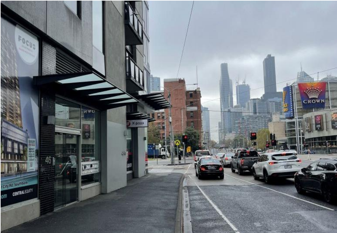
Figure 17 Building seen from the west side of Clarendon Street, south of Normanby Road
