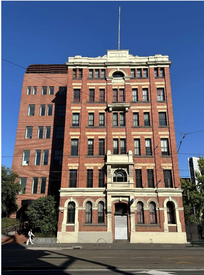
Figure 5 Principal (east) elevation of the Robur Tea Building to Clarendon Street
