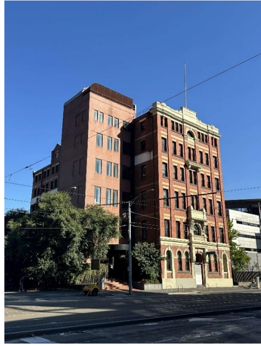
Figure 15 East elevation of building
