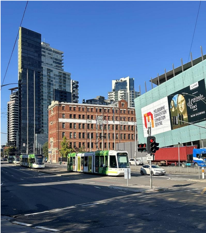
Figure 26 View of the Tea House from opposite the convention centre, note the contrast in materials and design
