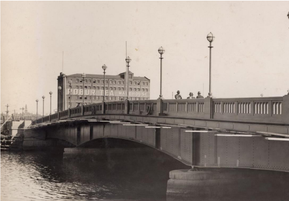
Figure 21 View looking south to the Tea House across the newly constructed Spencer Street bridge, c. 1929 Source: State Library of Victoria
