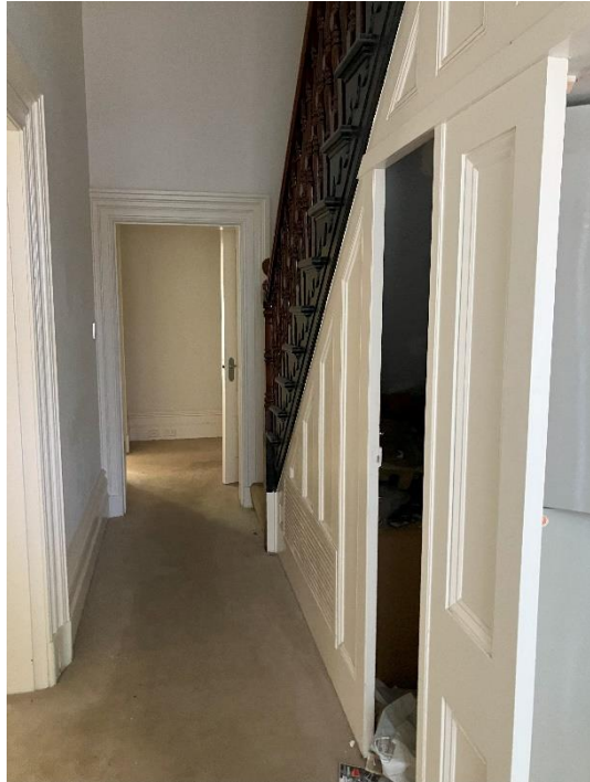
Basement entrance under the rear (servants) staircase
